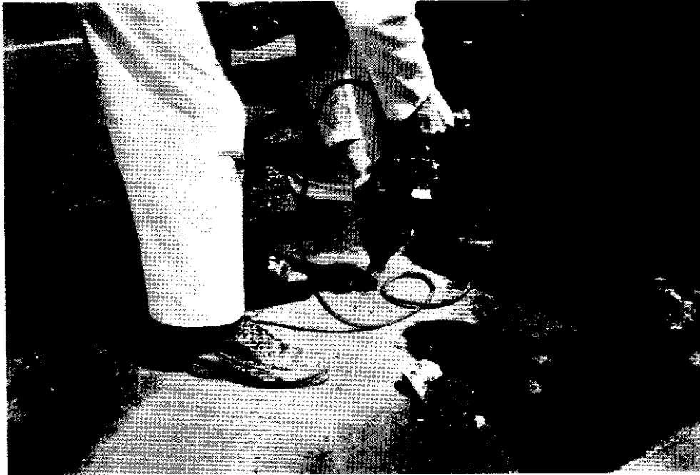
Figure 22. Digging Concrete in Core Location to Reach Rebar for Ground (Columbia River Bridge Deck)
