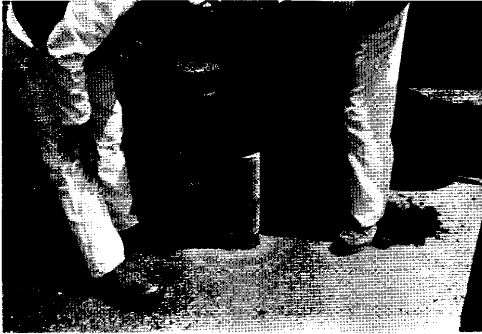
Figure 18. Core Sampling AC Overlay and Membrane by Truck-Mounted, Nitrogen-Cooled Coring Rig (Columbia River Bridge Deck)
