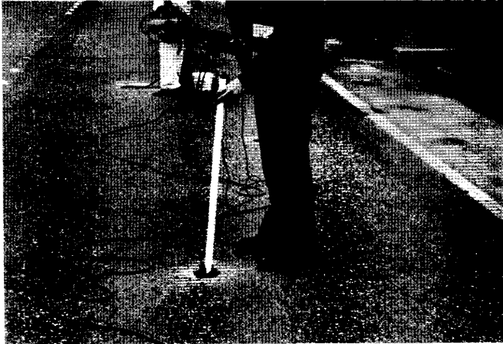
Figure 20. Half-Cell Measurement on Exposed Concrete in a Core Location (Ebey Slough Bridge Deck)
