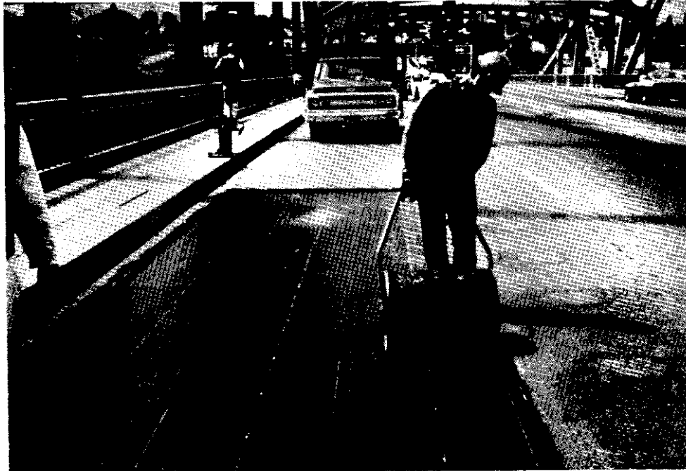
Figure 28. Using a Hand Roller to Bring Membrane Completely in Contact with Concrete Surface (Columbia River Bridge Deck)
