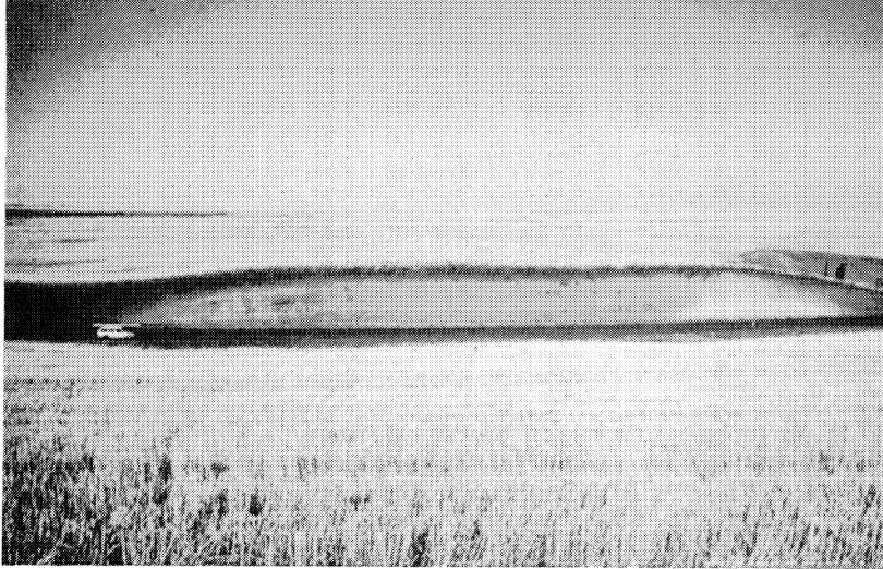
Figure 29. The natural surface drainage is away from the slope face. Little erosion damage has occurred.
