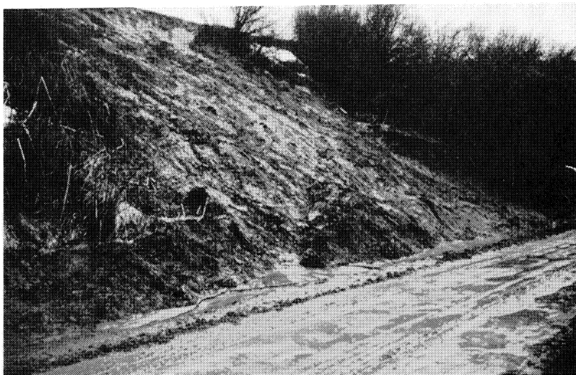
Figure 35. Relatively large scale mudflow located near Pullman. Undisturbed soil to the right of the photograph indicates the depth of failure at approximately 3 feet.
