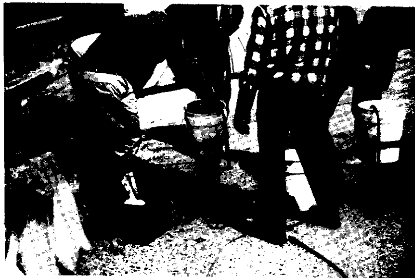
Mixing component A and B, gray pigment, and powdered carbon in 5 gallon pails.
