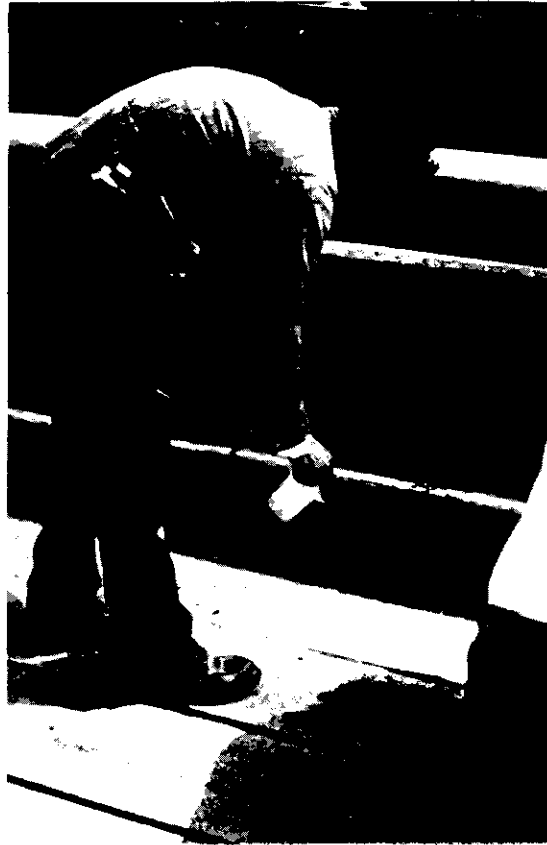
Sprinkling silica sand by hand on the conductive polymer for skid resistance.
