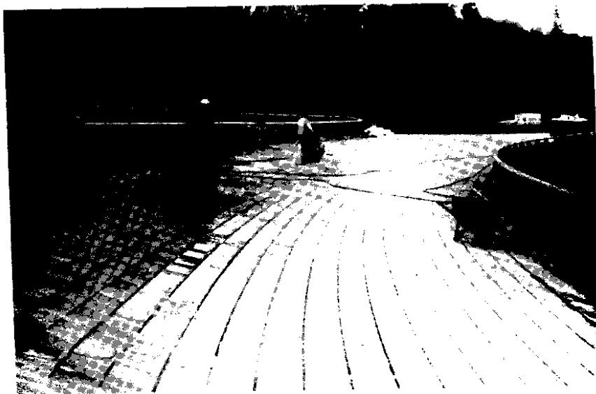
Slots at one foot center running longitudinal on the deck.
