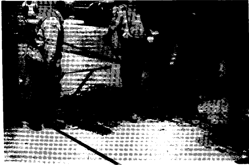
Distribution of slurry mixture in front of screed. Note screed bars on deck and handle for pulling screed.
