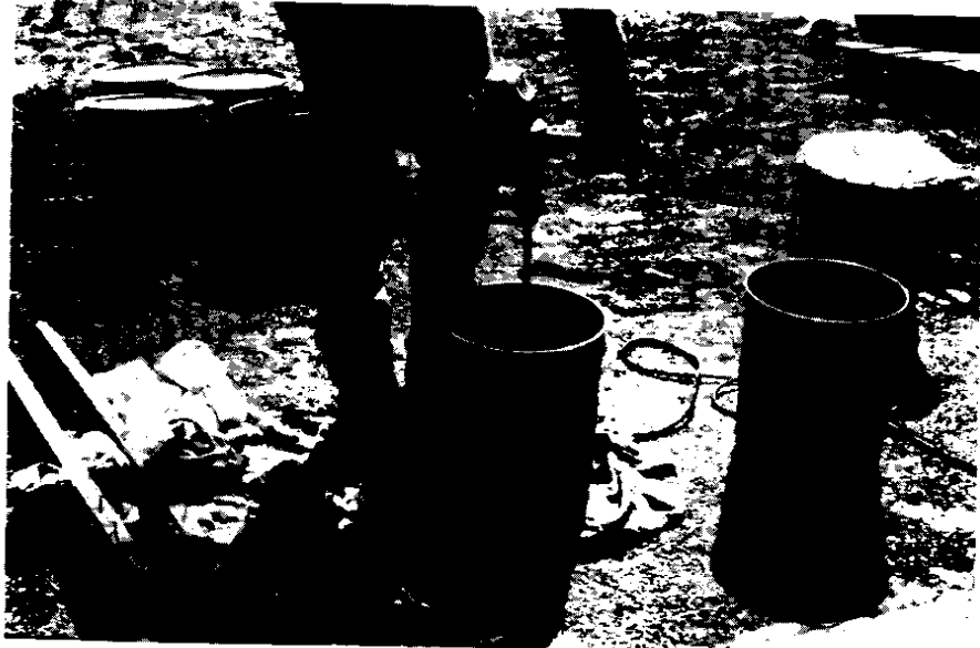
Hand mixing of epoxy binder for broom and seed method.
