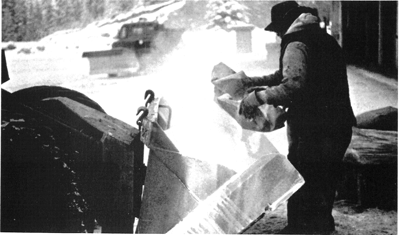
Figure (5) Bagged CMA being emptied into loader bucket
