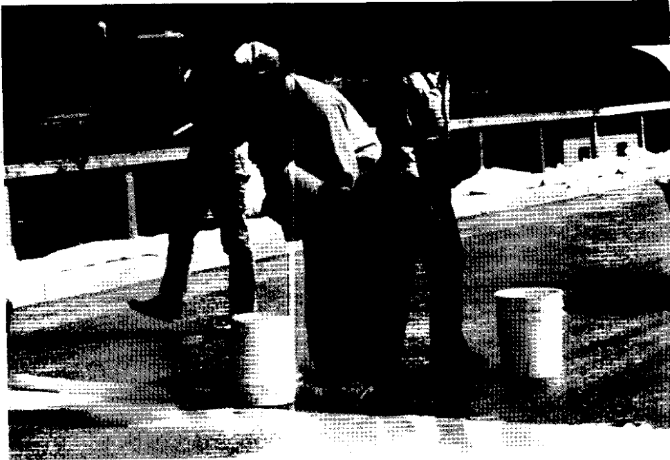
Spreading Aggregate by Hand
