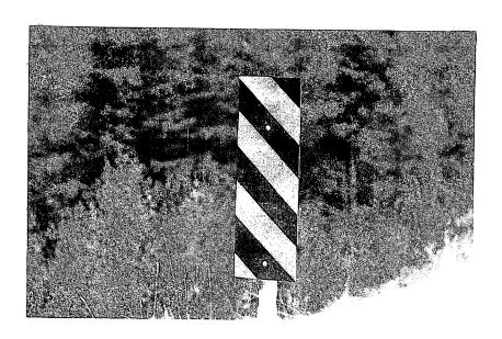
Plate 2-4 Hazard Panel on Barrier Top
