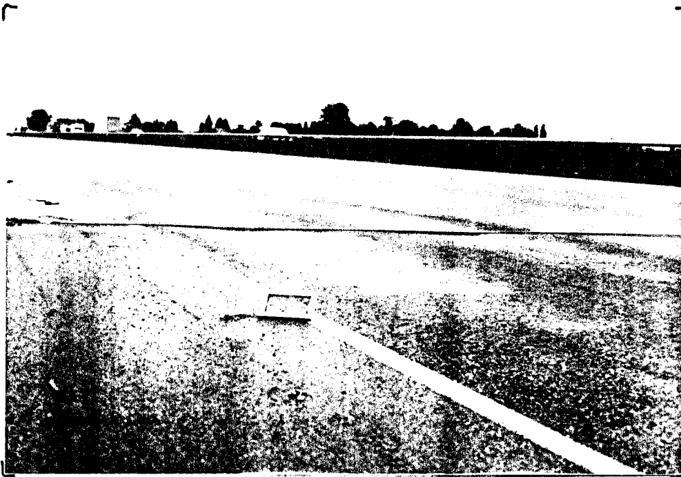
5/645 E - Surface shows some raveling, rutting and flushing in various areas. Heavy high speed traffic. Paved 1982. Rated 9
