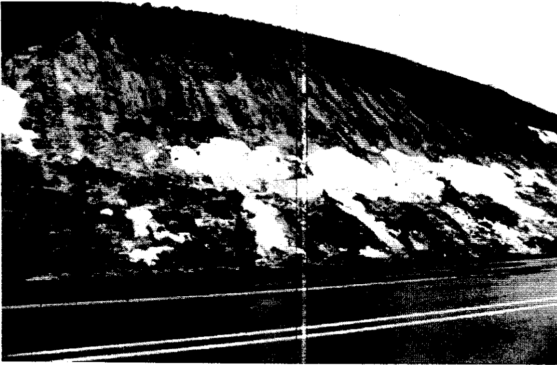
Figure 15 Failure of Cut Slope in Clayey Loess
