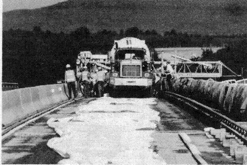
Visqueen placed to protect deck
