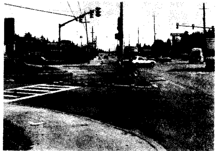
Photo 5.6 Free right turn lanes speed up traffic, and increase the discomfort and apparent danger to pedestrians. They should be eliminated and replaced with small radius corners.
