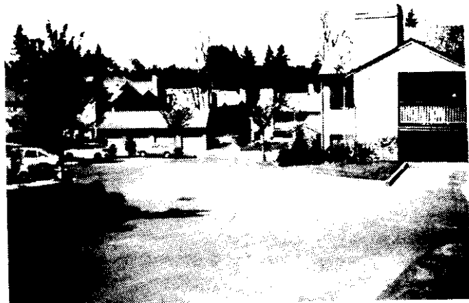
Photo of existing entry condition. The existing landscape is auto dominated, consisting of wide parking lots with few walkways.
