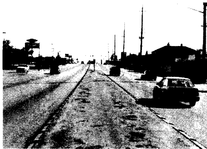
Photo 4.3. Existing median in Lynnwood prevents left turns for about 1/2 mile, even though there are driveways on both sides of the street. Planting the median would visually scale down the highway.
