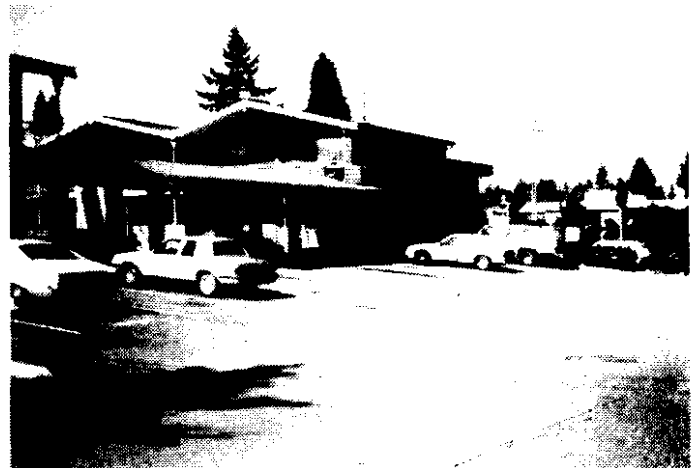
Existing conditions. The apartment is set back from the road by a 'head in' parking lot, making travel by foot difficult and unsafe for many. No sidewalk, curbs or planters exist.
