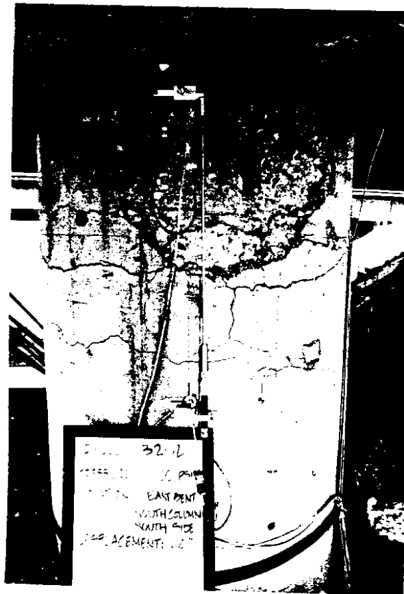
Figure 7.13. Photograph of Damage at 2.0 Percent Drift
