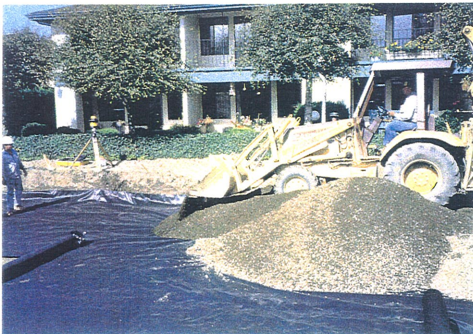
Figure 5.98 - Spreading out the initial lift during the recent project.
