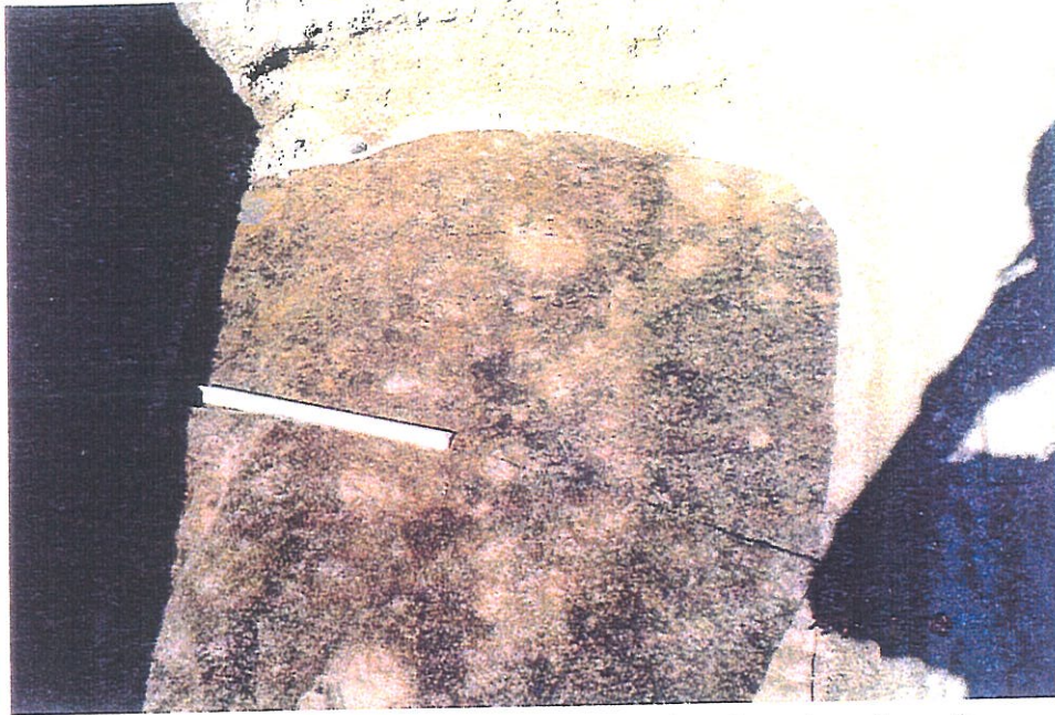
Figure 5.84 - Geotextile folded back exposing the subgrade surface.
