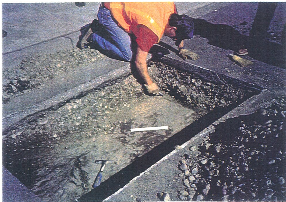
Figure 5.65 - Geotextile being cut prior to being removed.
