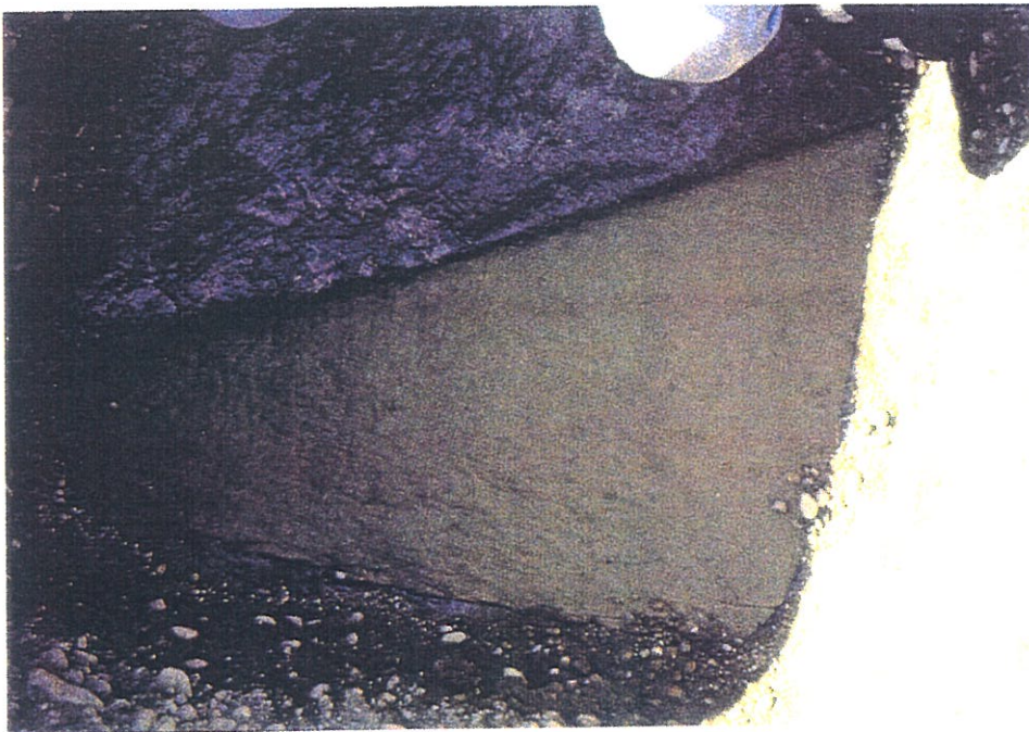
Figure 5.75 - Geotextile folded back exposing the subgrade surface.
