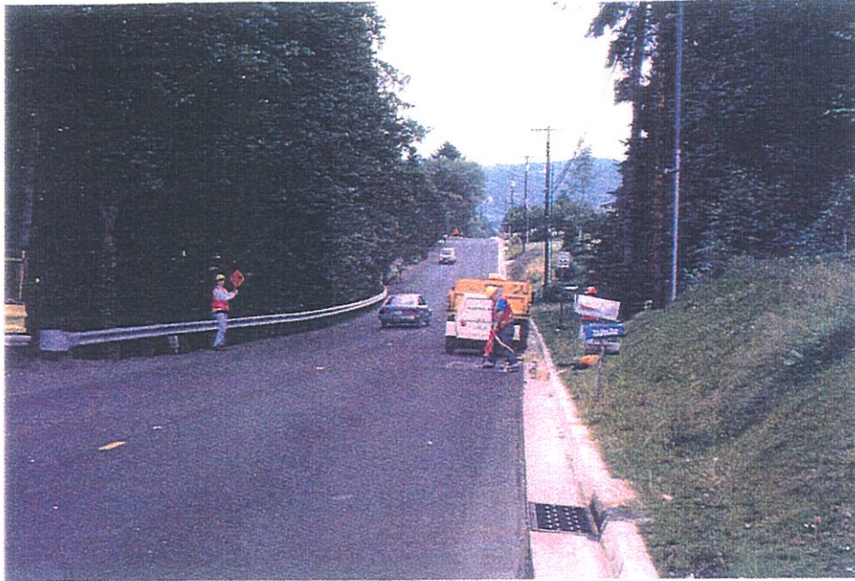
Figure 5.89 - Looking east towards the excavation on Olson Road.
