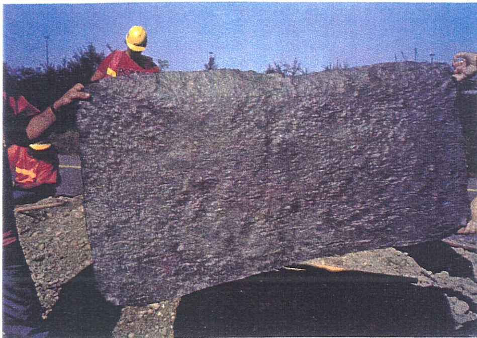
Figure 5.76 - Bottom surface of the exhumed geotextile.
