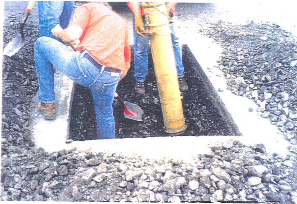
Figure 5.18 - Vac-all extension removing the ballast material.
