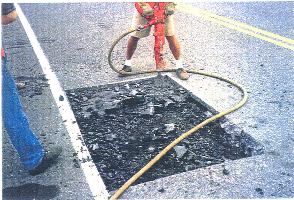
Figure 5.17 - Using the jack hammer to remove the ACP.
