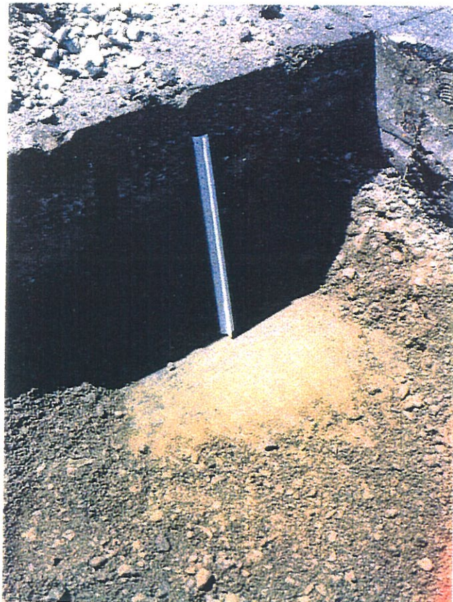
Figure 5.33 - Photograph showing exposed geotextile and pavement/base course section.
