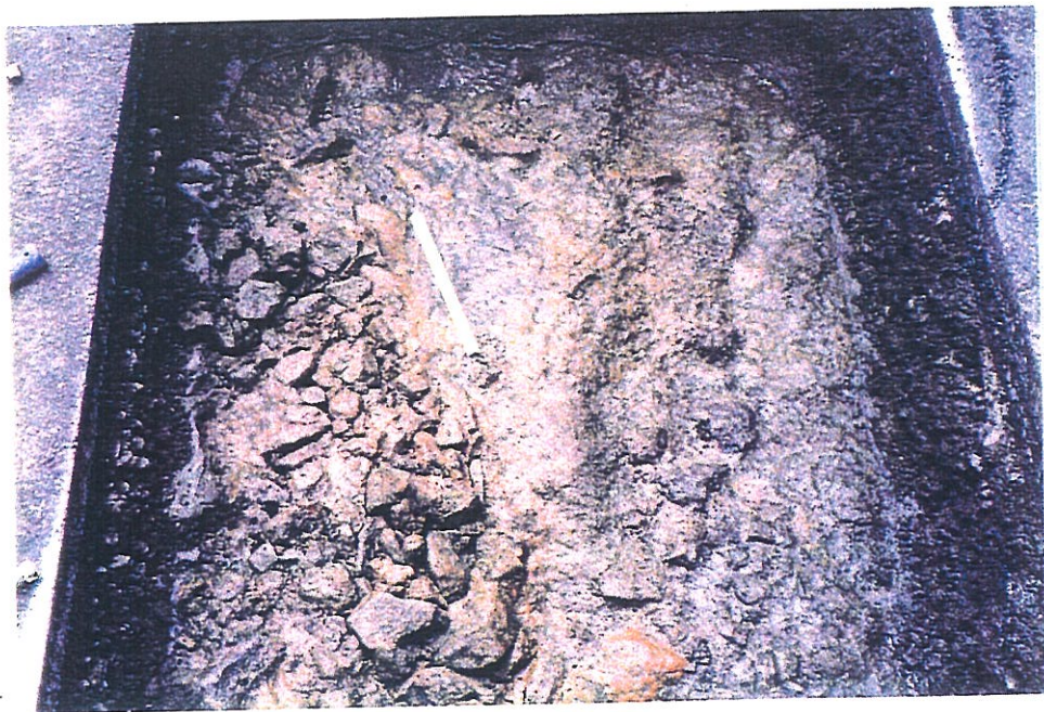
Figure 5.94 - Exposed subgrade surface. Looking west.
