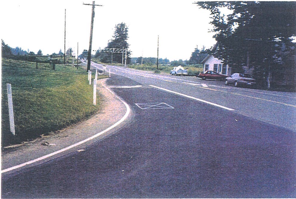
Figure 5.43 - Testpit location in the right turn pocket of SR-546.
