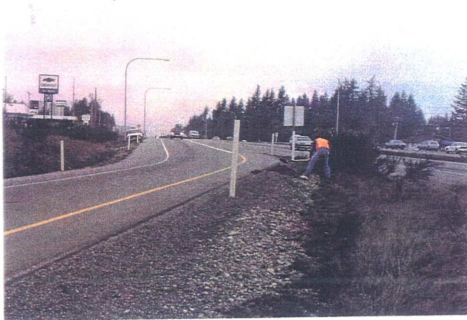
Figure 5.70 - Looking north at the south bound SR-16 off ramp.
