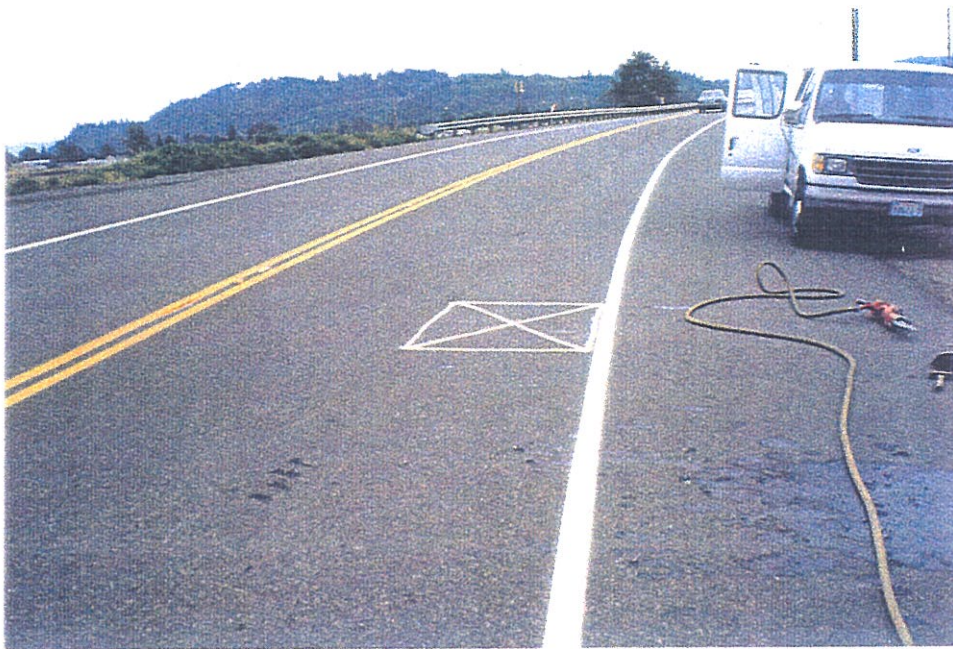
Figure 5.16 - Testpit location and pavement conditions.
