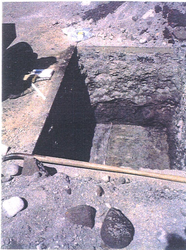
Figure 5.58 - Roadway section overlying the exposed geotextile.
