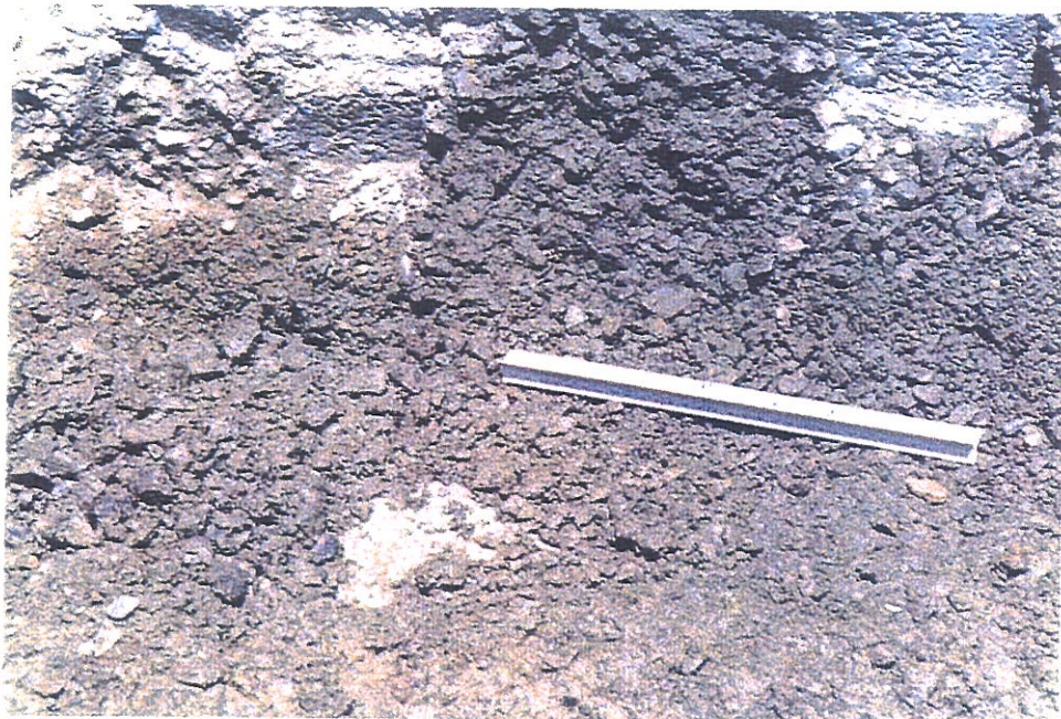
Figure 5.26 - Wet base course immediately above the geotextile.
