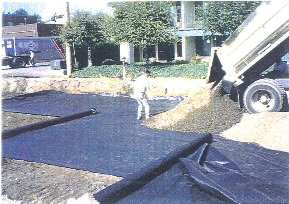
Figure 5.97 - Placement of base material during a recent and adjacent project.
