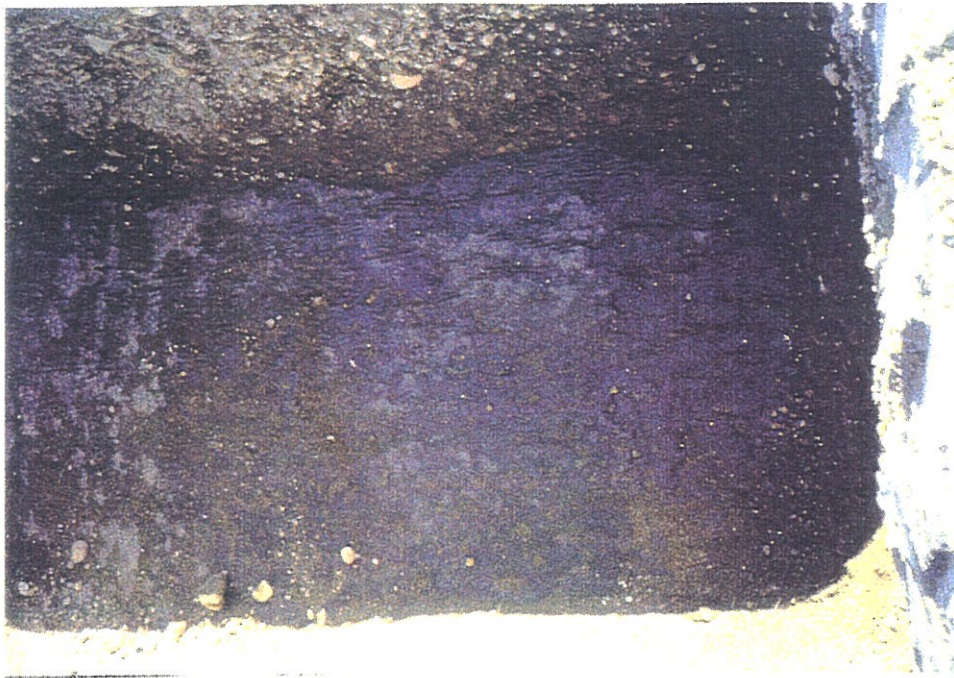
Figure 5.74 - Upper surface of the exposed geotextile separator.
