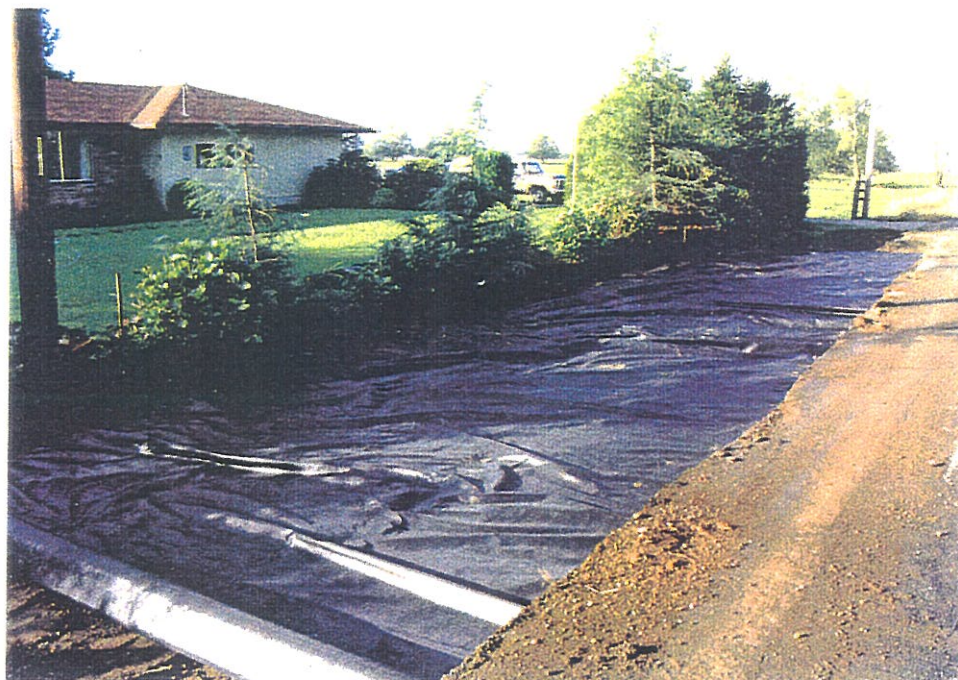
Figure 5.41 - Typical geotextile installation procedure for the turn pockets (Courtesy of WSDOT).
