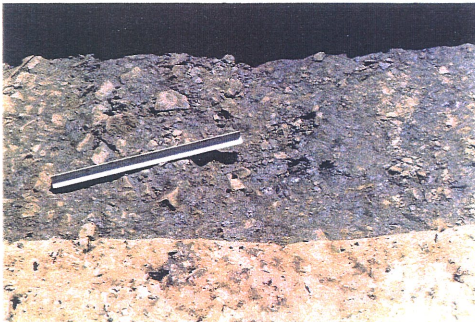
Figure 5.53 - Geotextile folded back revealing the gravelly subgrade.
