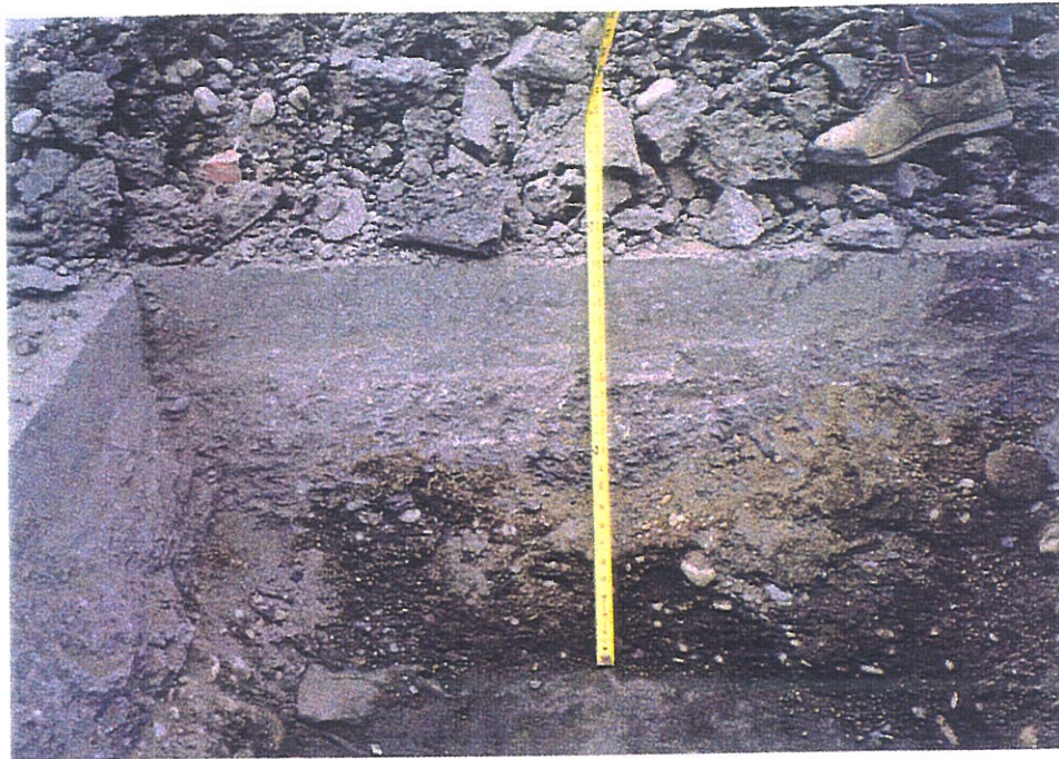
Figure 5.99 - Roadway section overlying the exposed geotextile.
