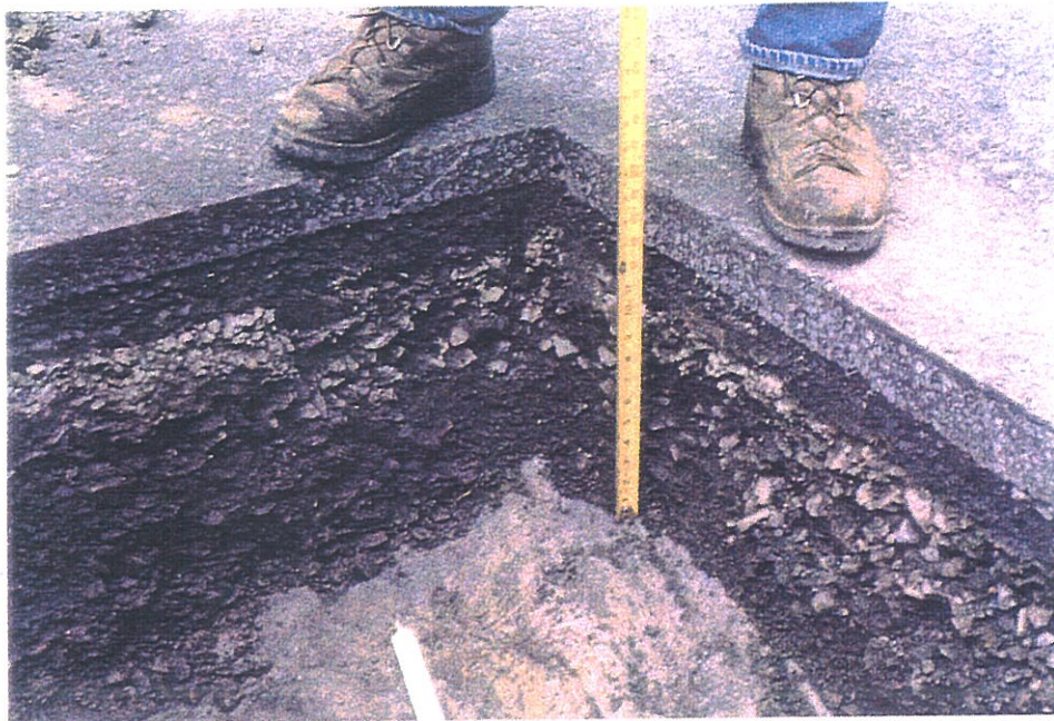
Figure 5.91 - Roadway section overlying the exposed geotextile.
