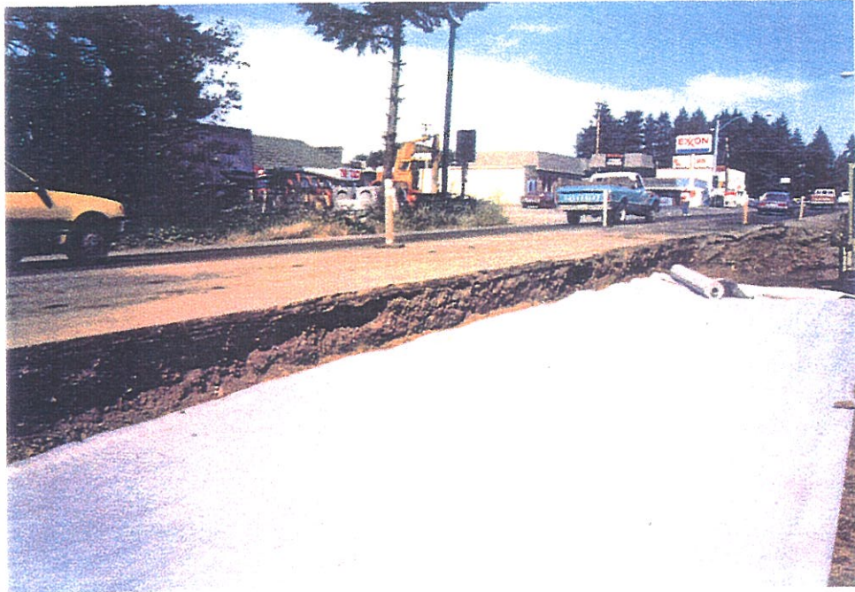
Figure 5.78 - Geotextile rolled out over prepared subgrade during construction (Courtesy of WSDOT).
