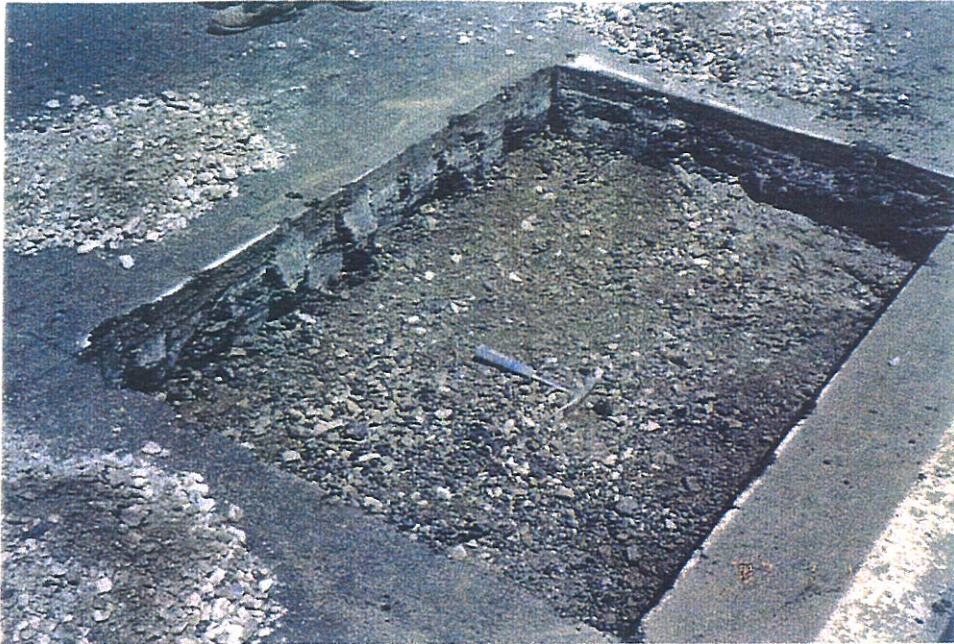
Figure 5.32 - Photograph of excavation with asphalt concrete removed.
