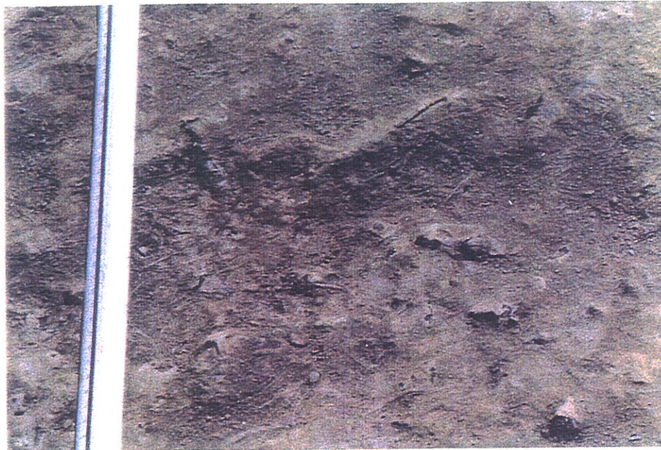
Figure 5.52 - Close-up of the geotextile showing gravels in the subgrade penetrating up through the fabric.
