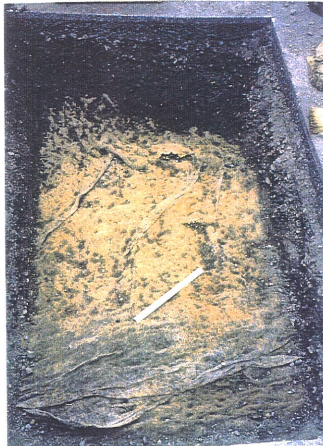
Figure 5.4 - Surface of the exposed geotextile showing folds and overlap (bottom).
