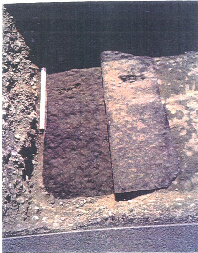
Figure 5.66 - Geotextile folded back exposing the subgrade surface.
