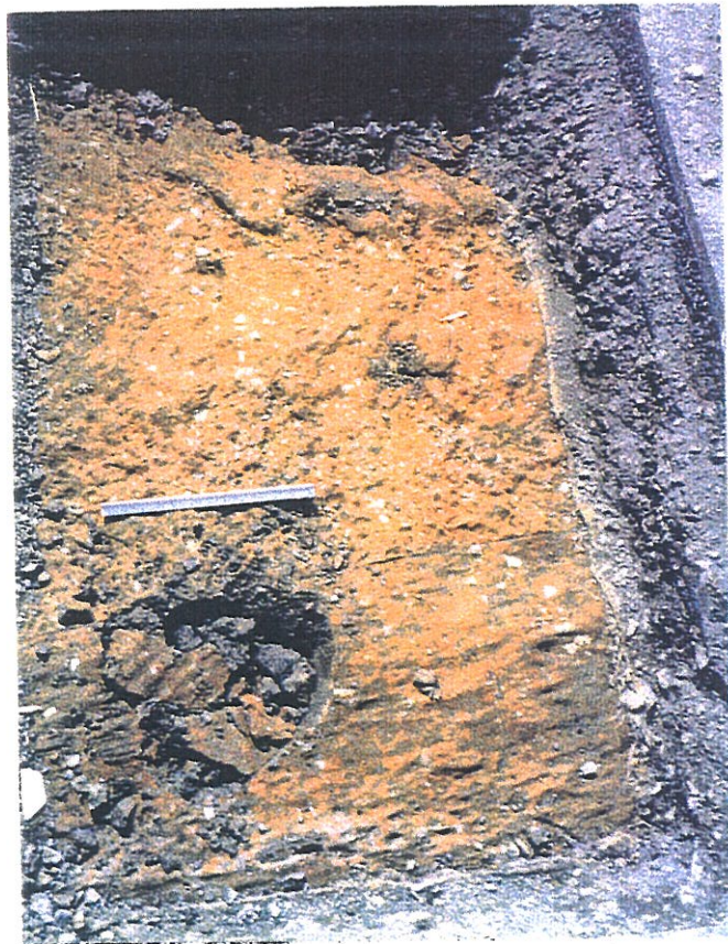
Figure 5.6 - Subgrade surface after subgrade samples had been taken, testpit 1a.
