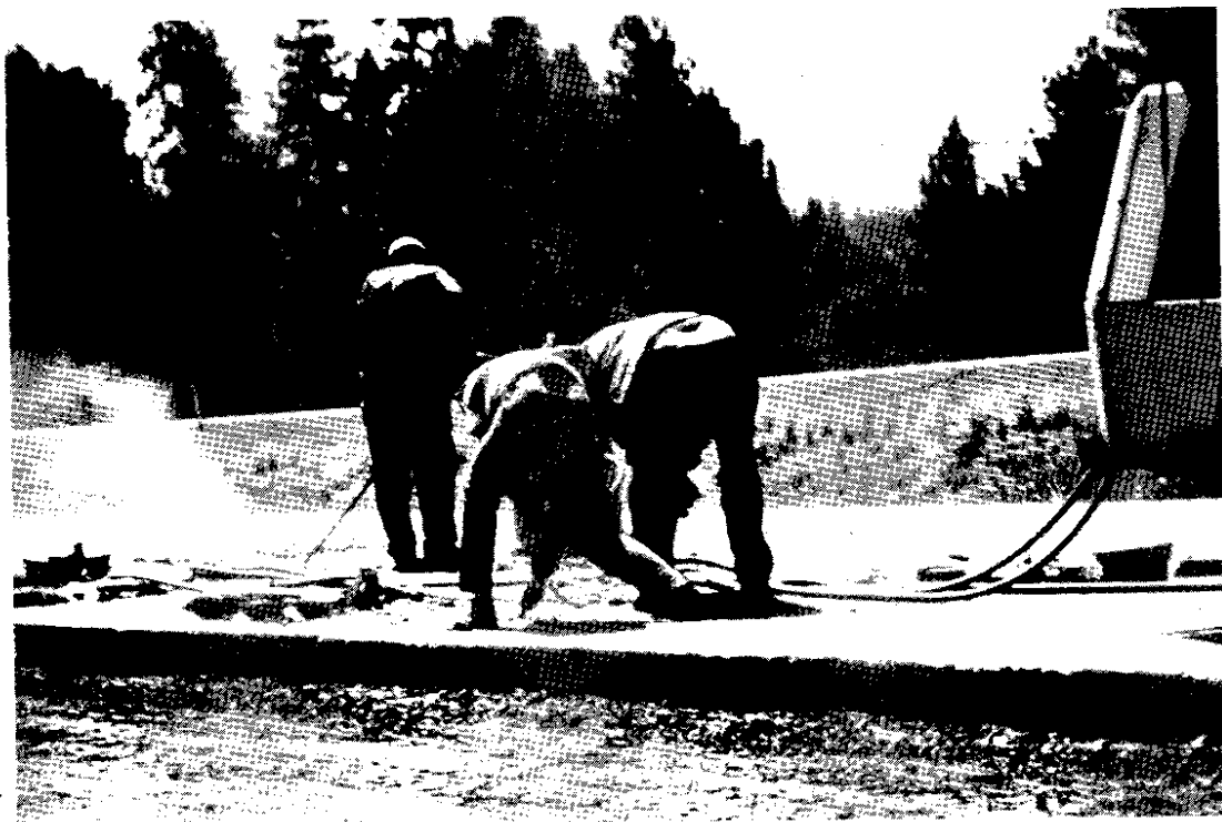
Picture 10. Removing concrete from dowel bar slots.
