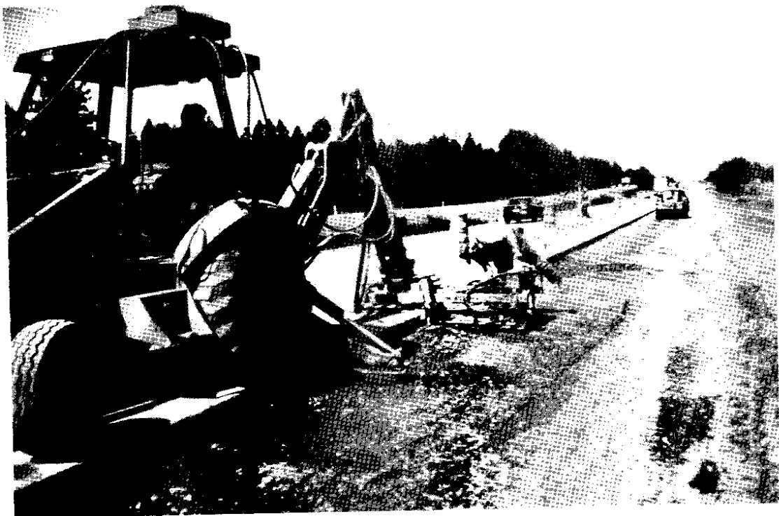
Picture 5. Hole drilling operation for tie bar placement.
