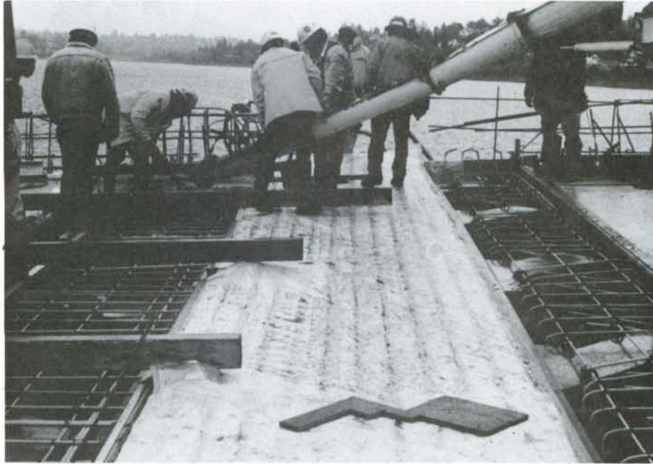
Pouring Concrete into Pontoon Expansion Joint Rebar
