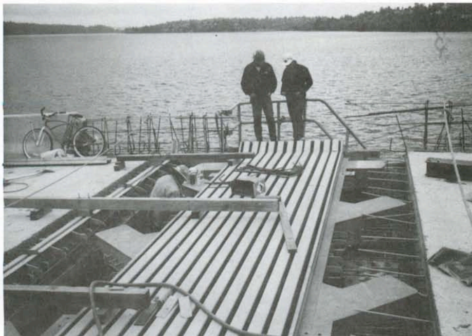
Pontoon Expansion Joint in Blockout
