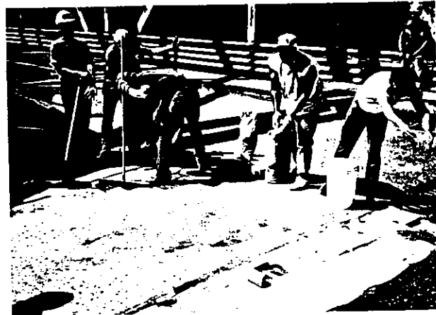
FIGURE 7 Hand broadcast of aggregate.
