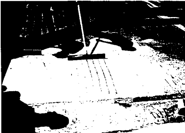
FIGURE 6 MMA spread with gage rake.
