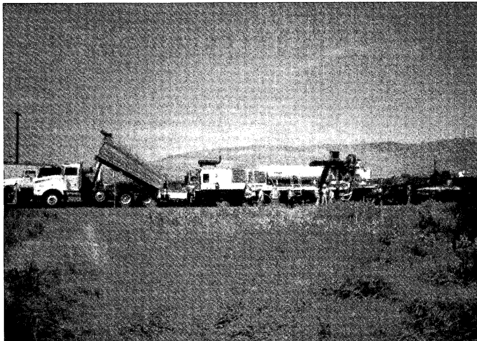
Picture 7. Truck delivering precoated aggregate, "Unit B", and conventional paving machine.
