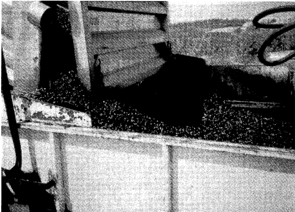
Picture 9. Addition of pre-coated material into hopper of "Unit B"..
