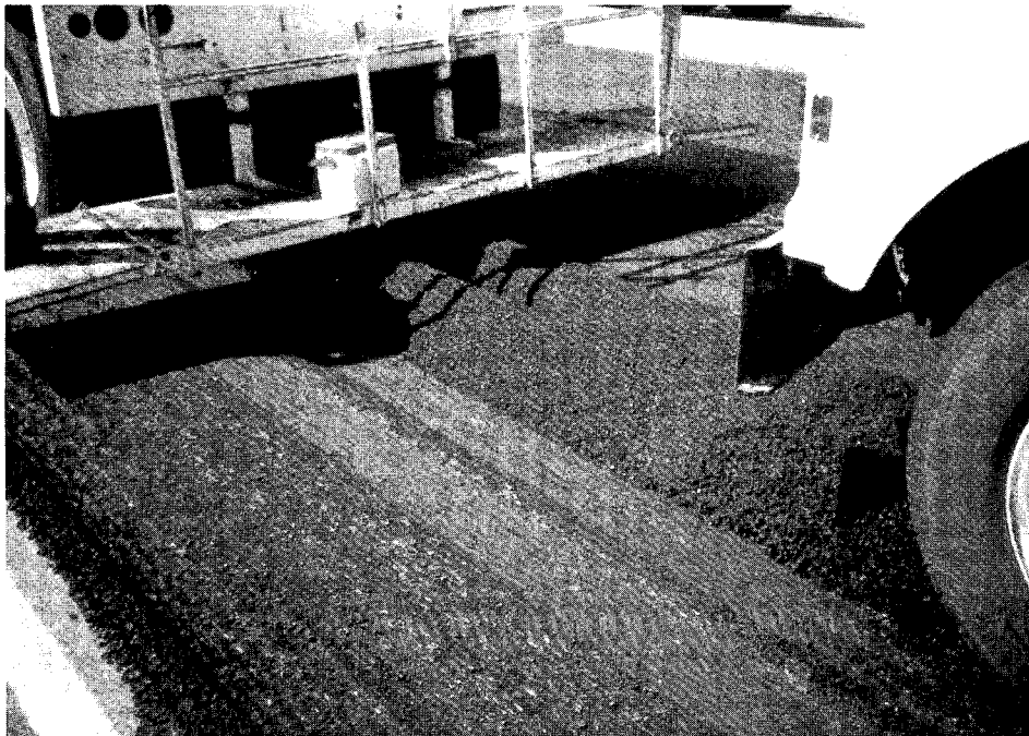
Picture 6. Milled and windrowed material after "Unit A".
