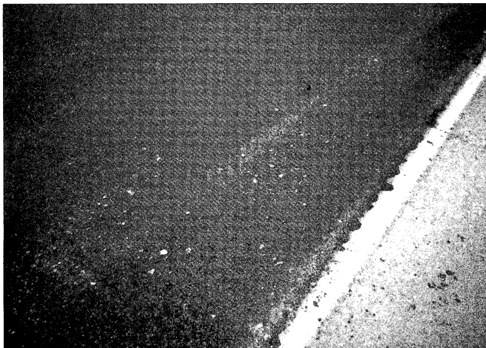
Picture 15. Close up of uncoated aggregate in HIPR material.
