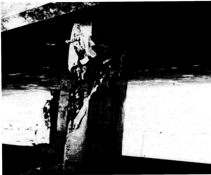
Figure 1.1-4: Cable Restrainers
