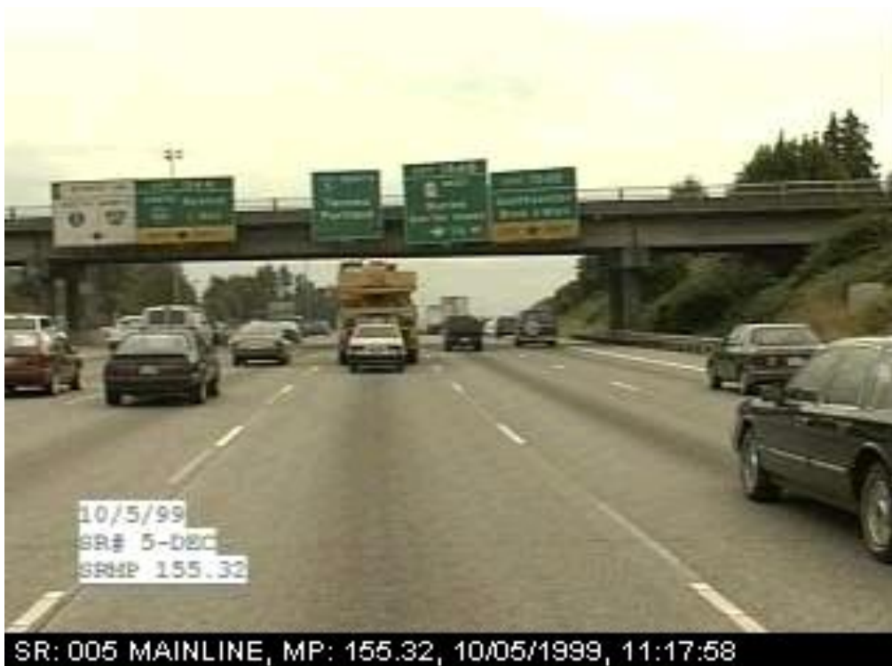
Figure 25. I-5 southbound at Southcenter near an independent alignment
