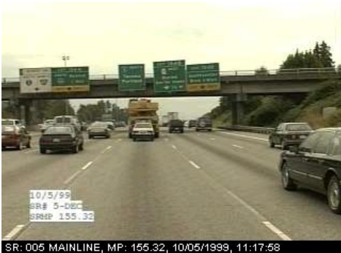
Figure 13: I-5 southbound at Southcenter near an independent alignment
