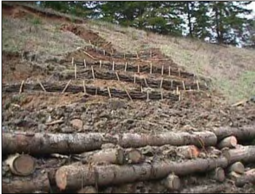
Figure 17. Live cribwall and willow walls
