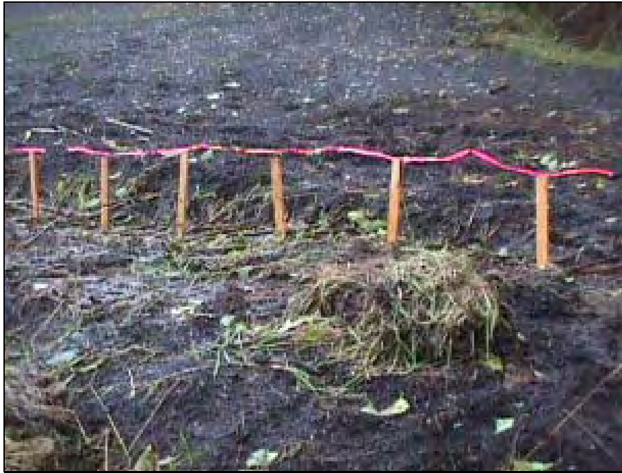
Figure F-3. Site 3 - Stakes placed below level terrace marking tape
