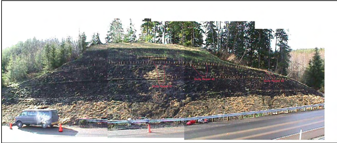
Figure 10. Site 3 immediately after construction
