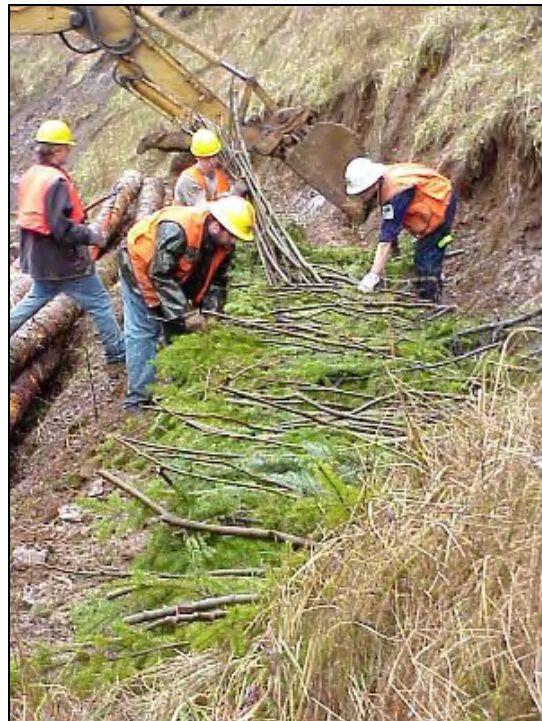
Figure 13. Cordon construction
