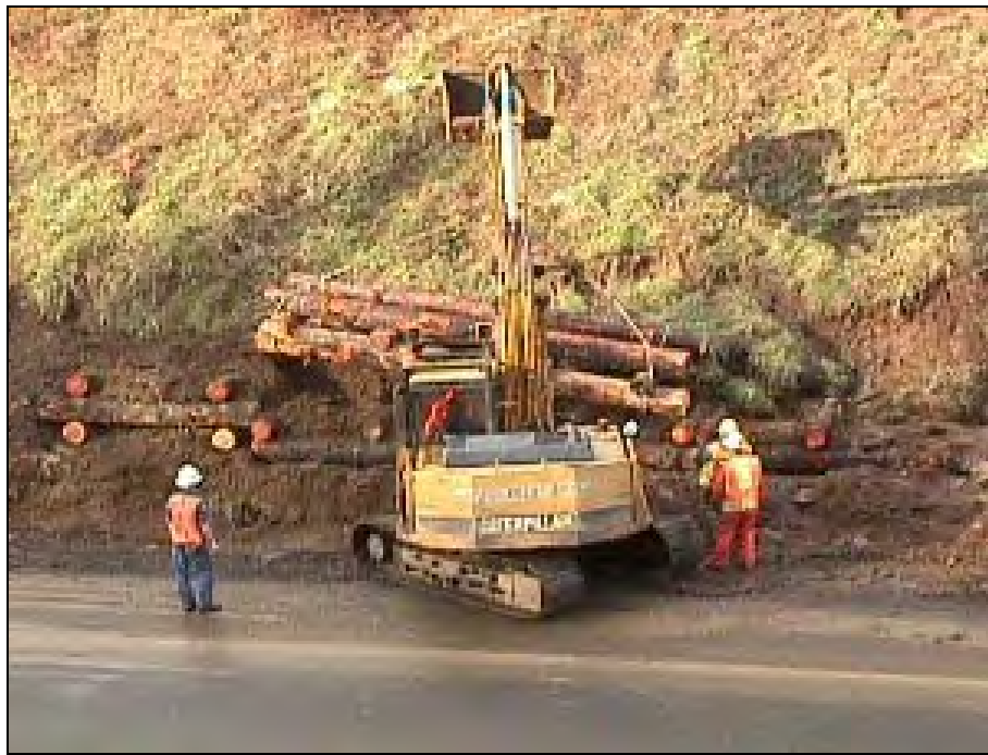
Figure 16. Installation of modular live cribwall sections
