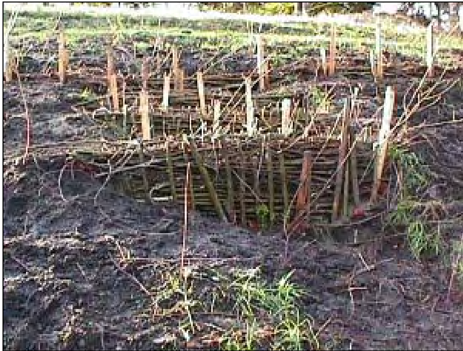
Figure 9. Branch packing parallel to contours
