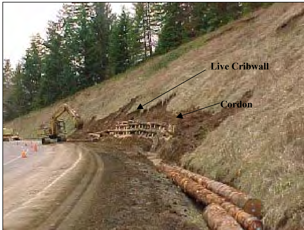
Figure 14. End of first week of construction.
