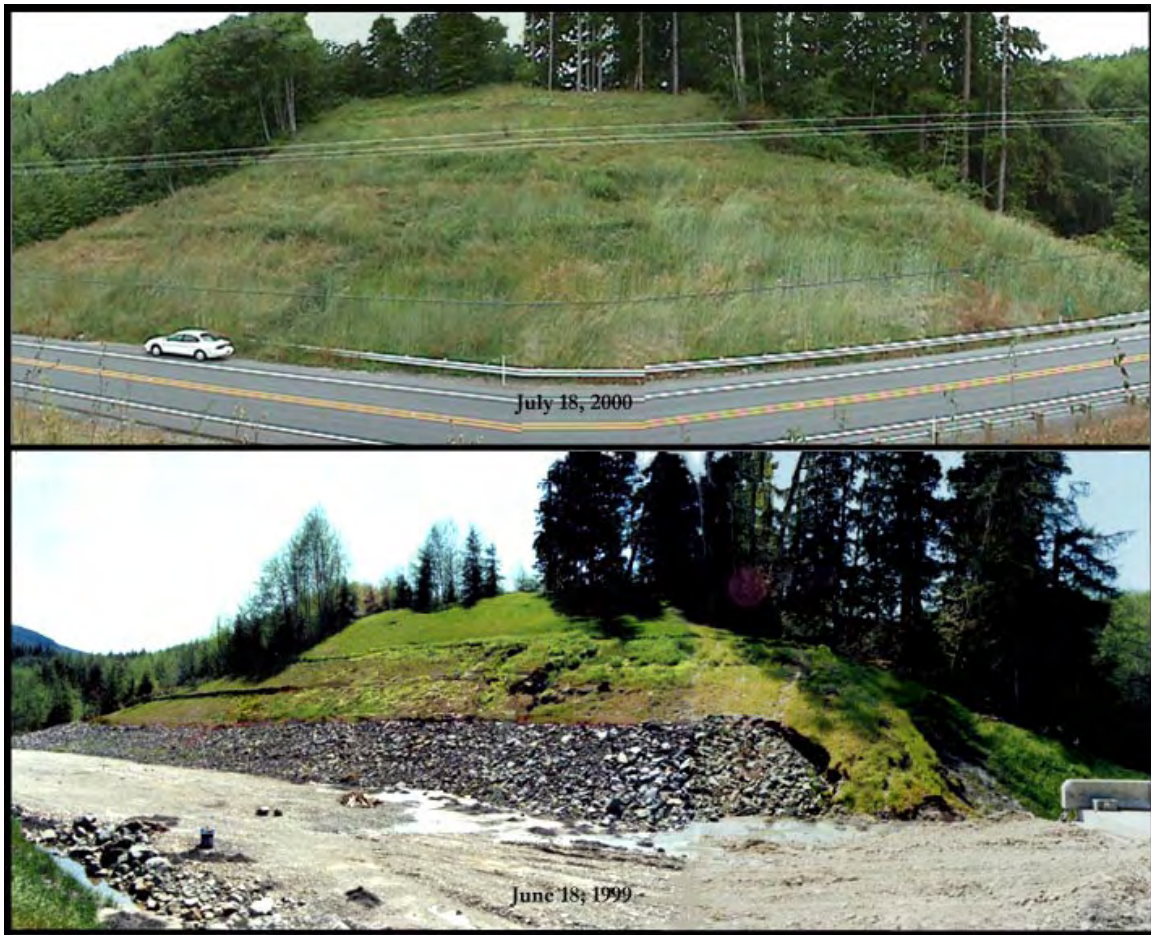
Figure 23. Site 3 Before and after soil bioengineering
