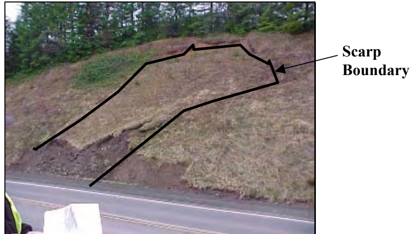
Figure 11. Area of instability
