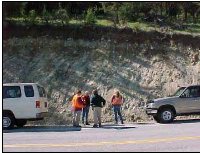
Figure 1. SR 971, Mile Post 8.22 vicinity, June 1999
