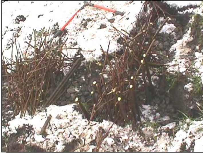
Figure 22. Branch packing parallel to slope contours.
