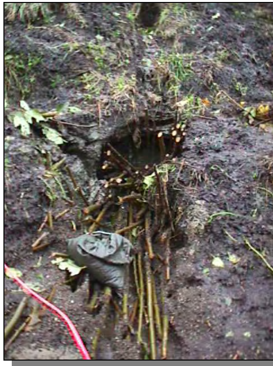
Figure 21. Brushlayers failed when placed perpendicular to the slope.
