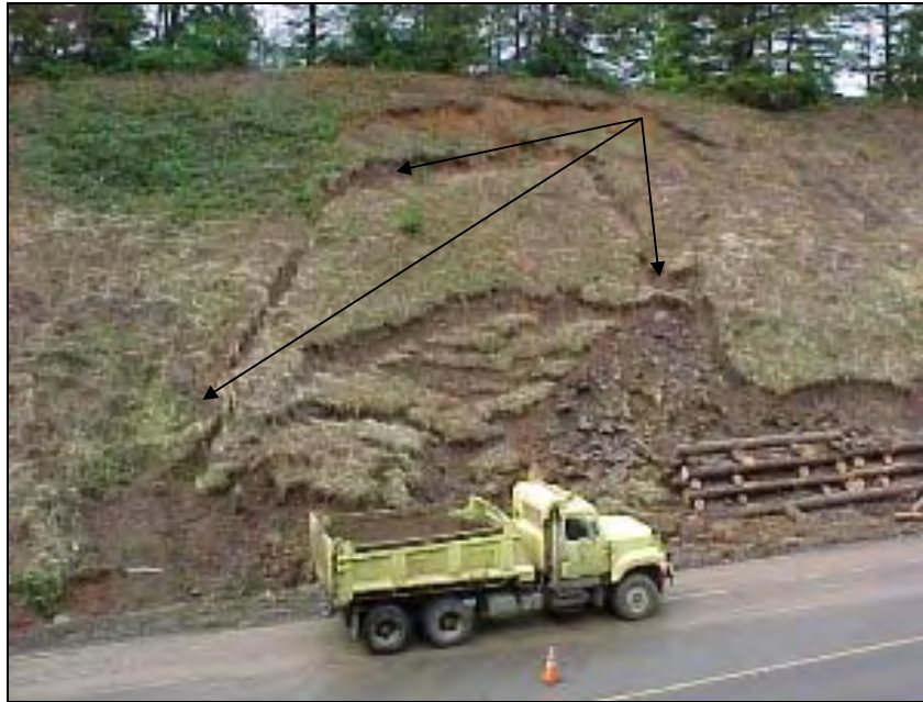
Figure 15. Slope failure
