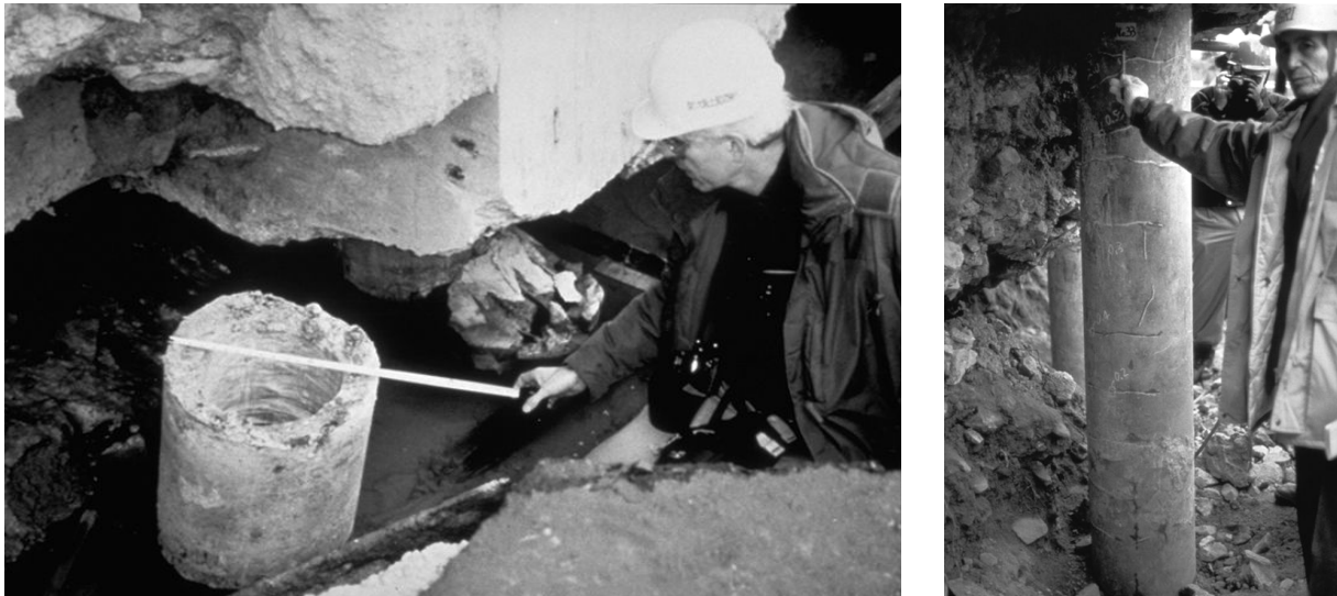
Figure 4.17. Pile damage due to lateral spreading in Kobe, Japan (from Izmit Collection, Earthquake Engineering Research Center, University of California, Berkeley).
