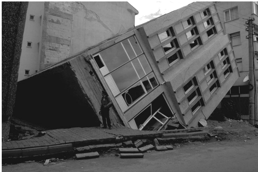
Figure 4.13. Liquefaction-induced bearing capacity failure in Adapazari, Turkey (from Izmit Collection, Earthquake Engineering Research Center, University of California, Berkeley).
