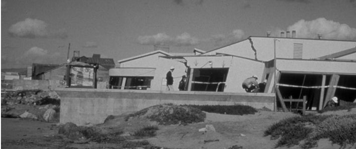
Figure 4.14. Damage to Monterey Bay Aquarium Research Institute following 1989 Loma Prieta earthquake.
