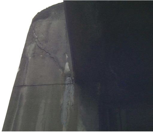
Figure 3.3. Damage to bent 100 knee joint immediately after the 2001 earthquake
