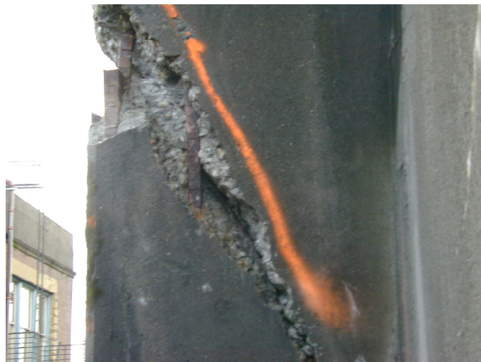
Figure 3.4. Damage to bent 100 knee joint of Alaskan Way Viaduct one month after the 2001 earthquake
