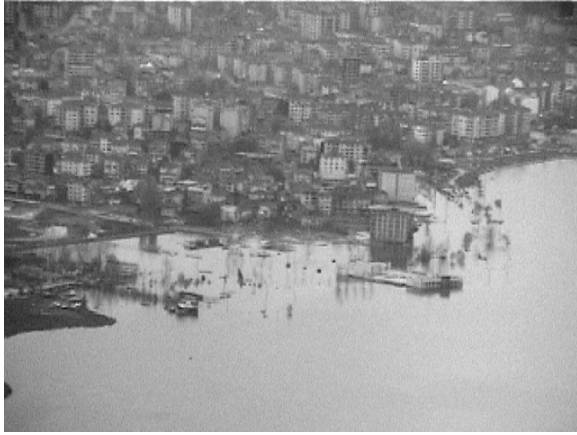
Figure 4.10. Coastal flooding due to liquefaction-induced subsidence in Golcuk (from Izmit Collection, Earthquake Engineering Research Center, University of California, Berkeley)
