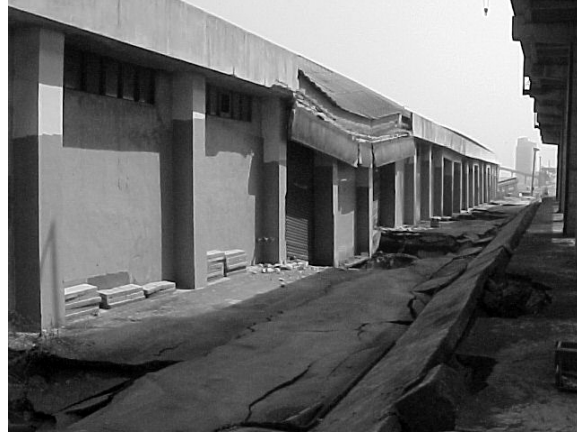
Figure 4.11. Structural failure due to liquefaction-induced settlement of isolated footing at Port of Taichung (from Izmit Collection, Earthquake Engineering Research Center, University of California, Berkeley)
