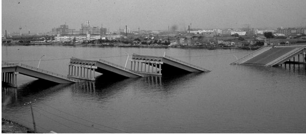
Figure 4.16. Failure of Showa River bridge in Niigata, Japan, due to lateral spreading.
