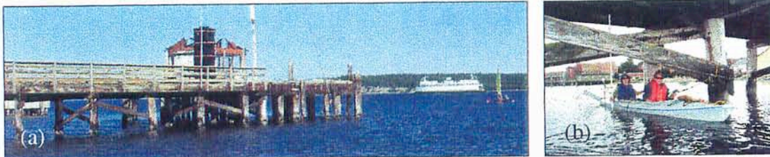
Figure 7. (a) Sun Tunnel installed at the existing dock in Port Townsend, Washington; (b) Measuring light under the dock.
