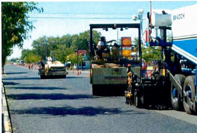
Photo 15. Rolling (seating) the NovaChip® surface.
