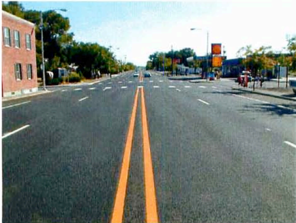
Photo 24. Soap Lake – Final NovaChip® surface.
