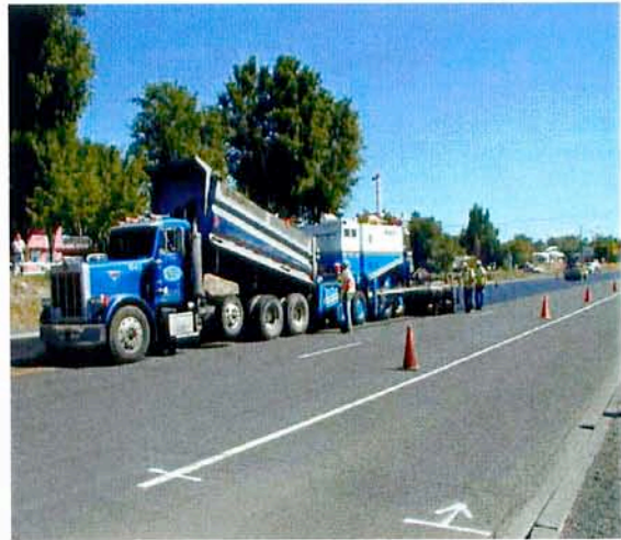
Photo 14. NovaChip® paving operation.
