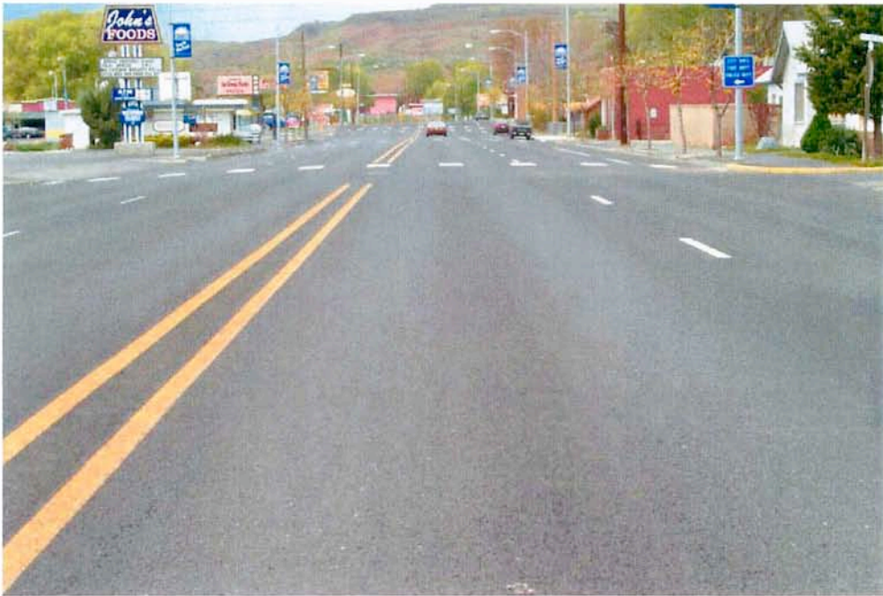
Photo 26. NovaChip® overlay through Soap Lake – May 2003.
