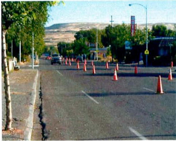
Photo 13. Traffic control in place.
