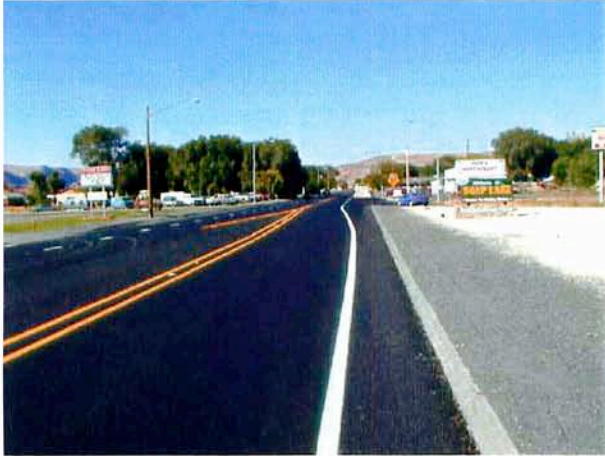
Photo 22. Soap Lake – Final NovaChip® surface.
