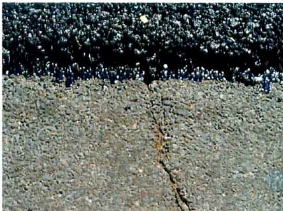
Photo 8. NovaChip® asphalt placed over existing transverse cracks.
