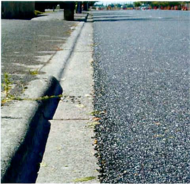
Photo 11. NovaChip® asphalt placed adjacent to curb and gutter.
