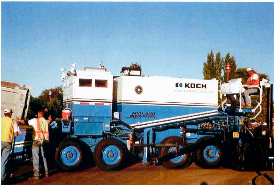
Photo 1. Novachip Paving Machine.
