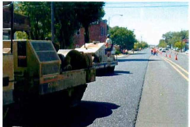
Photo 21. Compaction was completed with a 15 ton breakdown roller and 12 ton finish roller.
