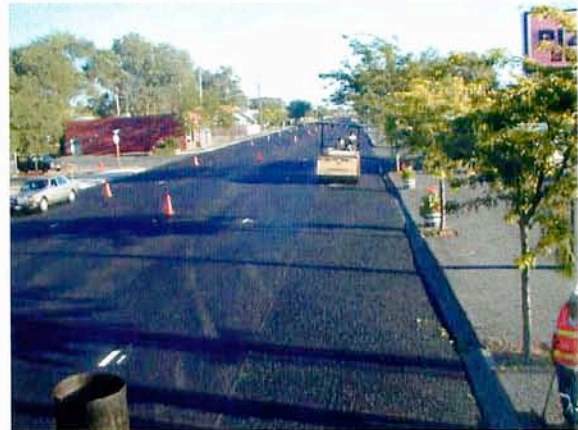
Photo 16. Compaction of the NovaChip® roadway surface.
