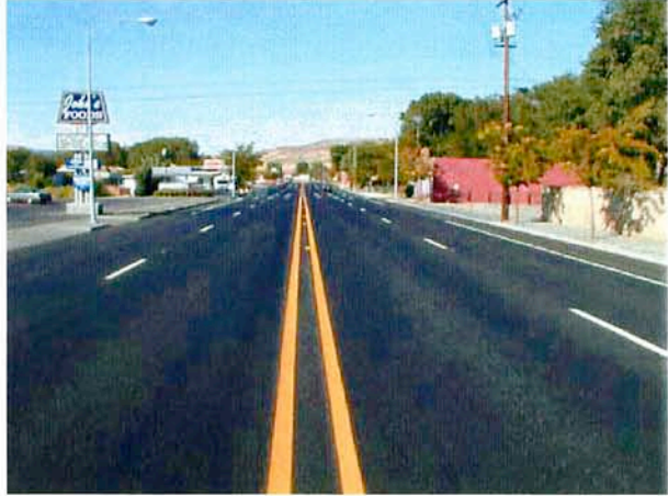
Photo 23. Soap Lake – Final NovaChip® surface.
