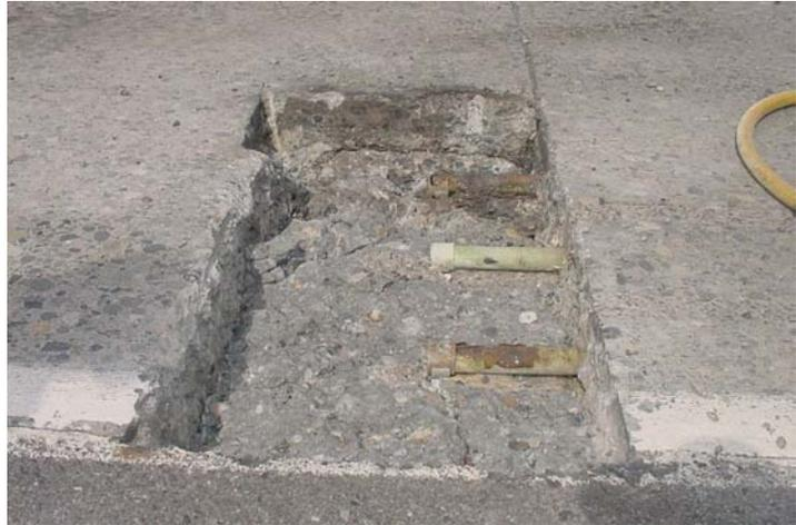
Photo 26. Epoxy coated dowel bars that have corroded possibly due to improper handling.
