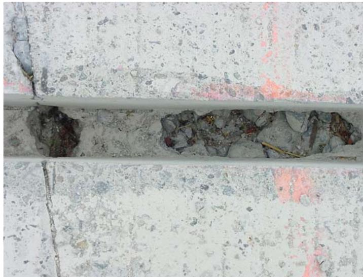
Photo 37. Patching material was poorly consolidated beneath the dowel bar, which may result in pop out of patching material.
