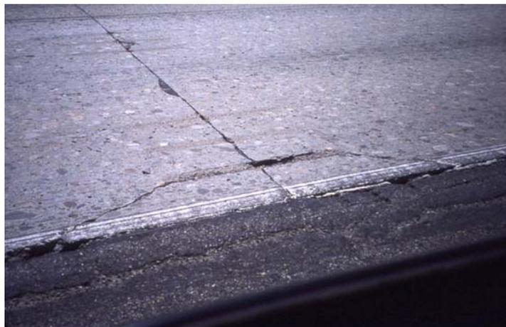
Photo 5. Corner cracking resulting from traffic loading when sawcuts penetrate too deep in the concrete roadway.
