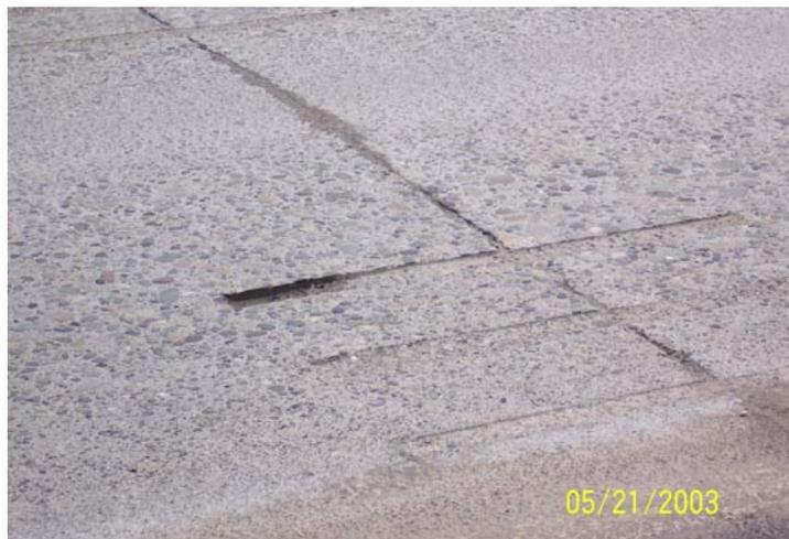
Photo 38. Opening to traffic prior to proper curing of patching material.
