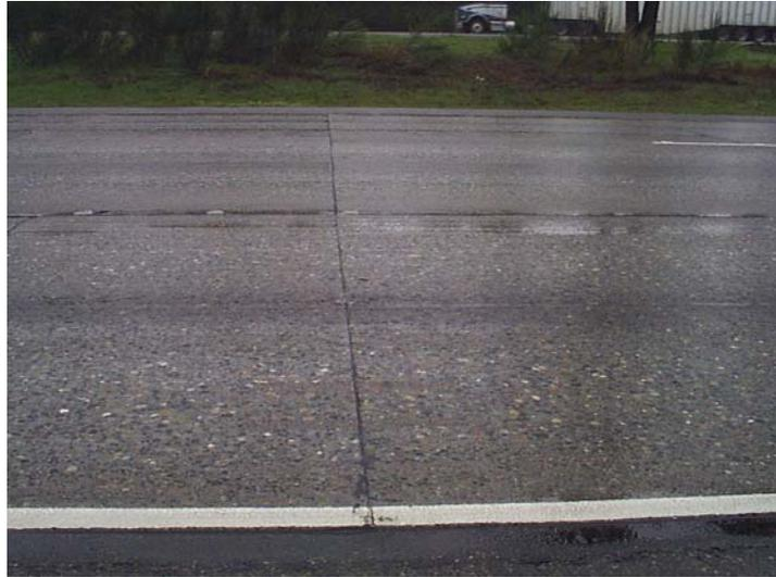
Photo 39. Diamond ground surface. The transverse crack has not been damaged.
