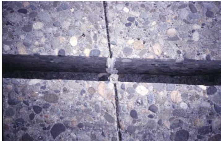
Photo 19. Slot has been caulked with silicon sealant.
