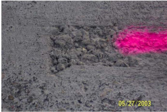
Photo 35. Segregated patching material, which may lead to additional spalling and cracking.
