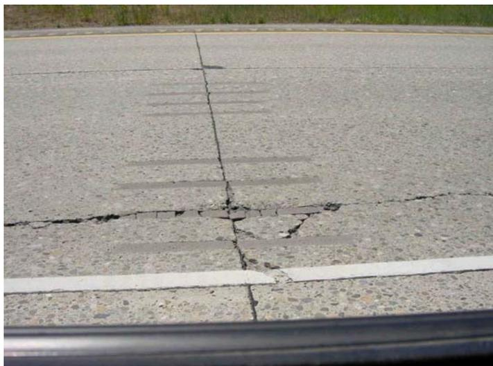
Photo 6. Existing longitudinal crack that intersected a dowel bar retrofit slot.
