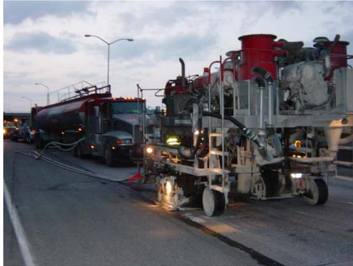
Photo 1. Saw cutting slots.
