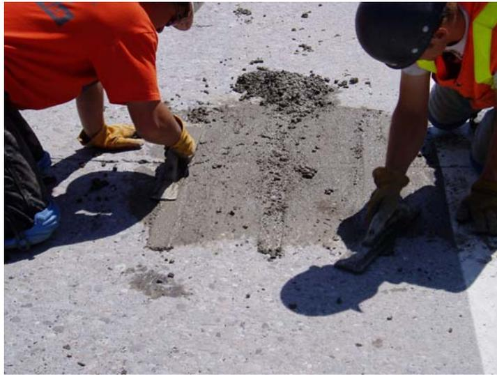
Photo 32. Finishing patching material.
