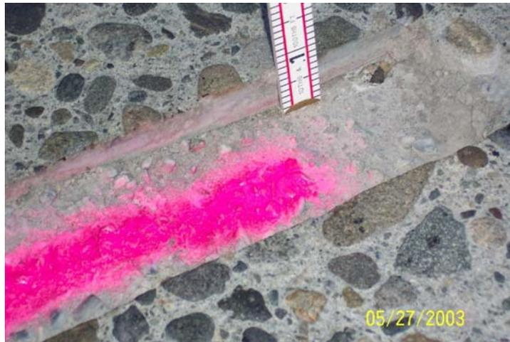
Photo 36. Patching material placed too low, results in poor ride quality and may cause cracking due to insufficient cover on bar.
