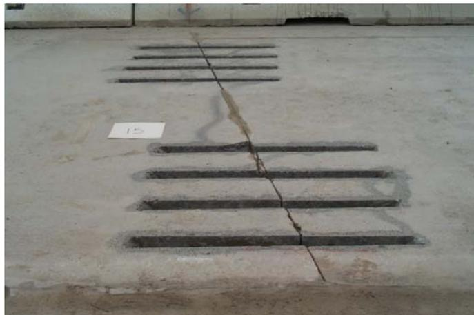
Photo 3. Dowel bar retrofit slots placed parallel to centerline over a skewed joint.
