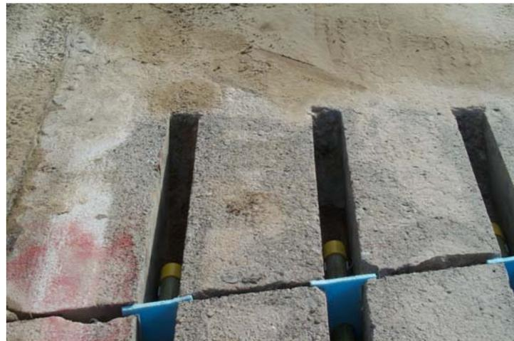
Photo 17. Sandblasting debris adjacent to slots should be cleared to avoid contamination during placement of patching material.
