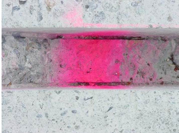
Photo 10. Concrete improperly removed from the bottom of the slot.
