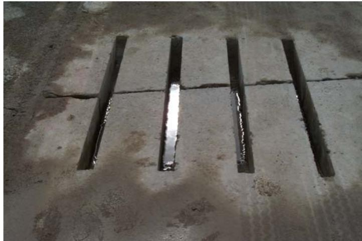
Photo 16. Removal of water, from slots, is required prior to placement of patching material.
