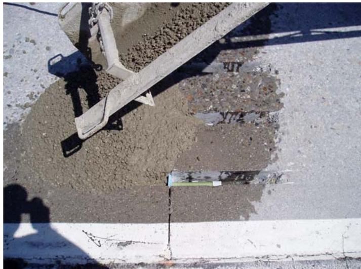
Photo 29. Placing patching material.
