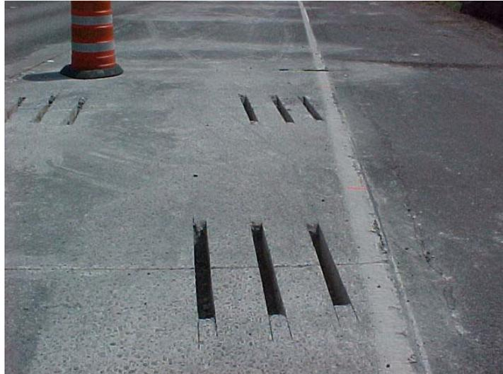
Photo 4. Slots should not be placed perpendicular to skewed joints.
