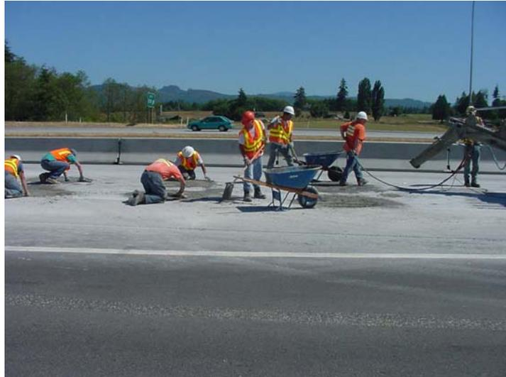
Photo 28. Placing patching material.
