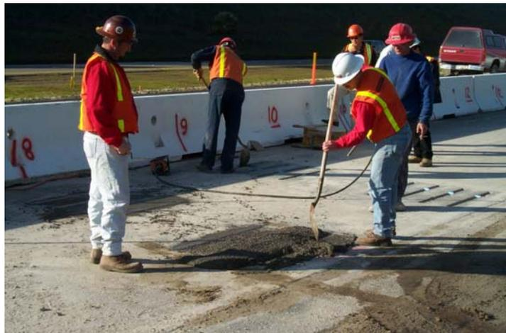
Photo 30. Shoveling patching material into slots.
