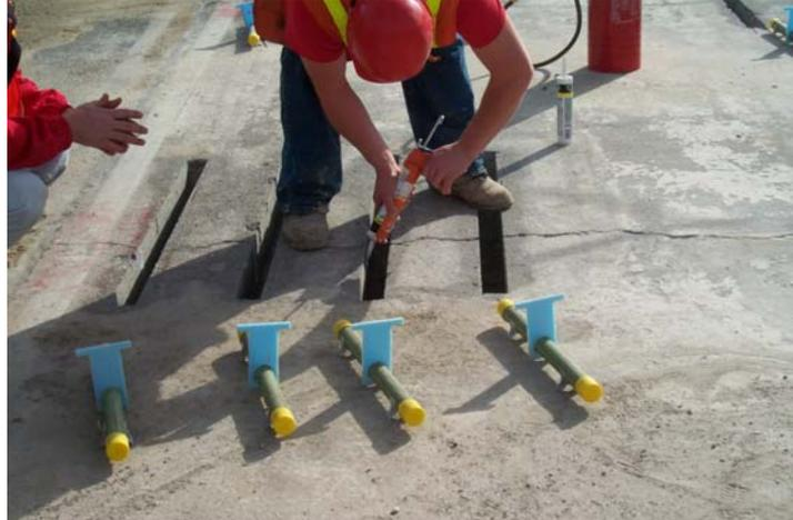
Photo 18. Caulking should be placed along the sides and bottom of the slots.
