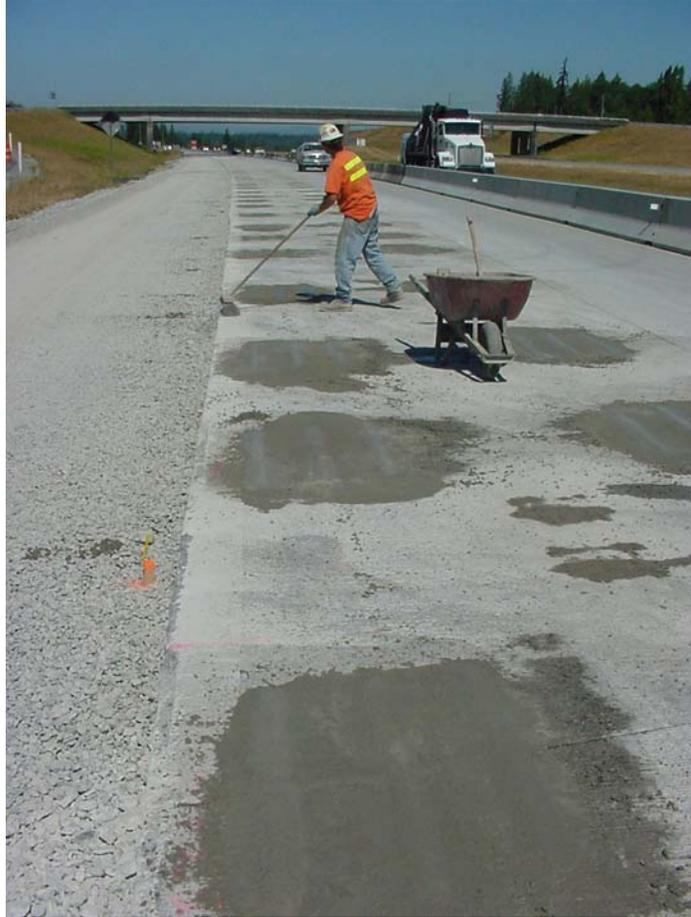
Photo 34. Completed placement of patching material.
