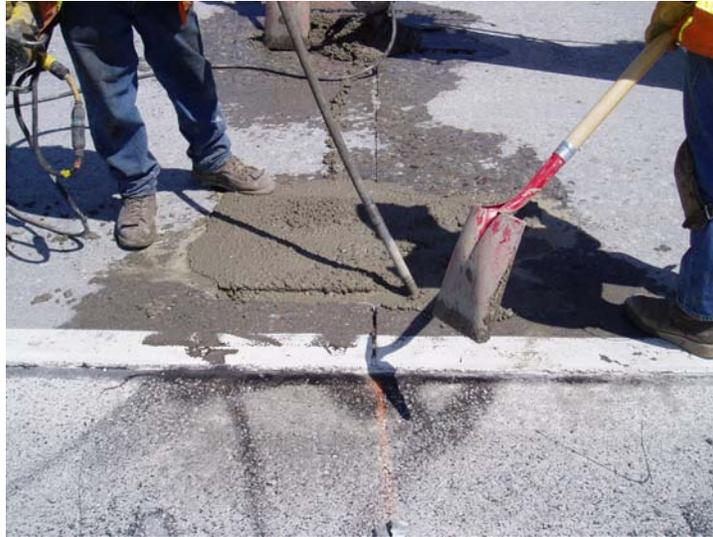
Photo 31. Consolidating patching material.
