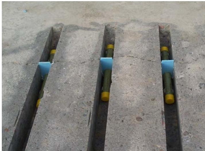
Photo 22. Dowel bars that have been placed and aligned in slots over a transverse crack.
