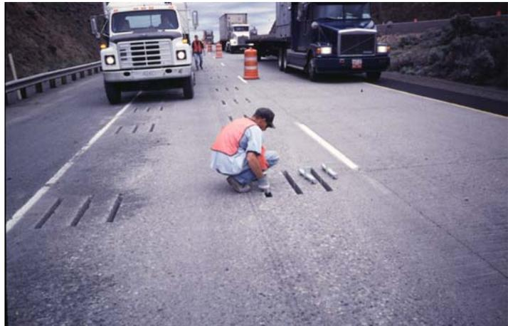
Photo 21. Dowel bar assemblies are placed into slots.
