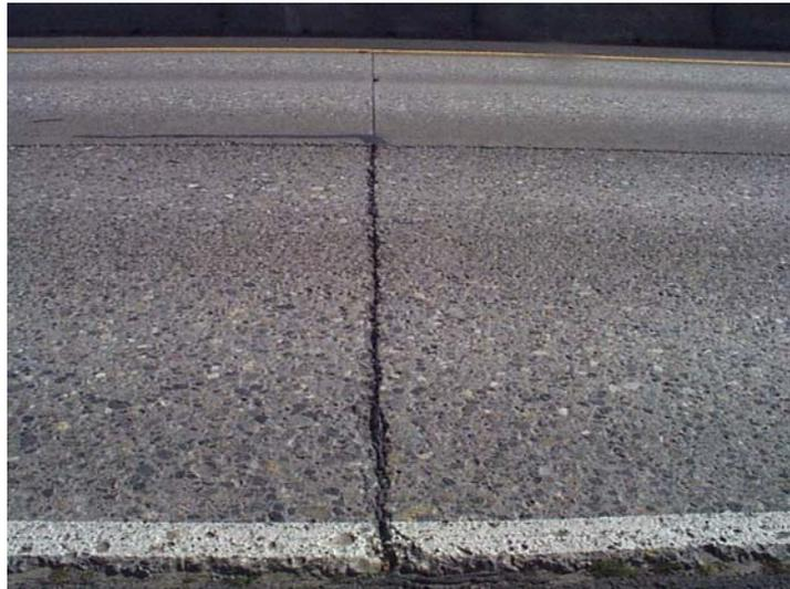
Photo 40. Rotomilled surface. The transverse joint has been damaged due to the impact of the rotomill on the concrete.
