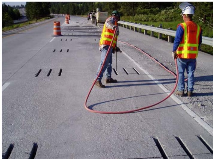
Photo 14. Cleaning slots with compressed air.
