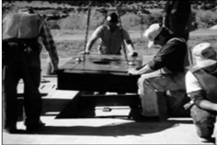
Figure 2-12. Single load cell installation (from International Road Dynamics Inc., www.irdinc.com )
