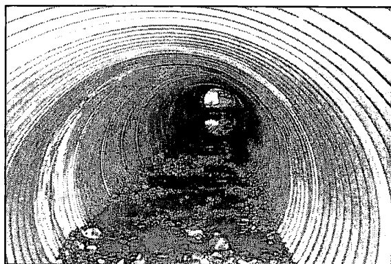
Figure 2. Example Culvert. (Note: this replacement culvert has not been re-watered.)
