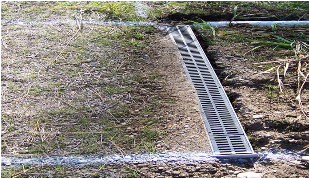
Figure 9. Slot Drain Installation
