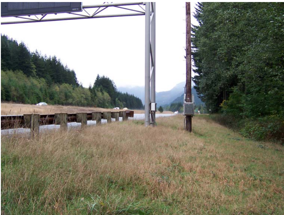
Figure 5. I-90 Remote Monitoring Site (North Bend)
