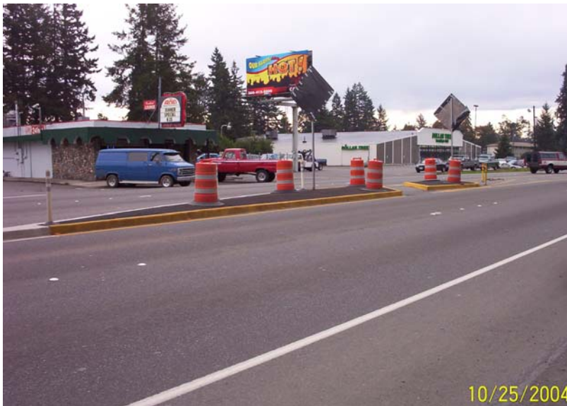
Figure 4. Pedestrian refuge islands at S. 180 th Street and SR 7
