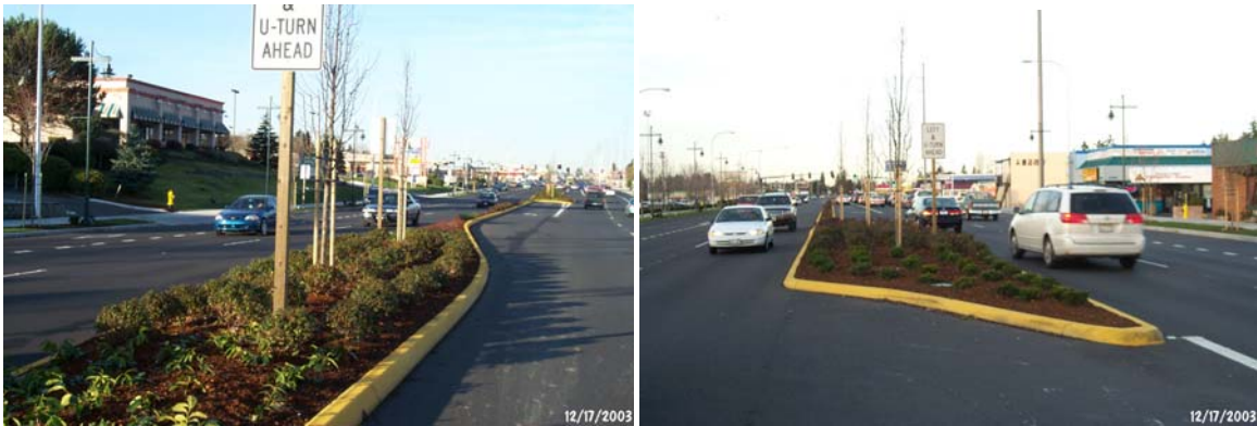
Figure 6-4. Federal Way Phase 1 – Completed Project with Left-Turn Pockets. Note Narrow Medians without Trees
