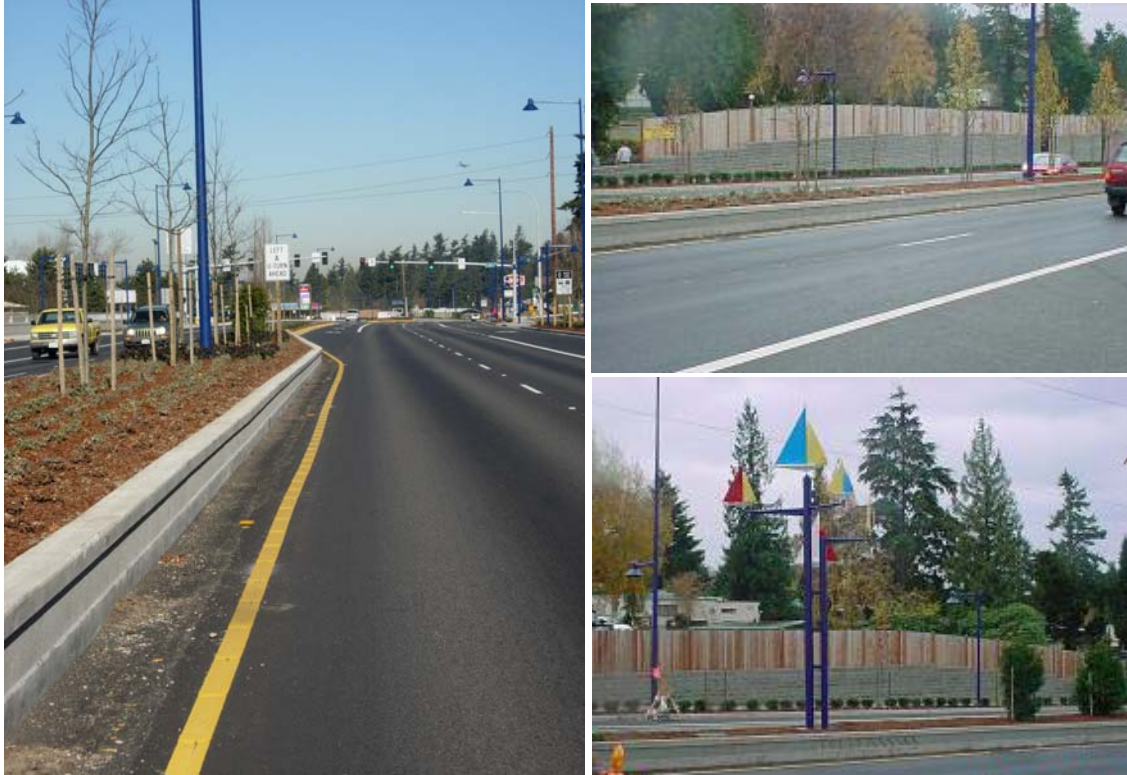
Figure 7-4. Des Moines – Low-Profile Median Barrier to Mitigate the Effects of Trees and Decorative Objects
