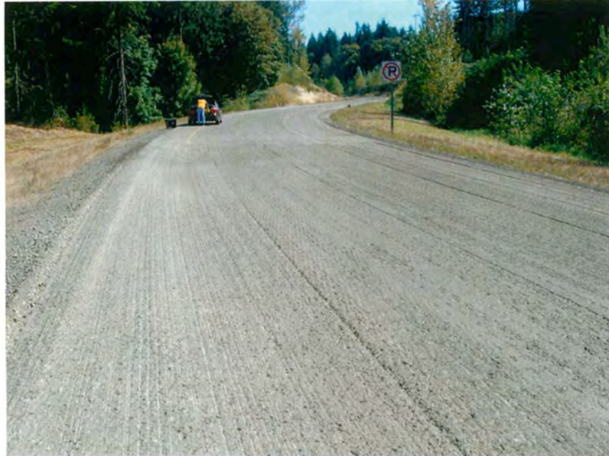
Figure 3.2: Milled and non-milled sections after cleaning.
