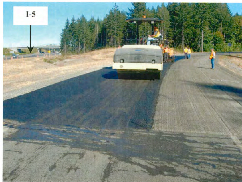
Figure 3.3: Compaction and paving of sections number 1 and 3, respectively.
