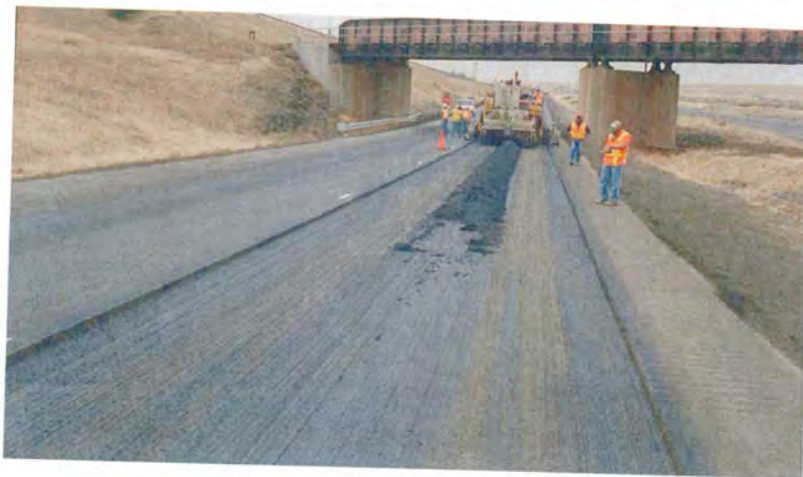
Figure 2.1: Tracking due to the presence of debris.
