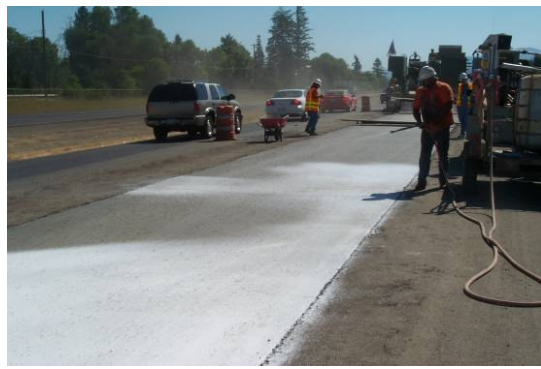
Image A. Hand application of curing compound.
