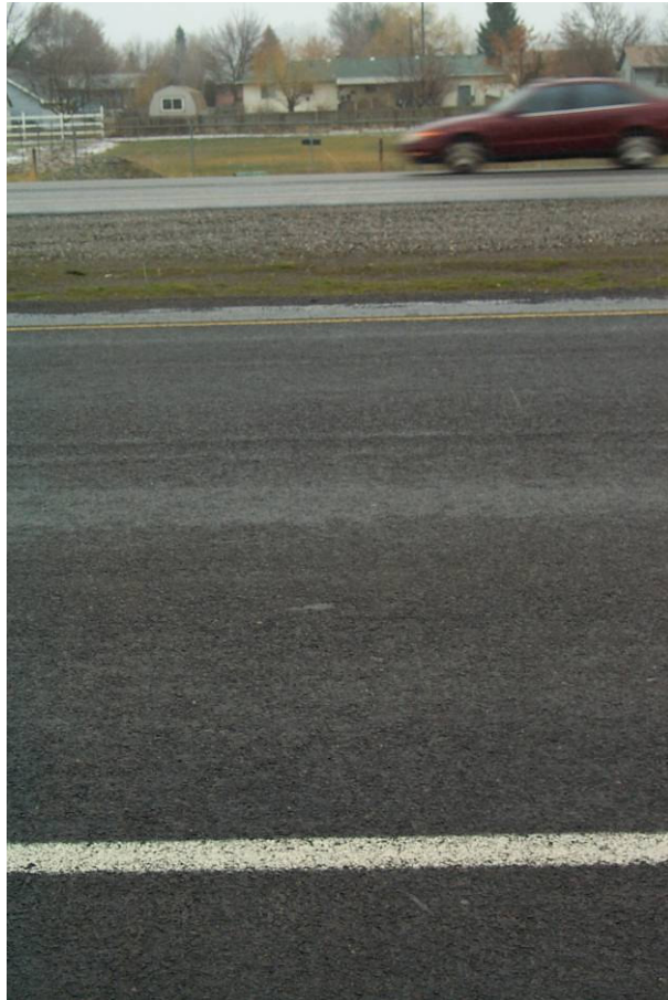
Image 6. Surface texture of the Macro Surfacing.
