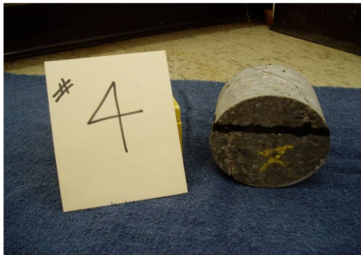
Figure 8. End view showing panel joint and cracks. August 2004
