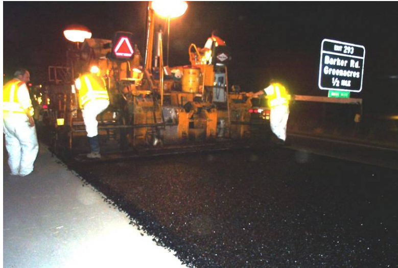
Figure 5. Paving of Modified Class D mix.
