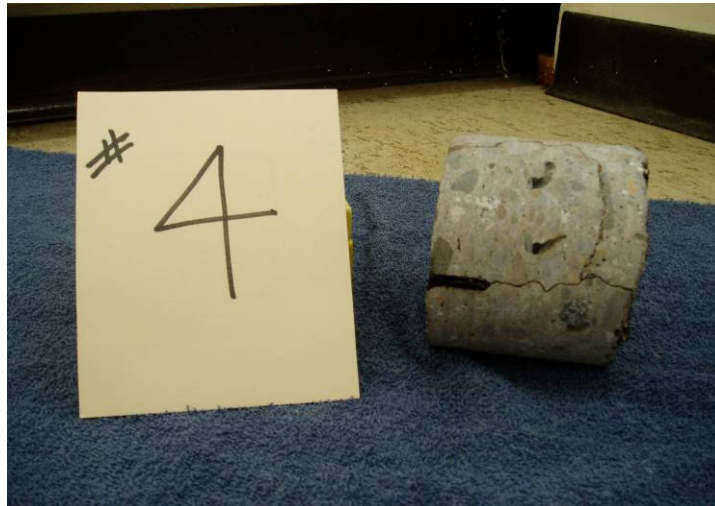
Figure 7. Side view showing panel joint and horizontal cracks. August 2004.
