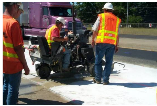
Image B. Joint sawing operation.
