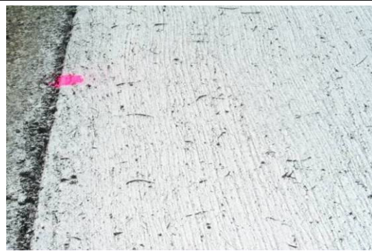
Image D. Surface of whitetopping showing fiber reinforcement.
