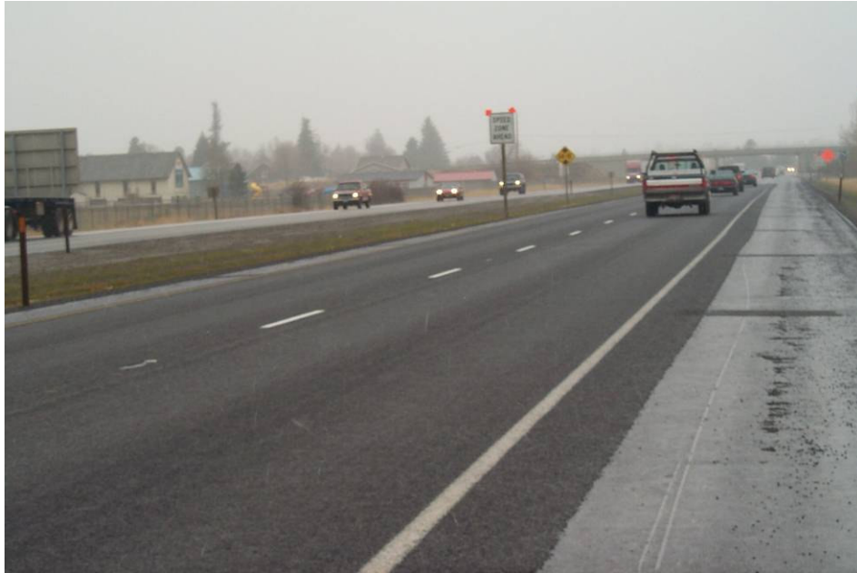
Image 4. Macro Surfacing Test Section placed on top of the Micro-Surfacing rut fill placed in the westbound lanes of I-90 (MP 293.15 to MP 293.55).
