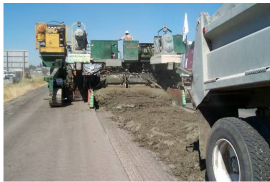
Image C. Truck delivering the wet concrete to the paver.
