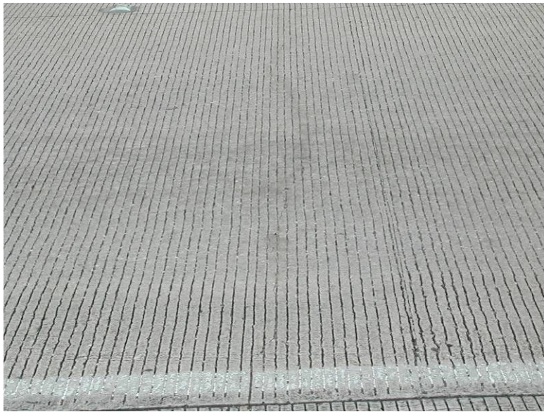
Figure 2. Concrete pavement on Interstate 45 in Houston, Texas after thirteen years of traffic.
