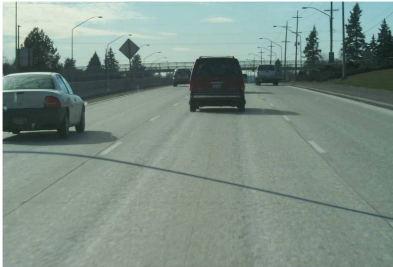
Figure 3. Wear due to studded tires on a PCC pavement (I-90 vicinity of Spokane).
