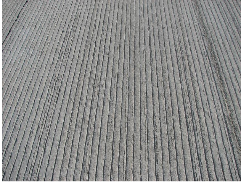
Figure 6. Close-up view of the pavement with longitudinal tining. May 2006.
