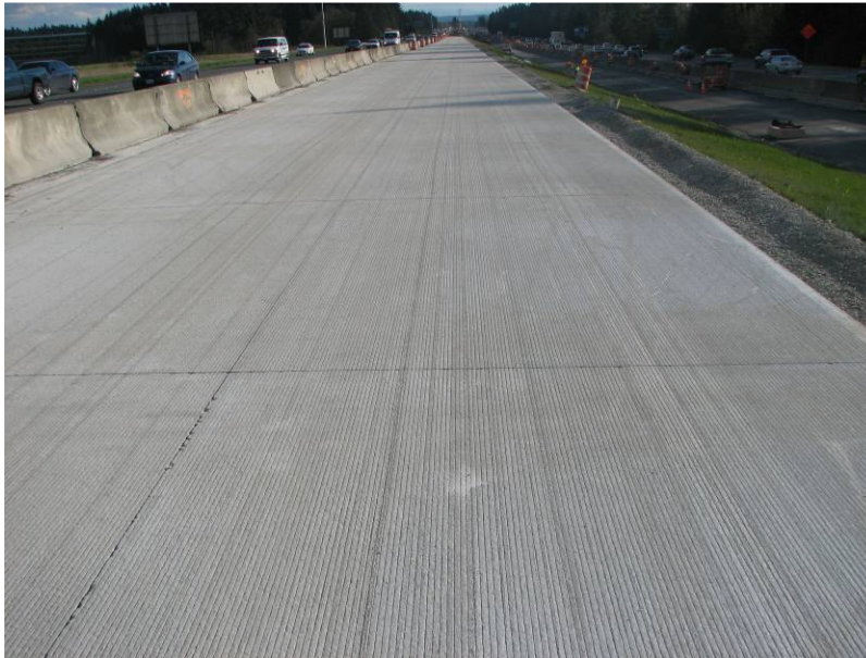
Figure 7. Longitudinal tining in the northbound HOV lane. May 2006.
