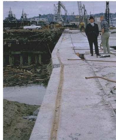
**Figure 1.3** Examples of liquefaction-related damage from the 1965 Seattle-Tacoma earthquake.
