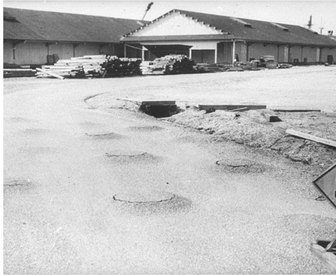
**Figure 1.2** Examples of liquefaction-related damage from the 1949 Olympia earthquake.
