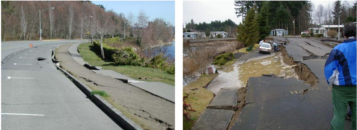
**Figure 1.4** Examples of liquefaction-related damage from the 2001 Nisqually earthquake.
