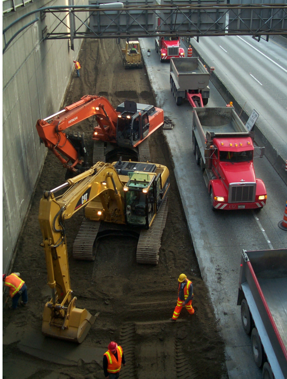
Figure 17 - Excavators working adjacent to structural walls (Photo courtesy of WSDOT).
