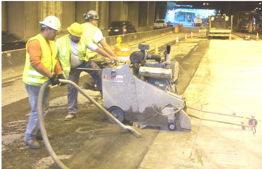
Figure 16 – Saw cutting PCC slab joints (Photo courtesy of WSDOT).
