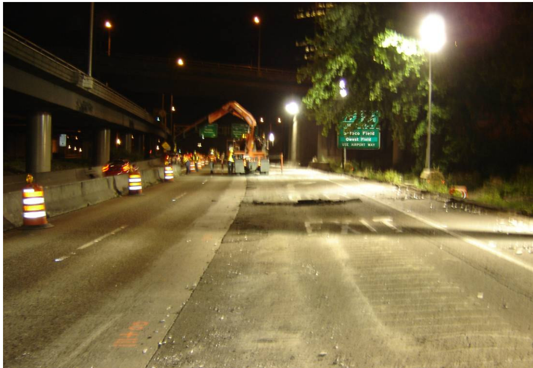
Figure 22 - Excavation crews working at night (Photo Courtesy of WSDOT).
