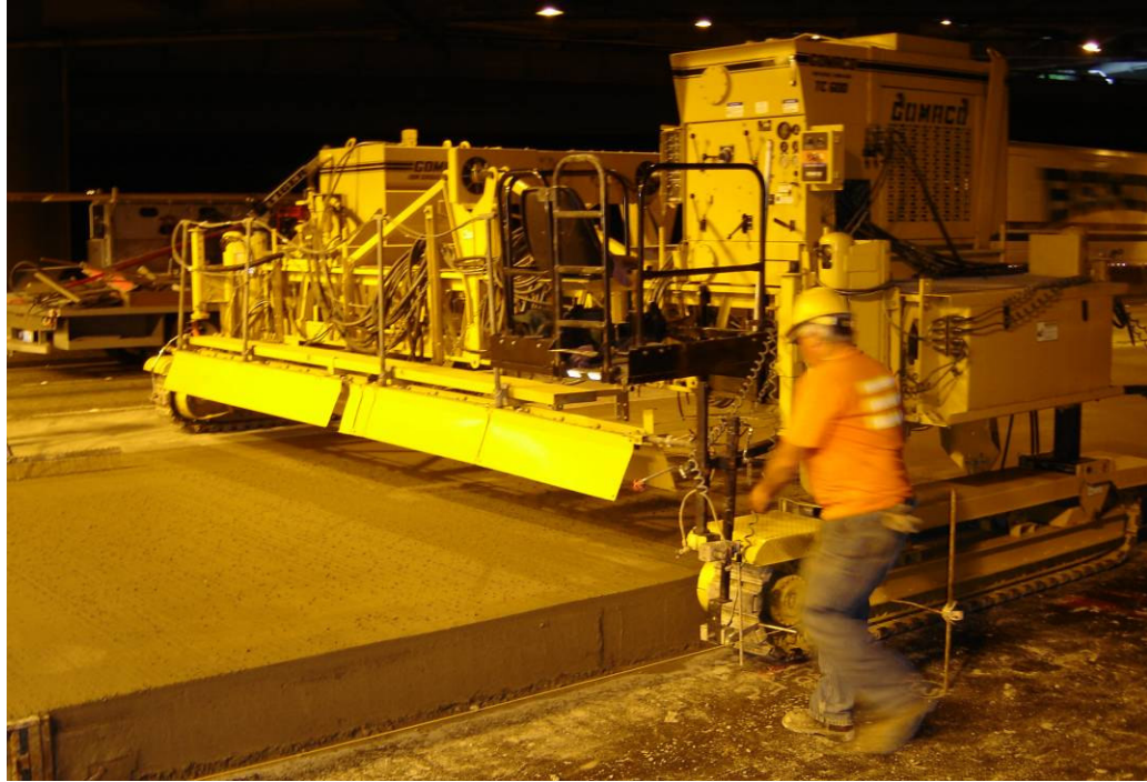
Figure 15 - Slipform PCC paving operation (Photo courtesy of WSDOT).
