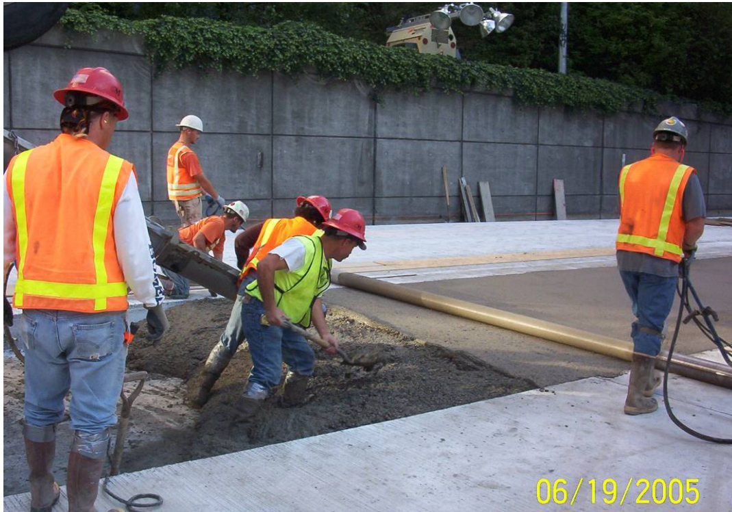
Figure 14 - Hand PCC paving with a bunion screed (Photo courtesy of WSDOT).
