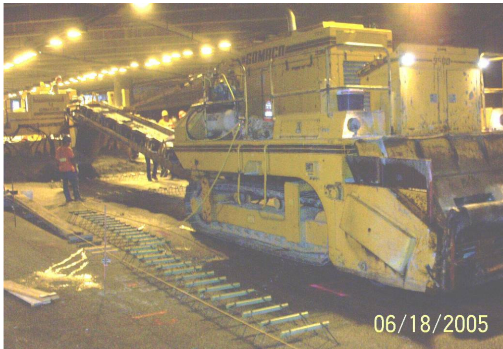
Figure 20 - PCC material transfer vehicle (Photo courtesy of WSDOT).
