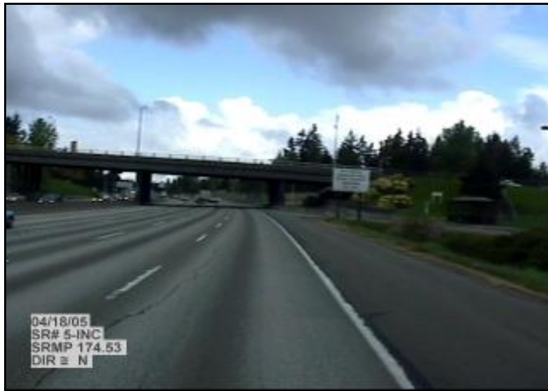
Figure 5. Photo Log from WSDOT of Pavement around Northgate Vicinity
