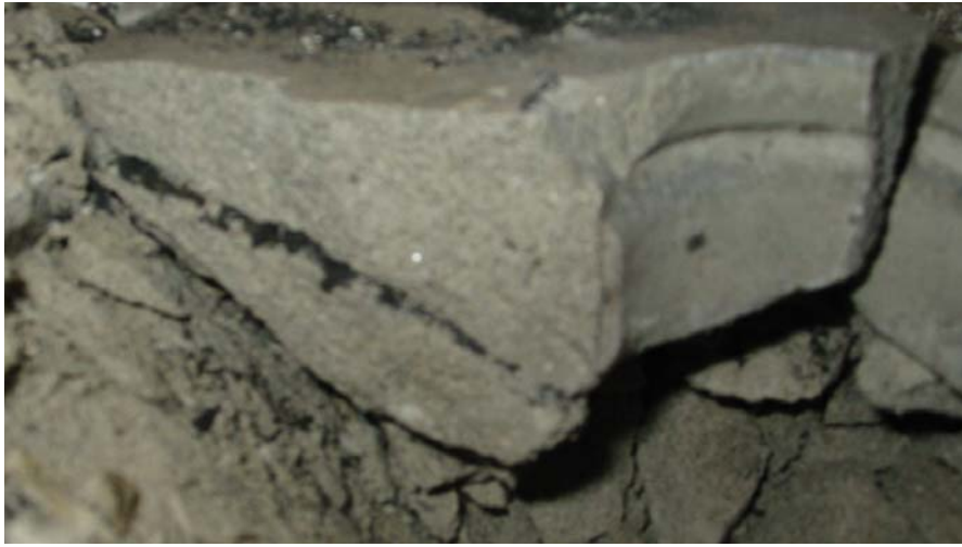
Figure 4.9: Layered grout cone: 14N08
