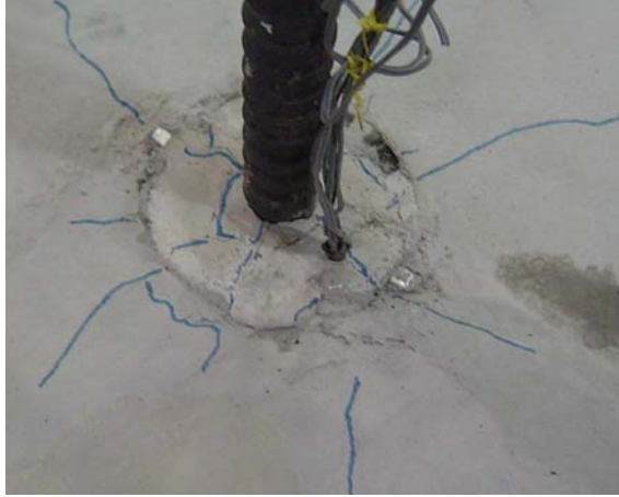
Figure D-10: Surface damage to Specimen AD8-FB
