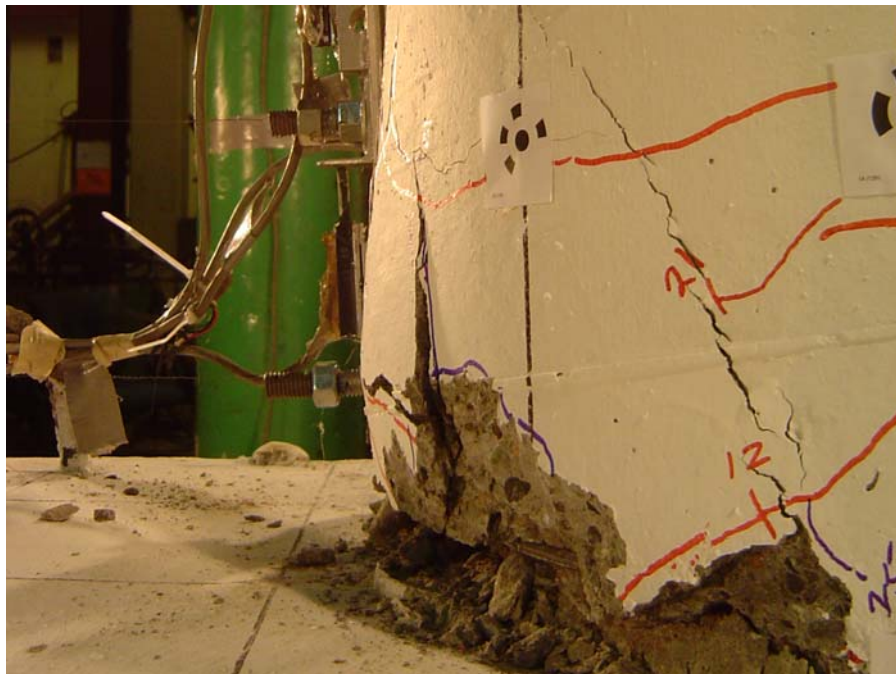
Figure 4-52: A bulge in the concrete cover indicates possible bar buckling in Specimen LB8-D2 during Cycle 30 (4.73%/-4.66%)
