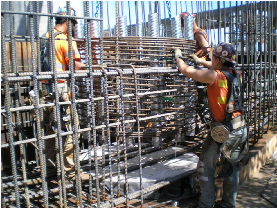
Figure 2-8: Template being tied with the reinforcement (WSDOT 2007)
