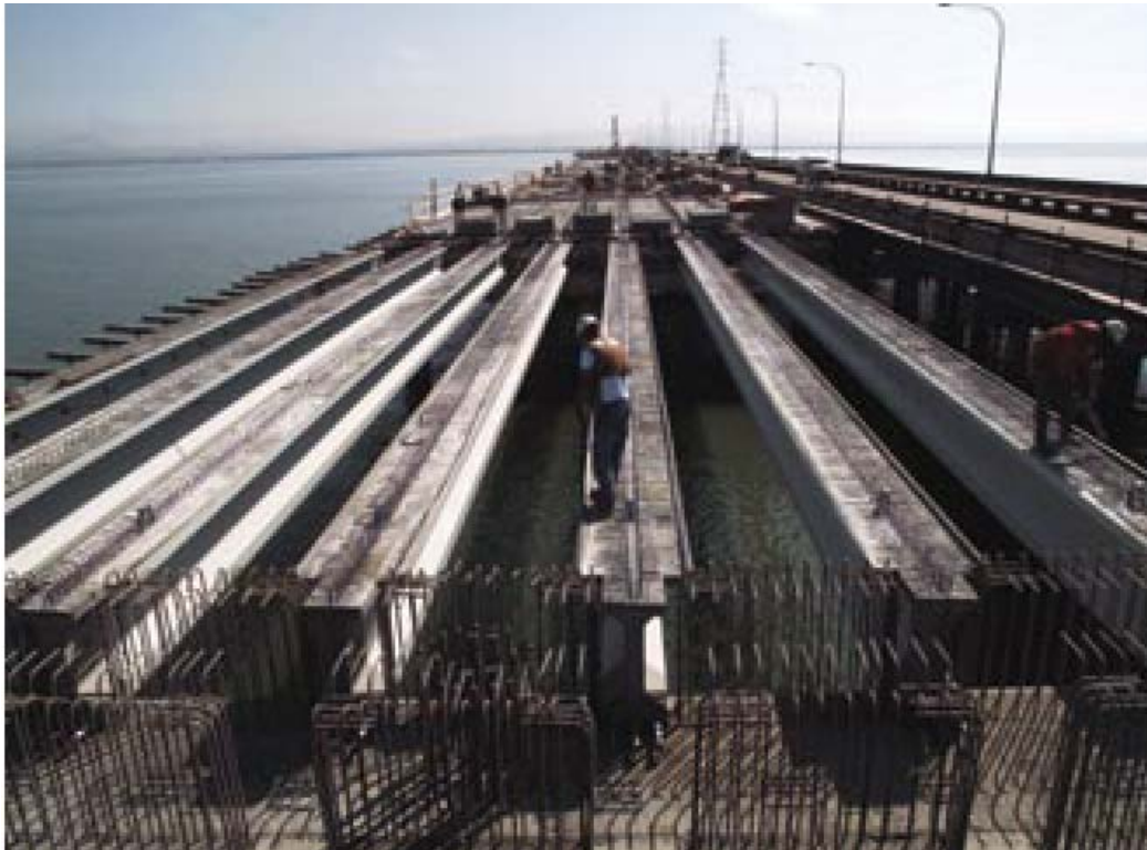
Figure 2-5: Placement of precast girders (Asnaashari et al. 2005)
