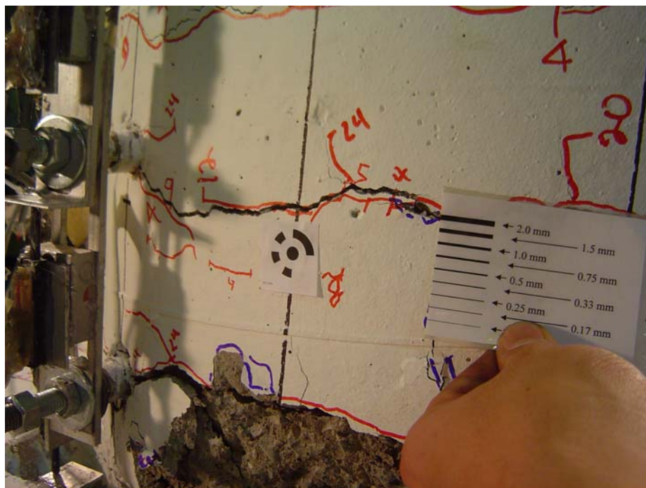
Figure 4-6: Crack localization in Specimen DB5-RE at Cycle 25 (2.96%/-3.02%)
