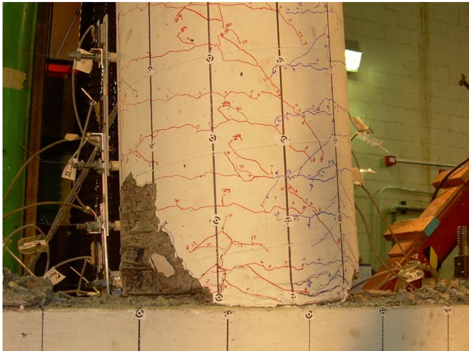
Figure 4-38: Fully spalled (10 inches) on the north face in Specimen LB8-D1 at Cycle 33 (7.11%/-6.93%)
