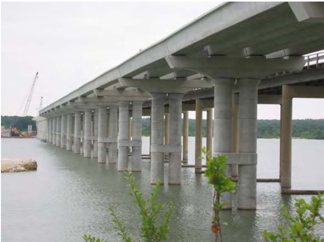
Figure 2-3: Construction of Lake Belton Bridge (Brenes 2006)
