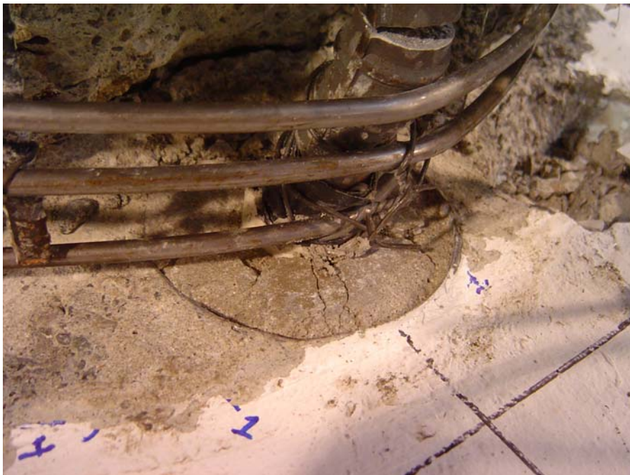
Figure 4-58: Specimen LB8-D2 with no spalling in the cap-beam; radial cracks in the grout at the end of testing
