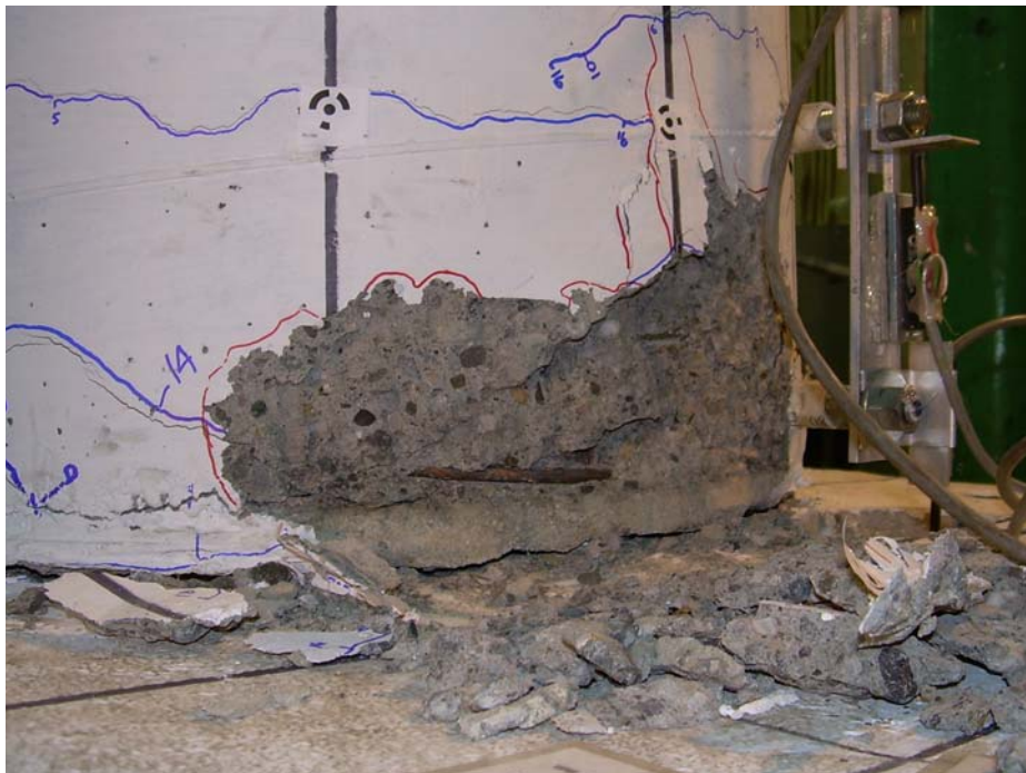
Figure 4-34: Reinforcement exposed in Specimen LB8-D1 Cycle 25 (3.03%/-3.06%)
