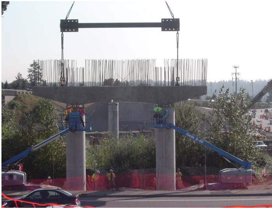
Figure 2-10: Erection of the precast bent-cap
