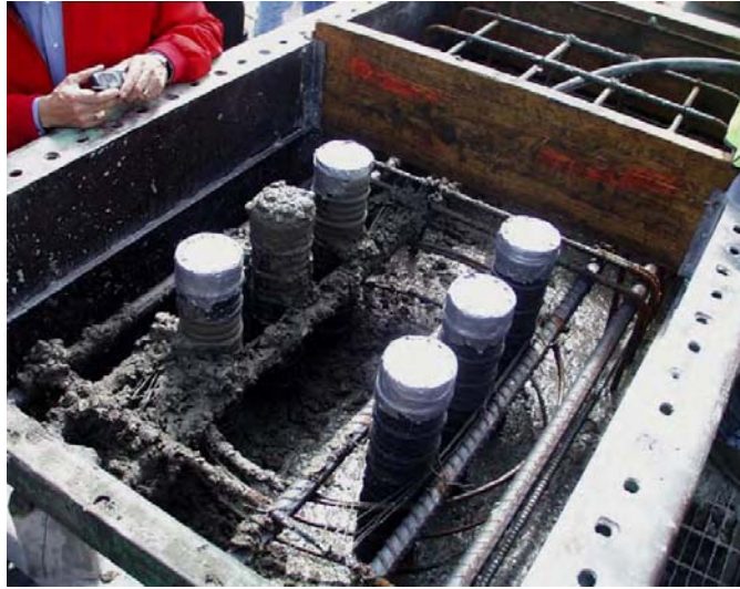
Figure 2-1: Corrugated ducts and joint reinforcement (Brenes 2006)
