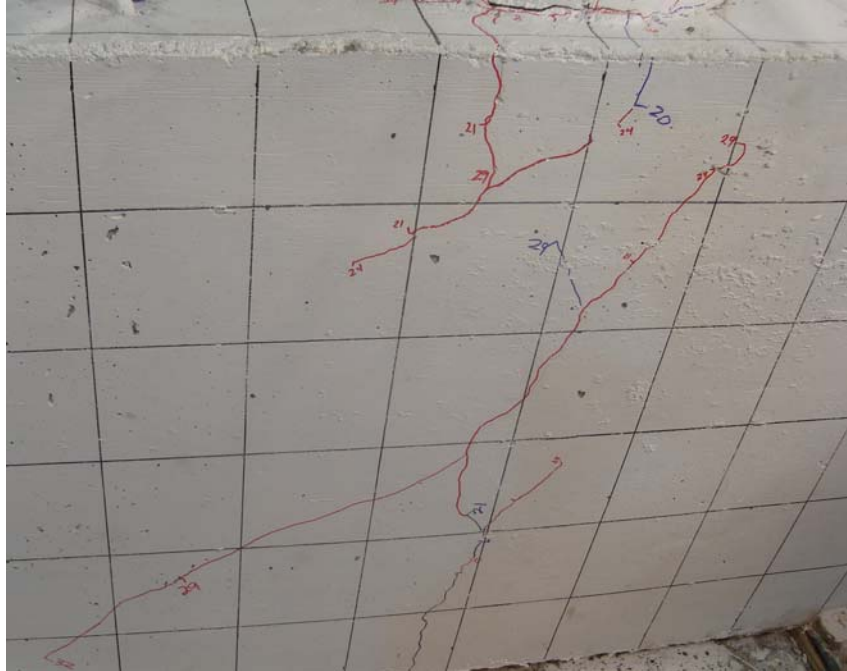
Figure 4-13: Damage to the west face of the cap-beam and diaphragm in Specimen DB5-RE at the end of testing
