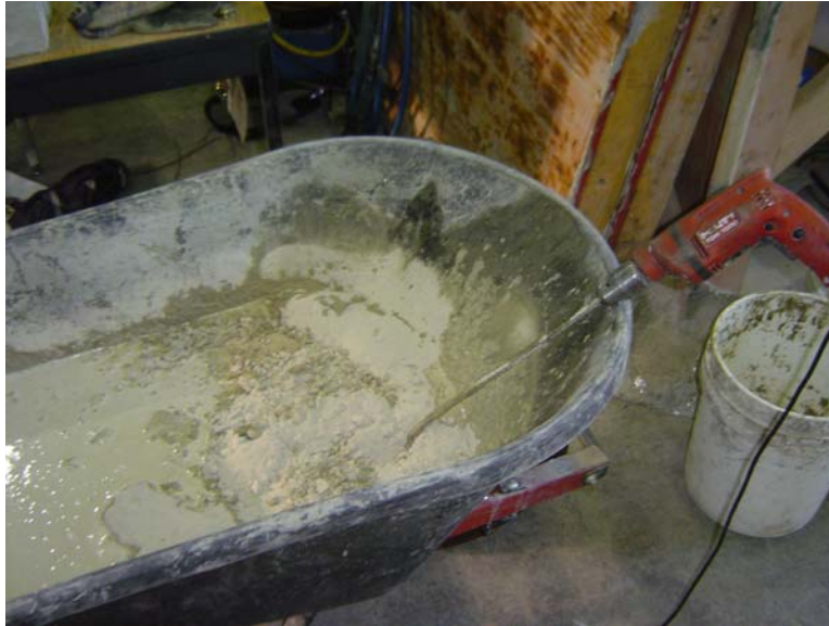
Figure B-14: Batching of grout mix
