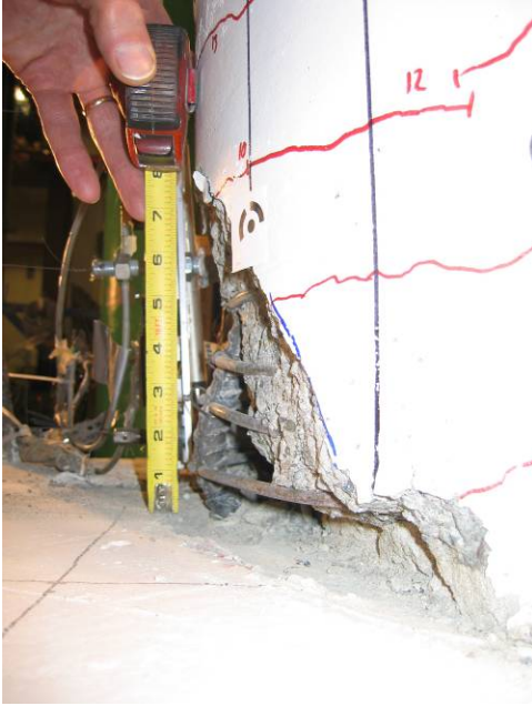
Figure 4-15. LB6-PT: Bar V00 buckled and spiral fractured, Cycle 32 (-5.38%).
