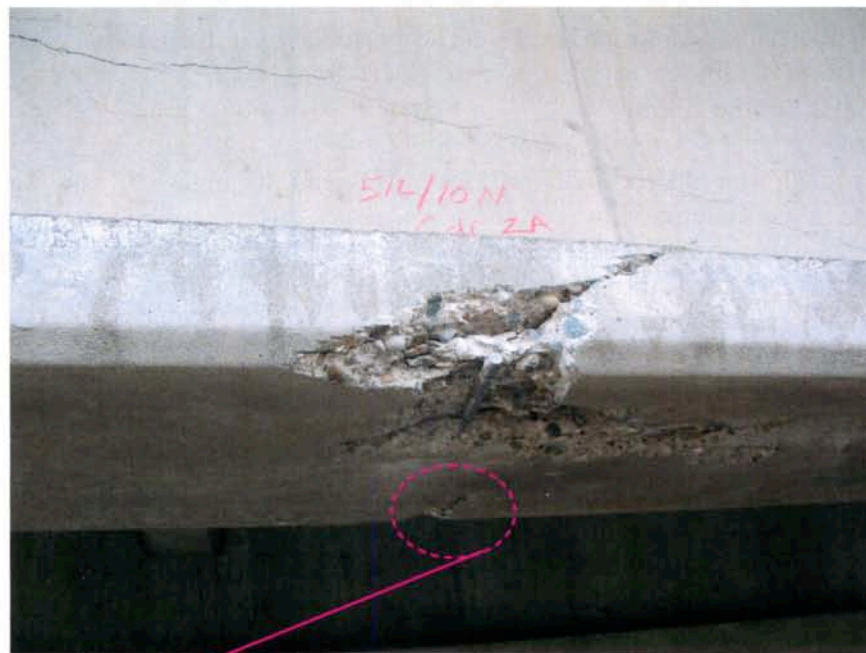
(c) Comparison with the real scenario (as shown in the photo, the impact loading position is a little bit away from the intermediate diaphragm, and a small area of the tensile failure developed on the back face of the girder flange, the same as showed in the simulation plots of (a) and (b))
