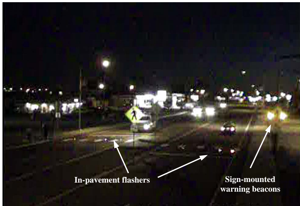
Figure 3.6. Warning lights lit for pedestrian crossing— after condition—Airway Heights
