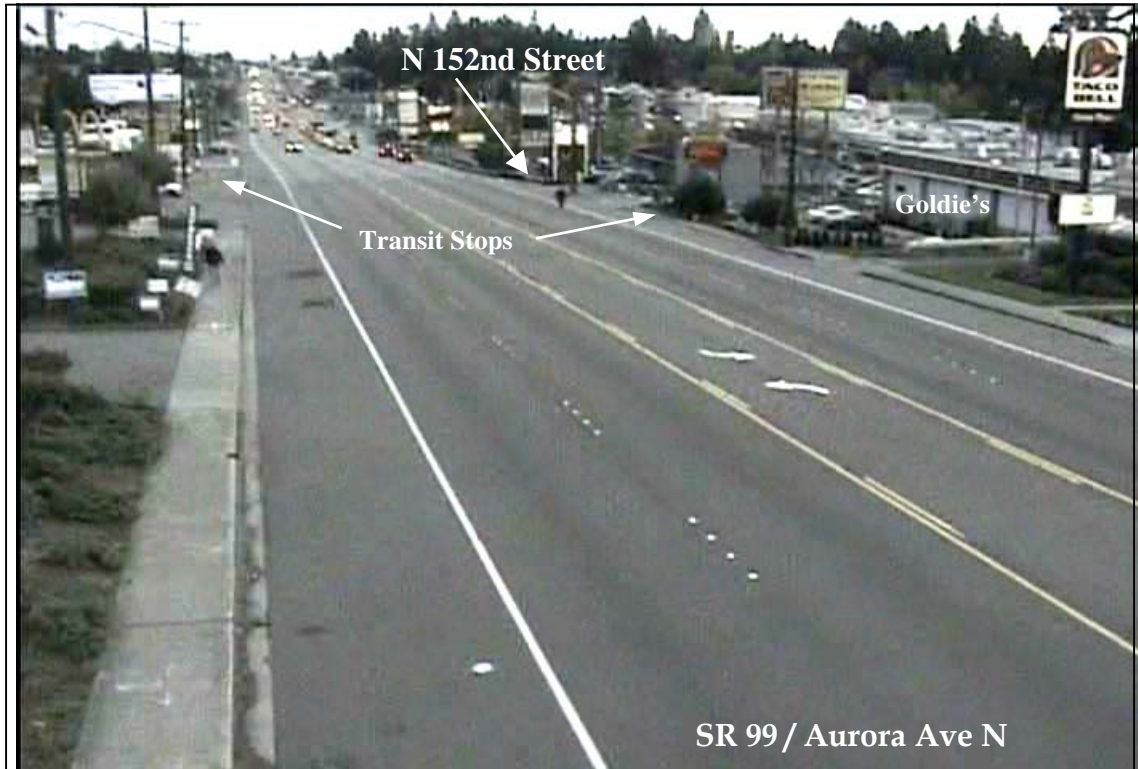
Figure 2.6. Observation boundaries, SR 99 south of N 152 nd Street—before improvements—Shoreline
