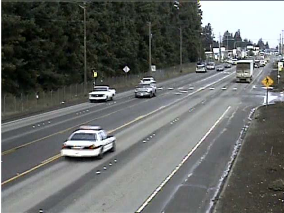
Figure 2.1. Observation boundaries north of S. 180 th Street— before phase—Spanaway (Kopf and Hallenbeck 2005)
