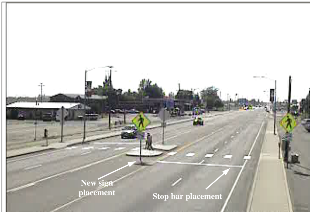
Figure 3.10. Median sign and stop bar placement— after condition—Airway Heights
