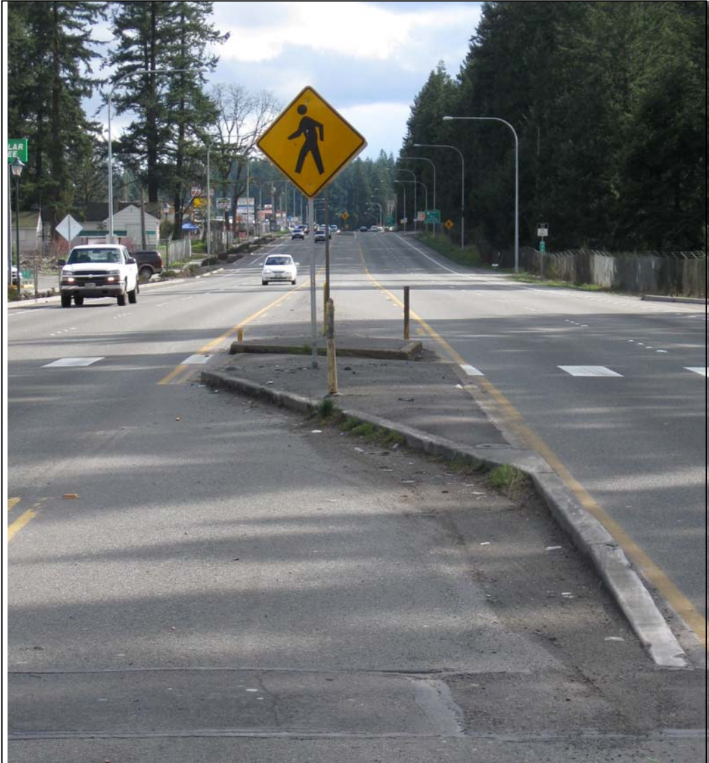
Figure 3.3. Front view of median with crosswalk markings—Spanaway
