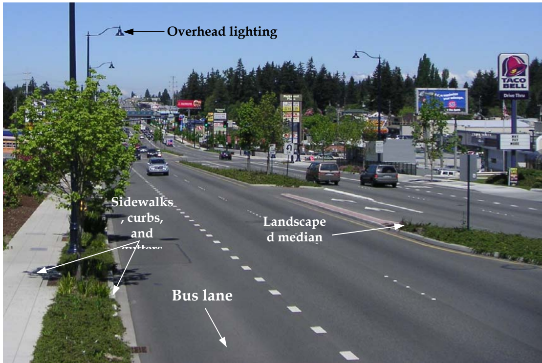
Figure 2.8. View of the improvements made to the project and surrounding area, SR 99 and N 152nd Street—Shoreline
