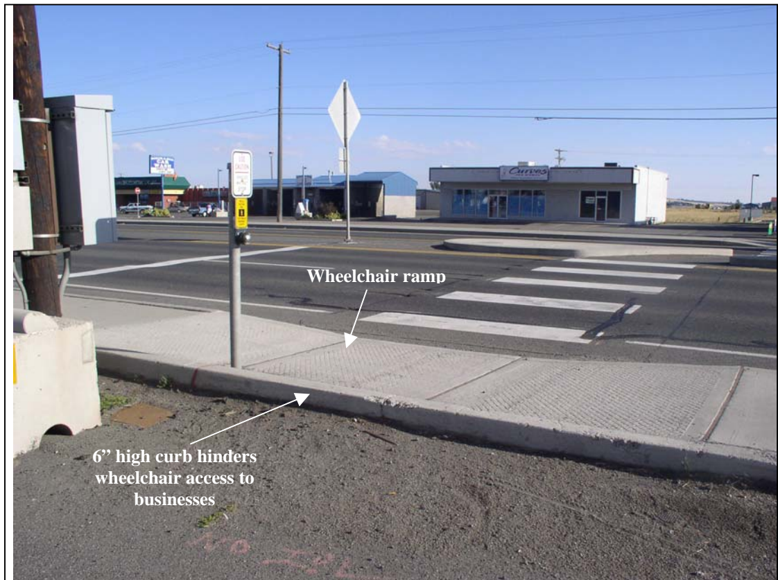
Figure 4.1. Wheelchair ramp on SR 2 between King and Lundstrom Streets
