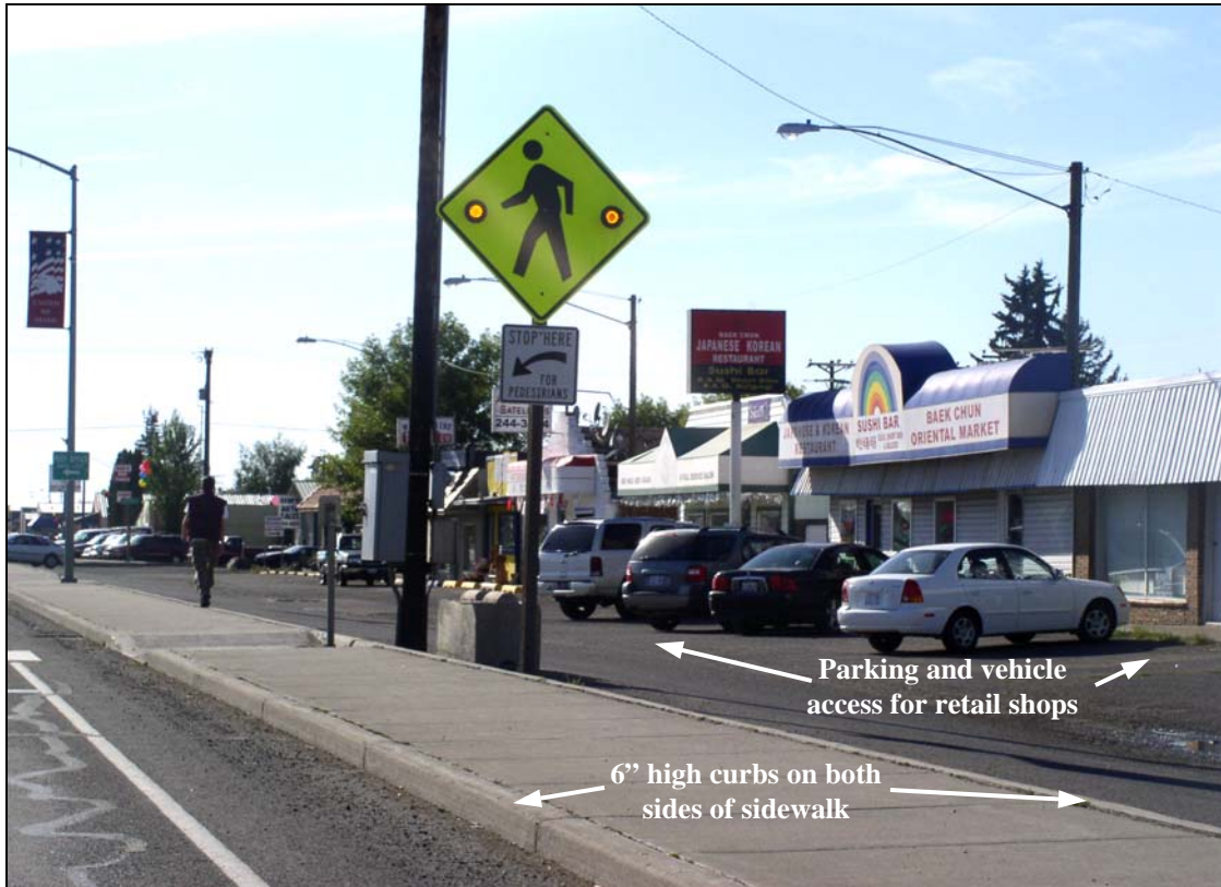
Figure 2.12. SR 2 sidewalk and parking detail (looking west)—Airway Heights
