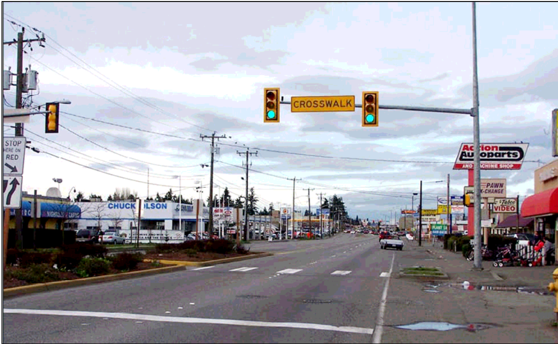
Figure 1.1. Typical streetscape of an arterial near Seattle, Washington (Jones & Stokes 2007)
