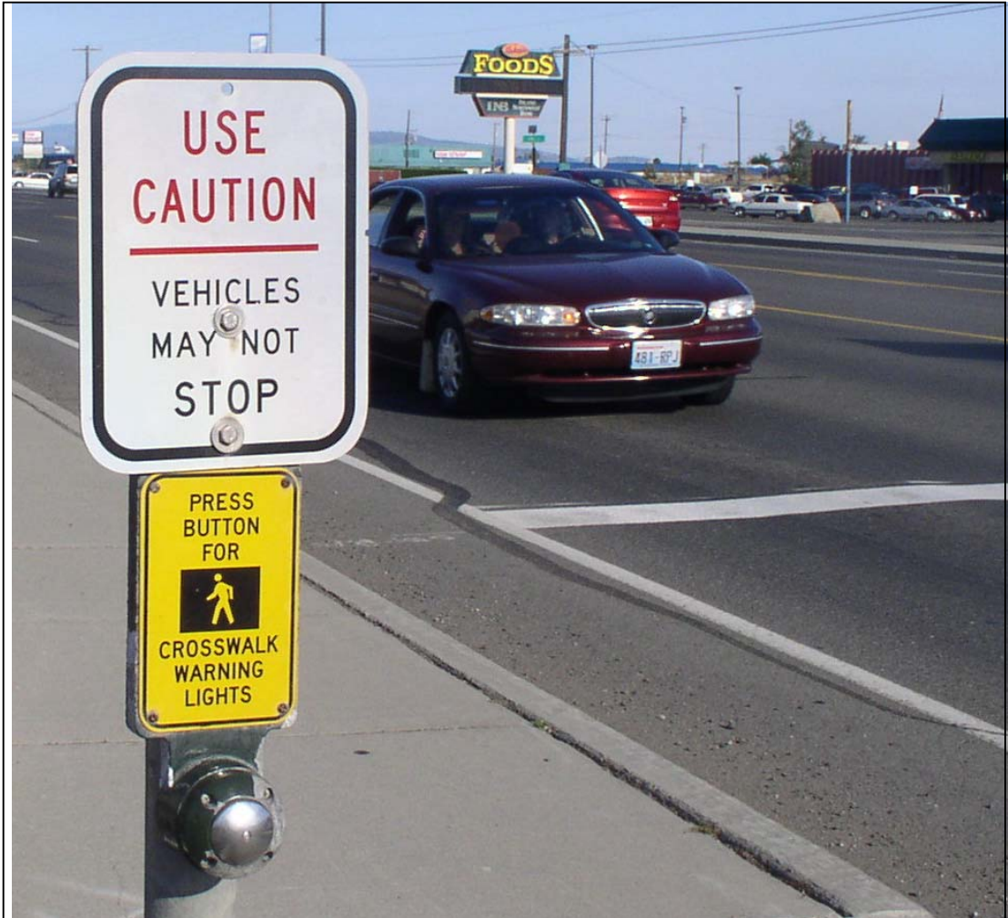
Figure 3.11. Signs present at the pedestrian actuation button—Airway Heights
