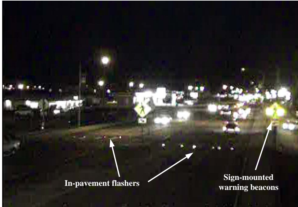
Figure 3.5. Warning lights lit for pedestrian crossing— before condition—Airway Heights
