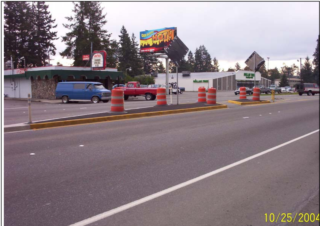
Figure 3.1. Pedestrian refuge islands at S. 180 th Street and SR 7—Spanaway (Kopf and Hallenbeck 2005)
