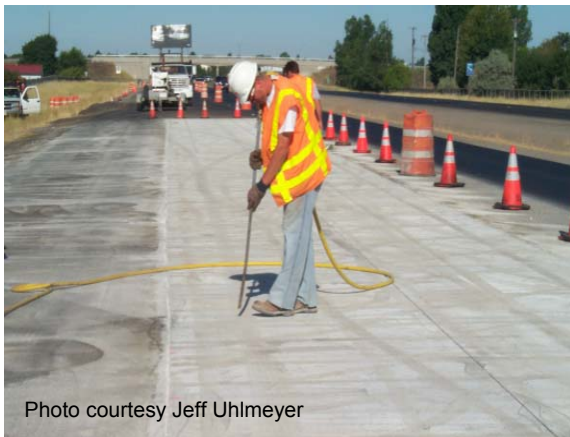
Figure 31 Cleaning joints.
