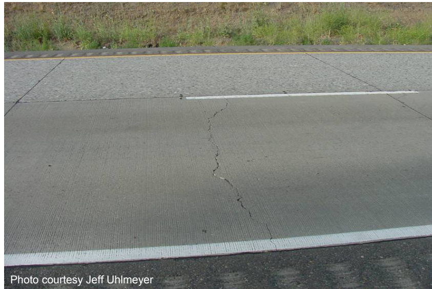
Figure 22 Transverse cracking.
