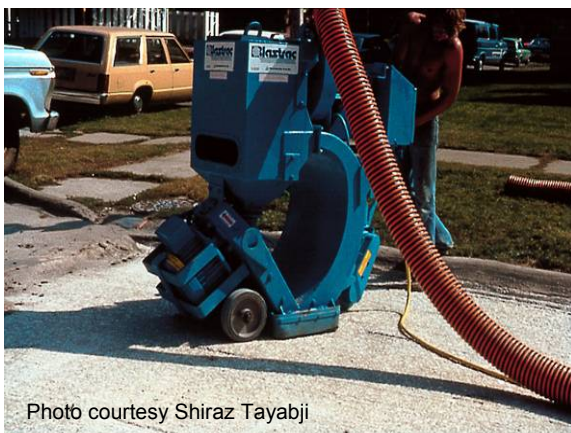
Figure 89 Shotblasting surface.
