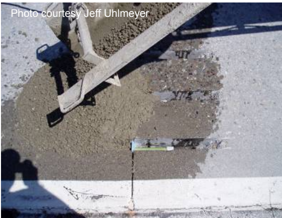
Figure 79 Placing patching material.
