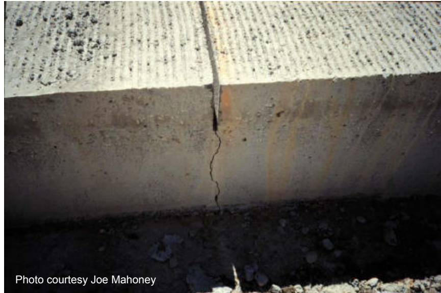
Figure 10 Aggregate interlock.
