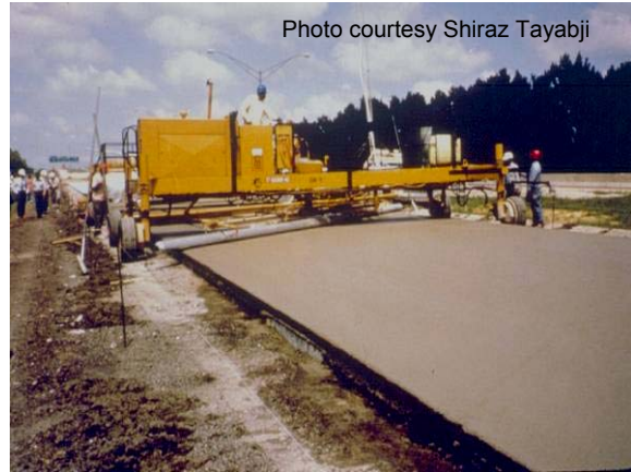
Figure 92 Placing bonded concrete overlay.
