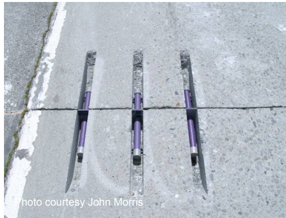
Figure 78 Dowel bar retrofit assembly in dowel bar slot.
