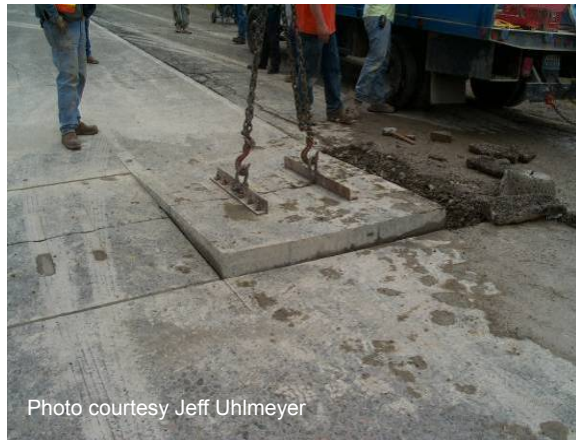
Figure 52 Concrete removal (lifting method).
