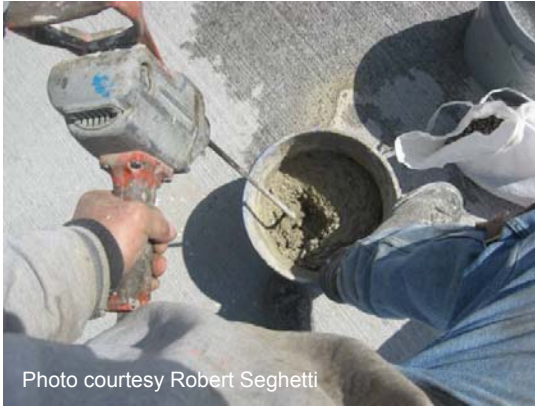
Figure 45 Mixing patching material.
