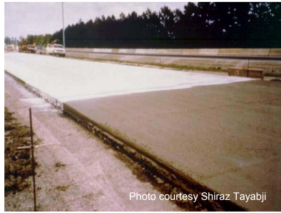
Figure 94 Curing bonded concrete overlay.
