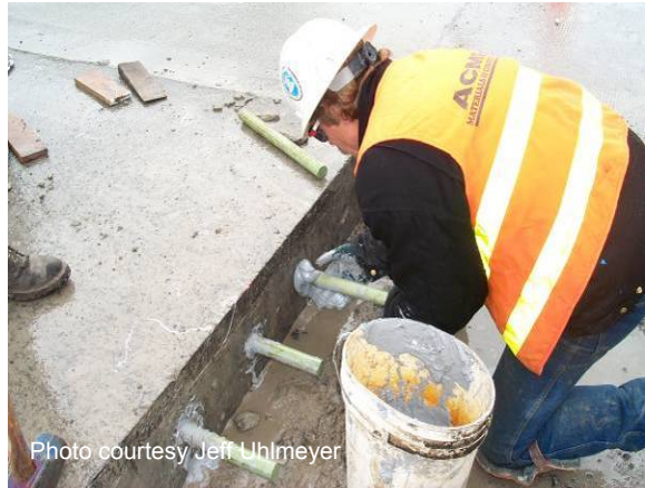
Figure 58 Inserting dowel bar.
