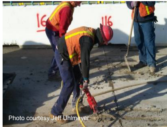
Figure 72 Removing concrete from dowel bar slot.
