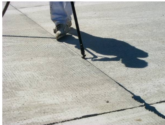
Figure 32 Sealing joints or cracks.
