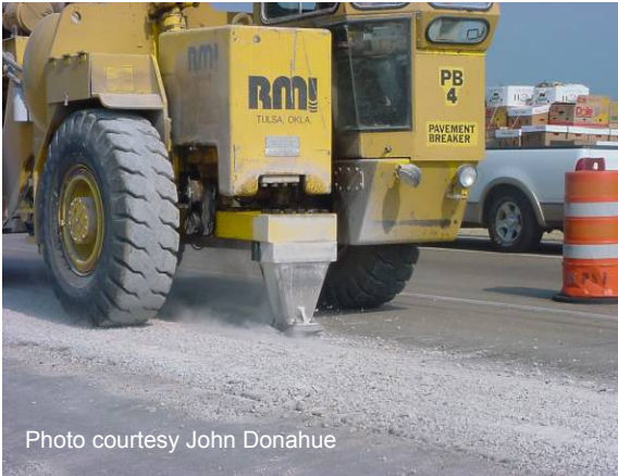
Figure 101 Resonant breaker.
