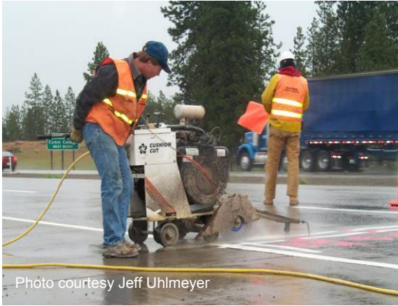
Figure 49 Sawcutting.
