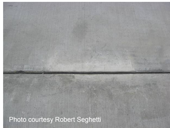
Figure 48 Final spall repair.
