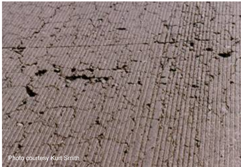
Figure 16 Alkali-Silica Reactivity.
