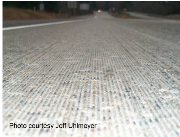
Figure 67 Diamond grinding surface.
