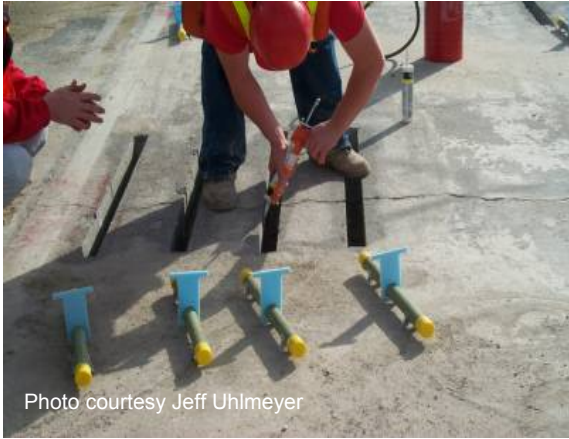
Figure 75 Applying silicone sealant.
