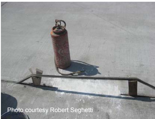
Figure 47 Applied curing compound.
