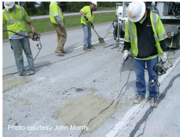
Figure 80 Consolidating patching material.
