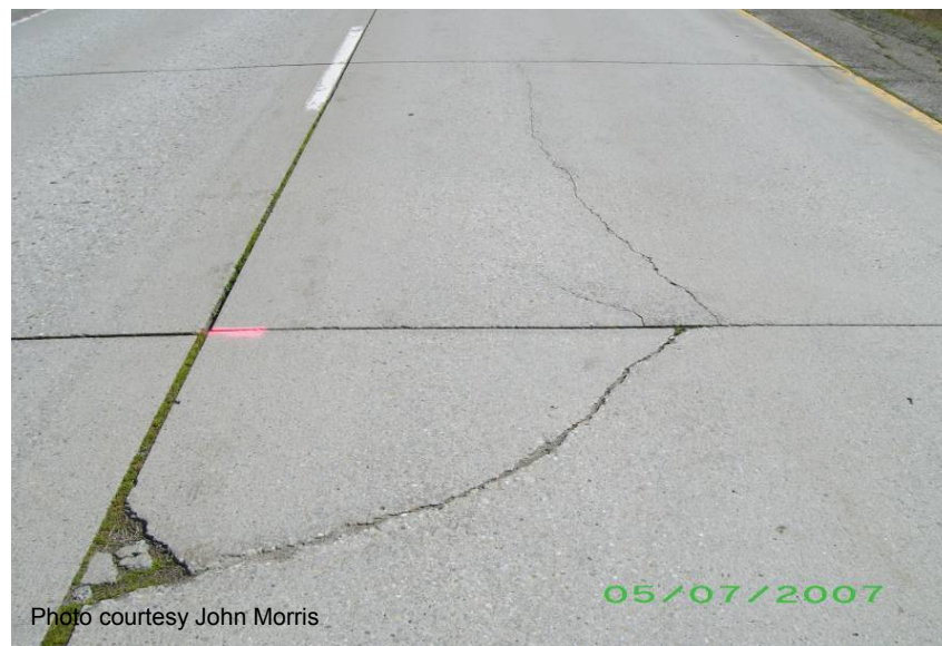
Figure 21 Corner cracking.
