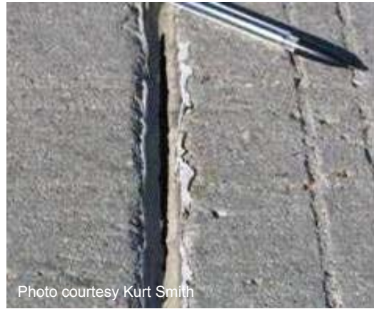
(b) Cohesive failure.
