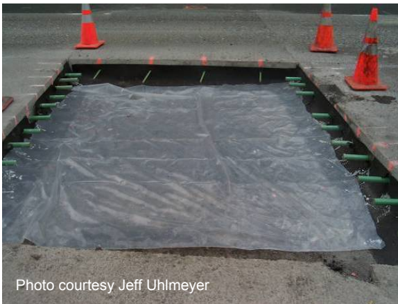
Figure 59 Plastic sheeting to debond concrete from base.
