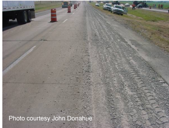
Figure 102 Resonant breaker surface.
