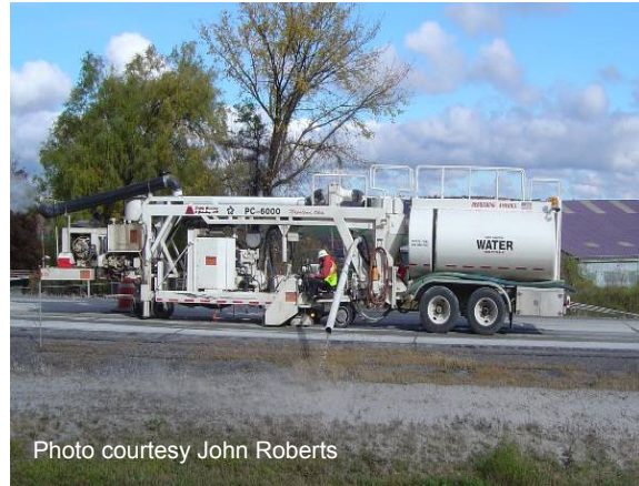
Figure 65 Diamond grinding machine.
