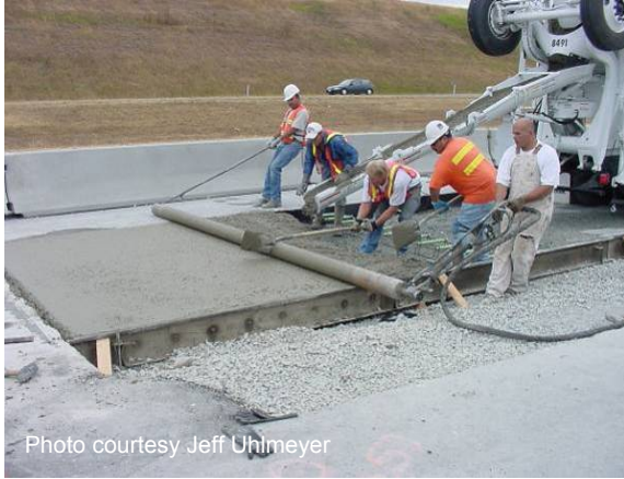
Figure 61 Final screed rolling.
