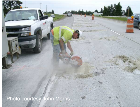
Figure 82 Resawing joint in dowel bar slots.
