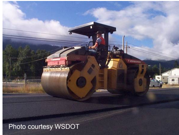
Figure 84 Compacting HMA.
