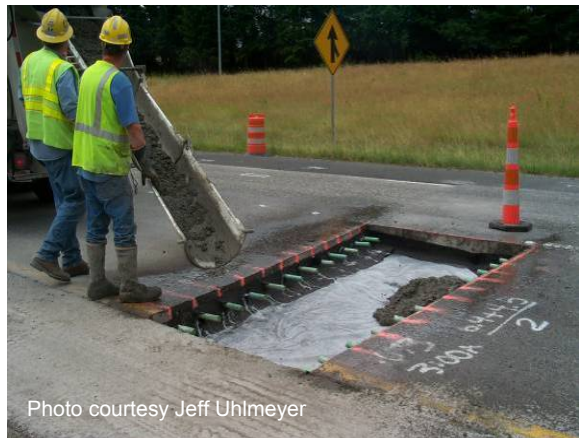
Figure 60 Placing concrete.
