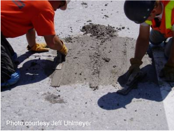
Figure 81 Finishing patching material.
