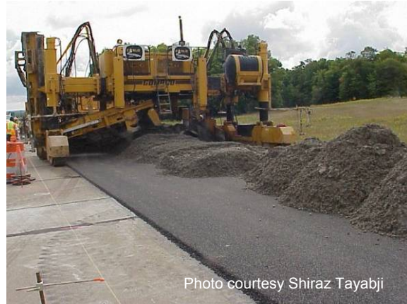
Figure 97 Placing concrete.
