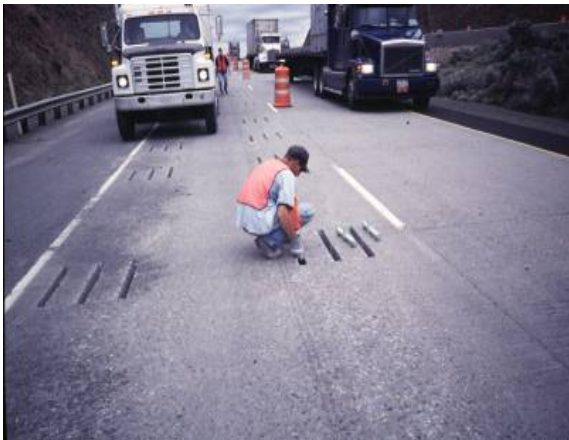
Figure 77 Inserting dowel bar retrofit assembly into dowel bar slot.
