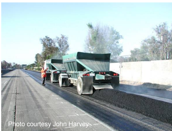
Figure 87 Delivery of HMA.
