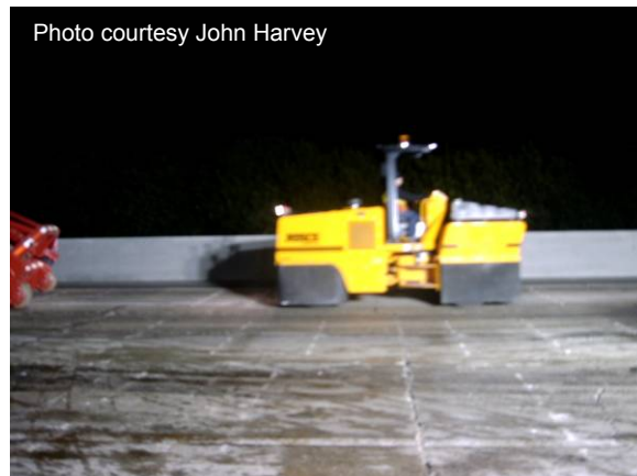
Figure 86 Seating concrete pavement.
