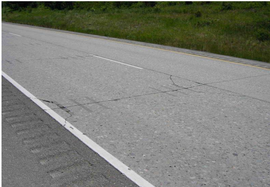
Figure 216 45-degree cracking.
