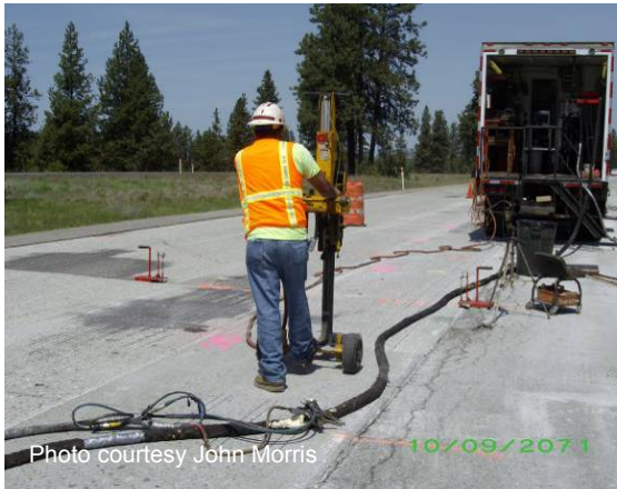
Figure 35 Drilling holes.
