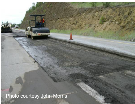
Figure 53 Compacting base.
