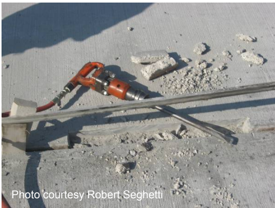
Figure 41 Removing concrete.
