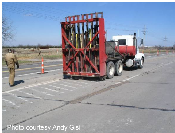
Figure 85 Drop hammer for cracking panels.
