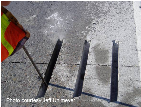
Figure 73 Cleaning dowel bar slots (close-up).
