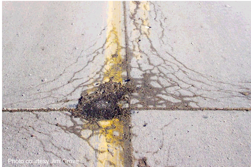
Figure 17 D-cracking.
