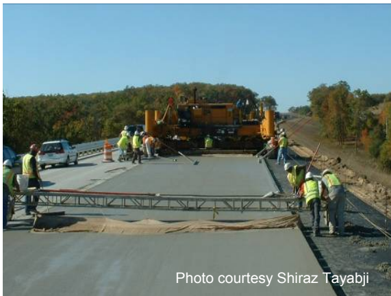
Figure 98 Finishing concrete.
