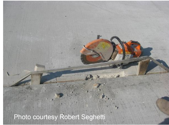
Figure 40 Sawcutting around spall.
