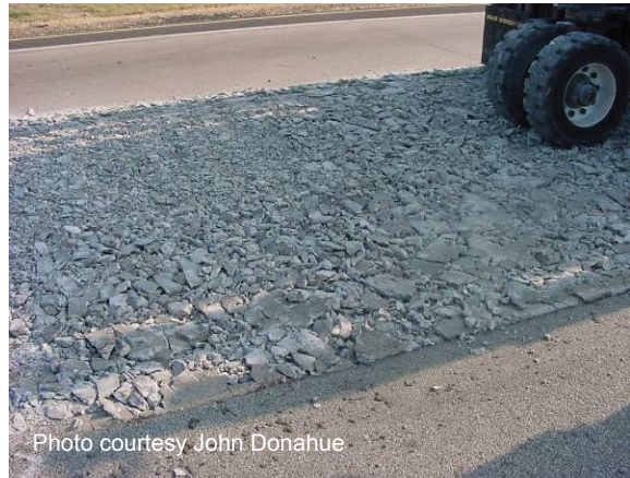
Figure 100 Multi-head breaker surface.
