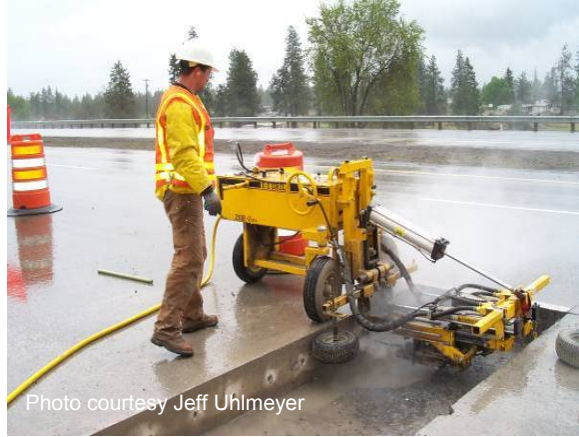
Figure 56 Drilling holes for dowel bars.
