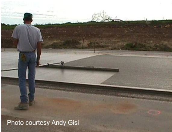
Figure 93 Tining bonded concrete overlay.
