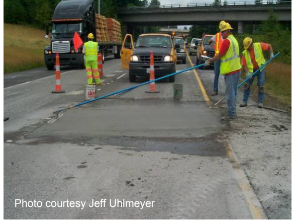
Figure 62 Finishing concrete.
