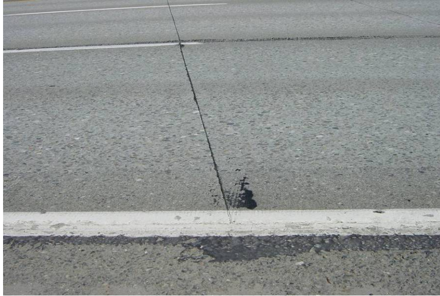
Figure 7 Contraction joint.
