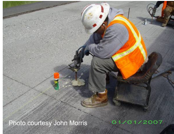
Figure 36 Pressure grouting.
