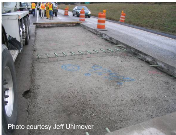
(a) Dowel bars in cages.
