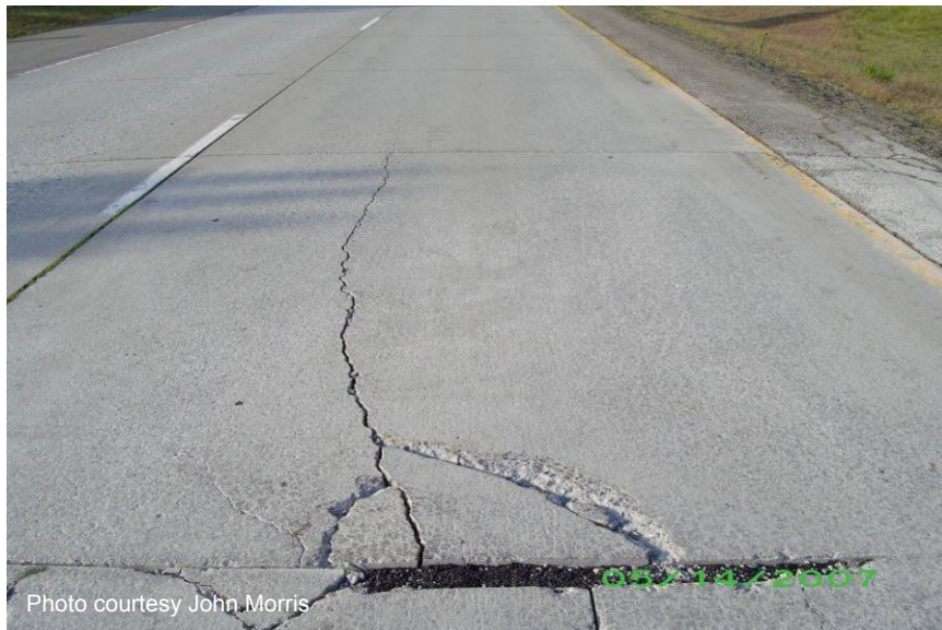
Figure 24 Multi-cracked panel.
