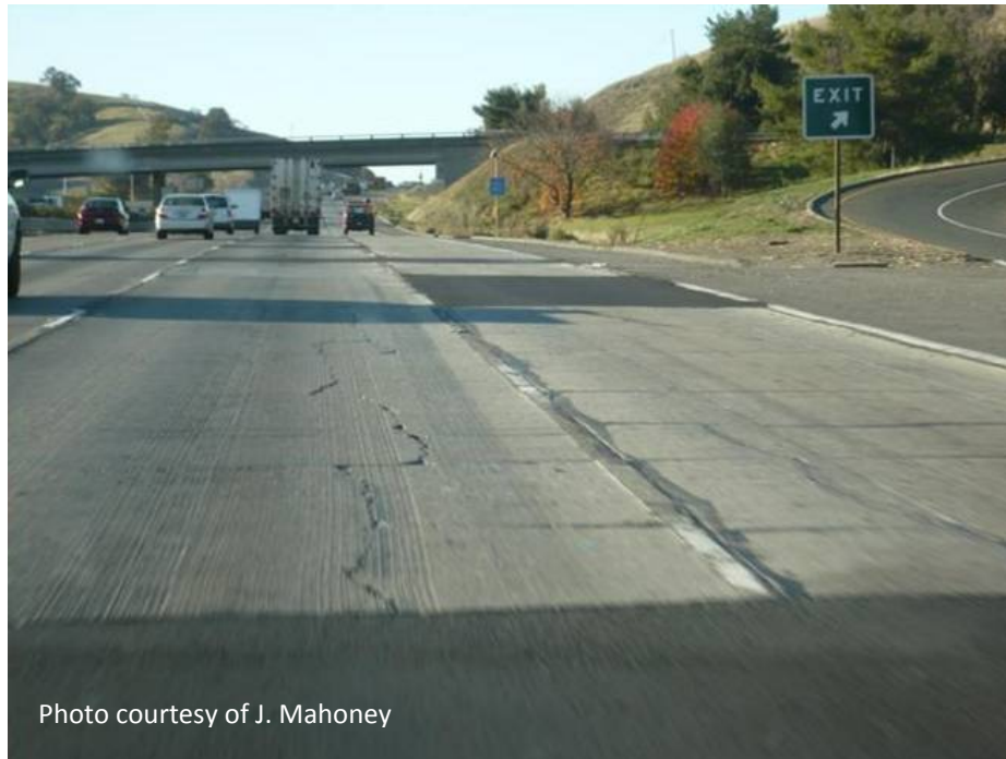
Figure 240 Severely deteriorated concrete pavement (I-80, California).
