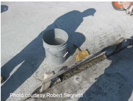
Figure 43 Applying bonding agent.
