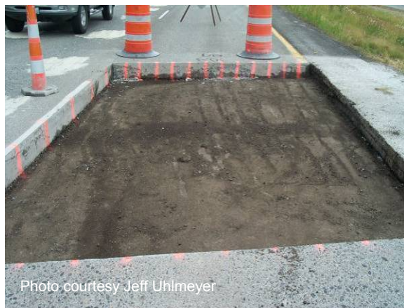
Figure 54 Prepared base.
