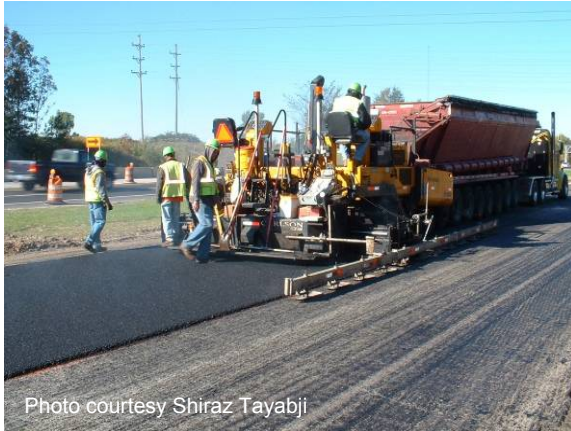
Figure 96 Placing HMA separator layer.
