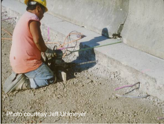
Figure 55 Drilling holes for tie bars.
