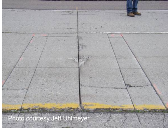
Figure 50 Relief saw cuts.
