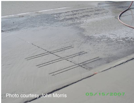
Figure 71 Cut dowel bar slots.
