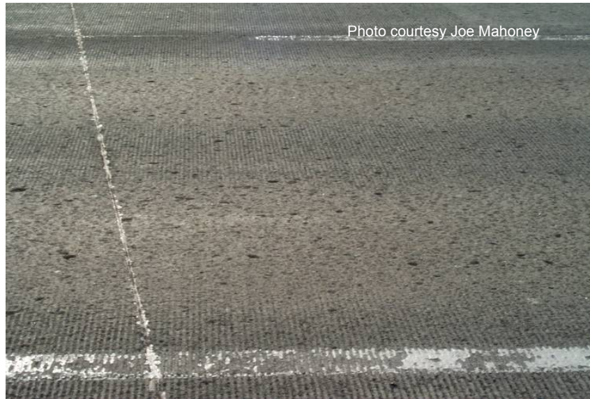
Figure 14 Moderate studded tire wear (SR 395 - no tining in wheelpaths).
