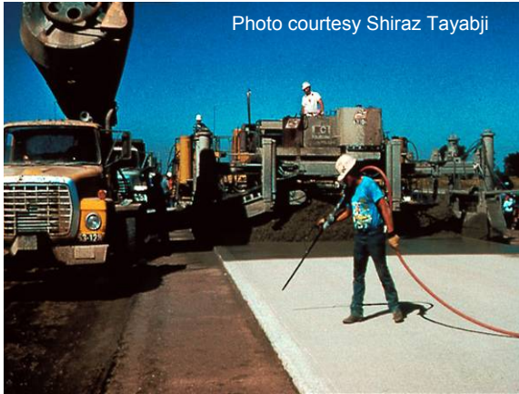
Figure 91 Final cleaning prior to paver.
