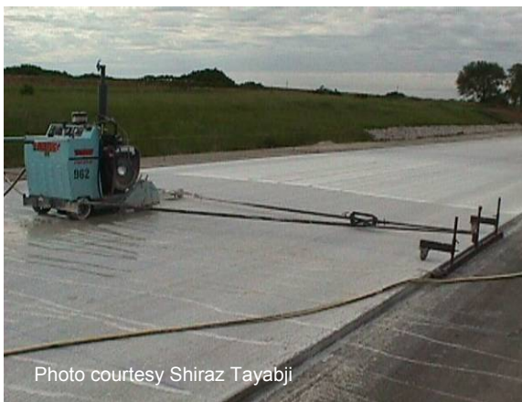
Figure 95 Joint sawing.
