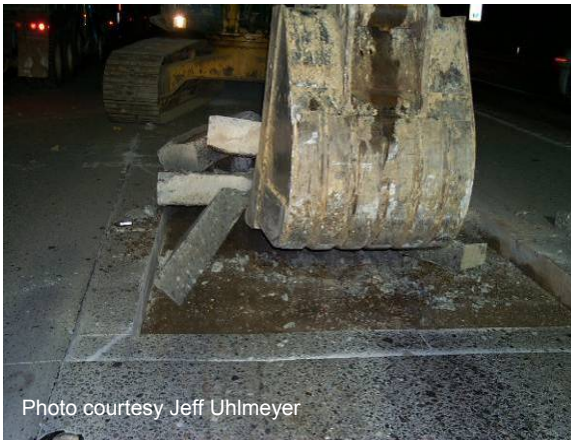
Figure 51 Concrete removal.
