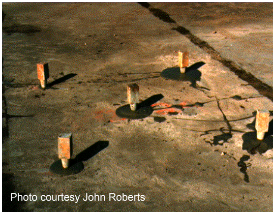
Figure 37 Plugging holes when pozzolan-cement is used.
