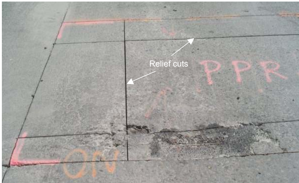
Figure 238 Relief cuts for panel replacements.
