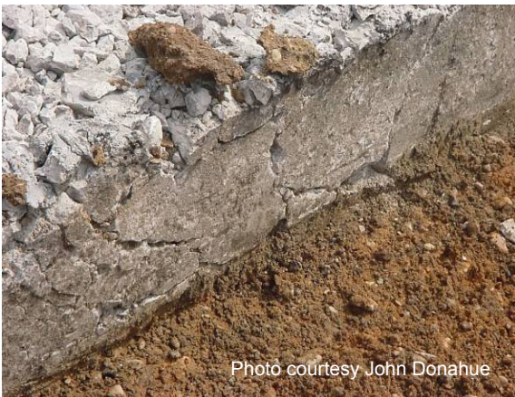
Figure 103 Rubblized concrete slab.
