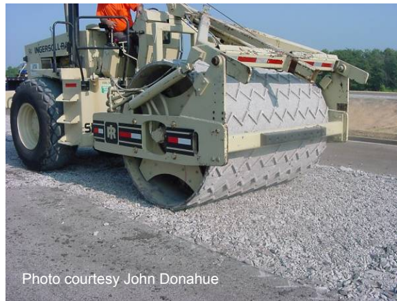
Figure 104 Rolling rubblized layer.
