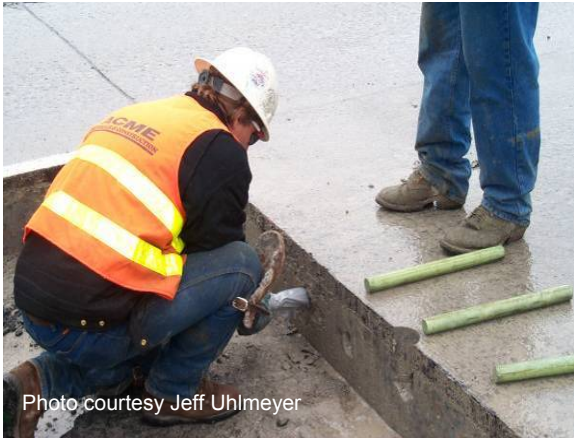
Figure 57 Inserting epoxy into dowel hole.
