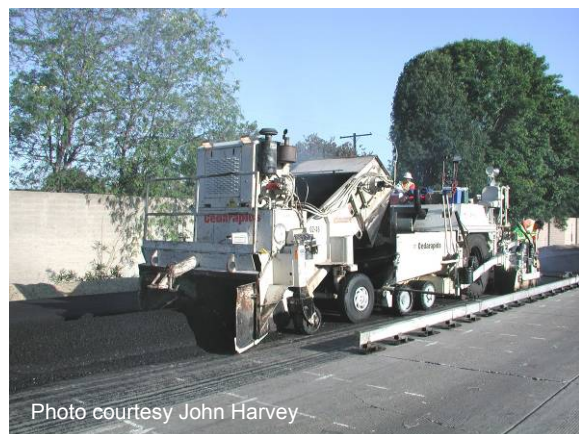
Figure 88 HMA pick up and paving.
