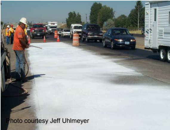
Figure 63 Applying curing compound.
