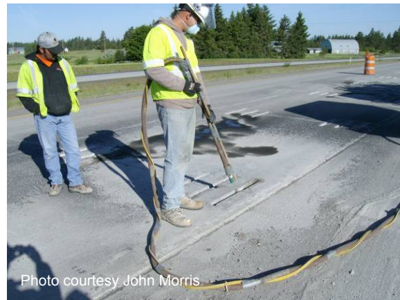
Figure 74 Cleaning dowel bar slots.
