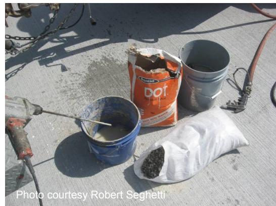
Figure 44 Materials for spall repair.
