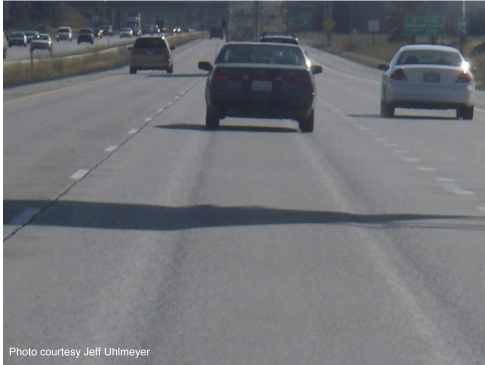
Figure 164 Studded tire wear on I-90, Spokane, Washington (2008).
