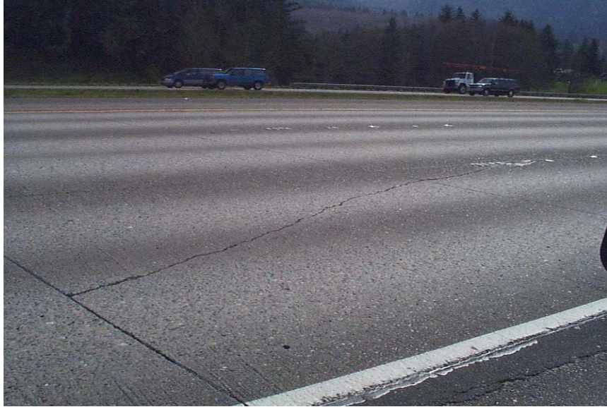
Figure 23 Longitudinal cracking.
