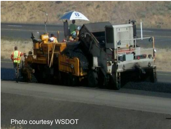
Figure 83 Placing HMA.
