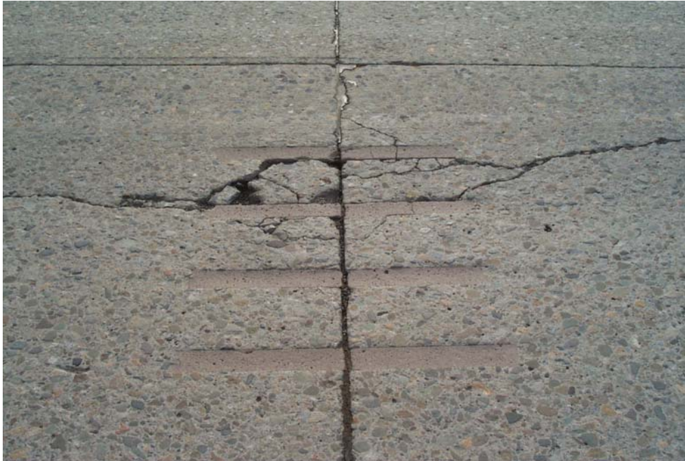
Figure A-21. Failure of dowel bar slot placed over existing longitudinal crack.
