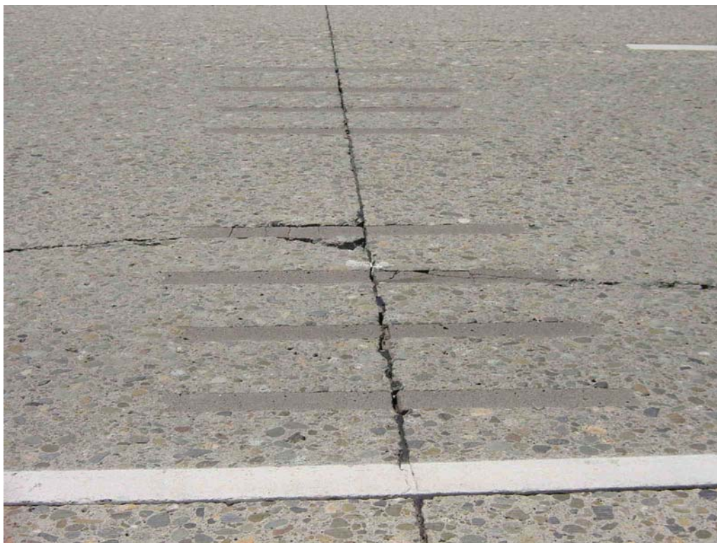
Figure A-20. Failure of dowel bar slot placed over existing longitudinal crack.
