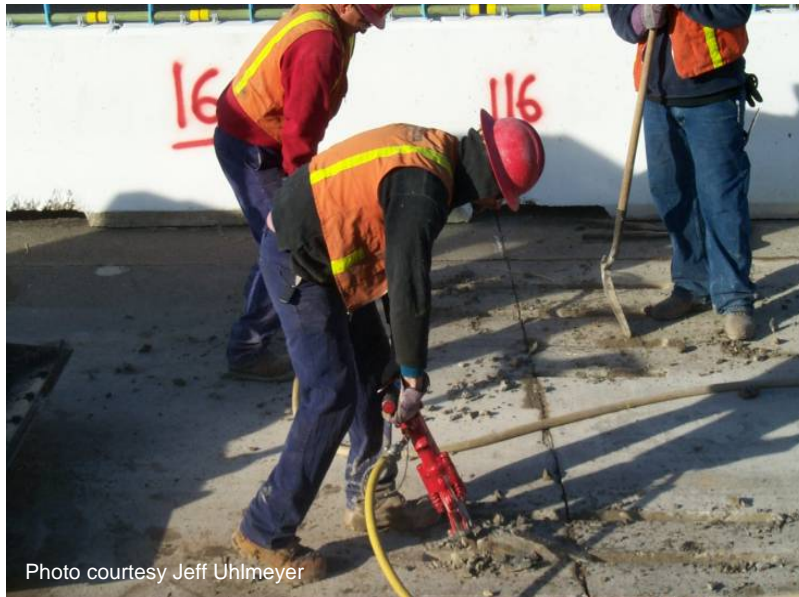
Figure A-23. Maintain jackhammer at no more than a 45-degree angle.
