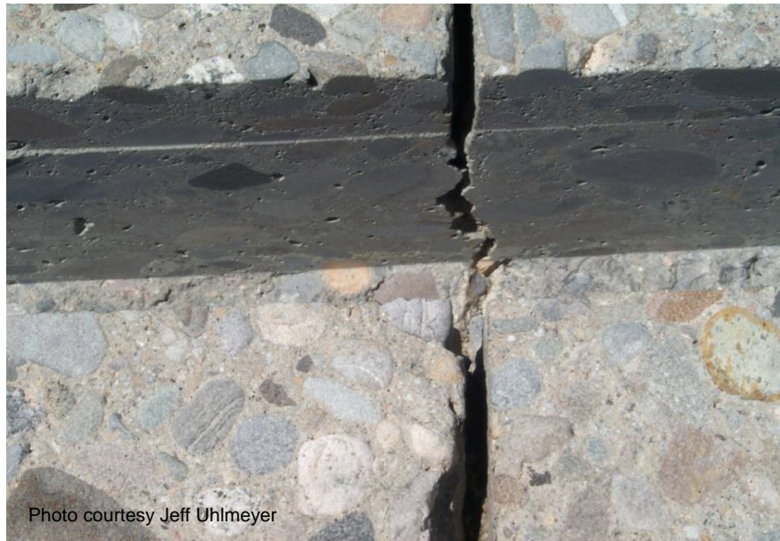
Figure A-42. Cleaned dowel bar slot.
