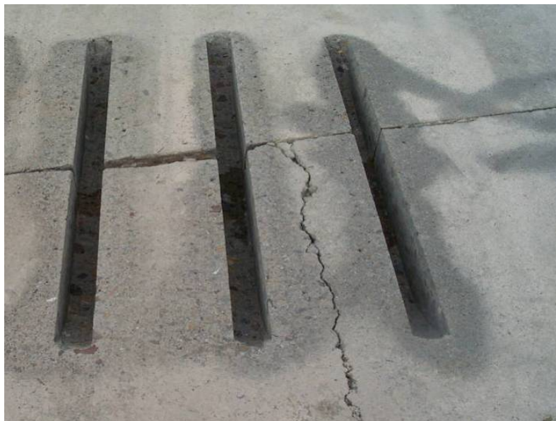
Figure A-18. Dowel bar slots aligned to miss an existing longitudinal crack.
