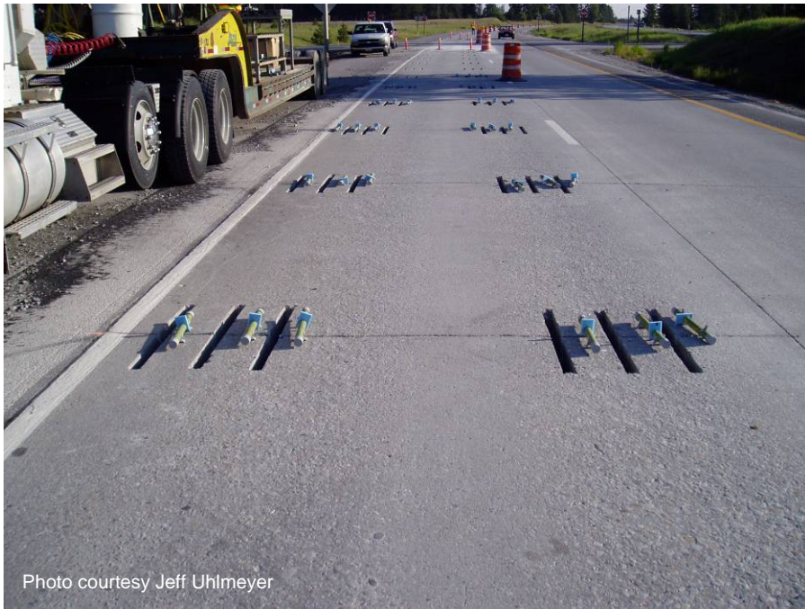
Figure A-53. Dowel bar retrofit assemblies.
