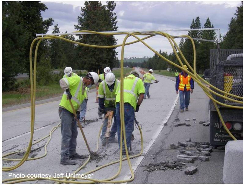
Figure A-24. Jackhammer operation.
