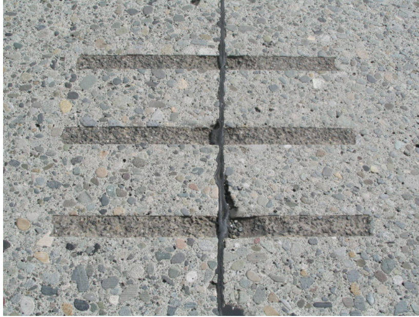
Figure A-46. Spalling of patching material.
