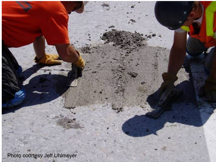
Figure A-71. Finishing patching material.
