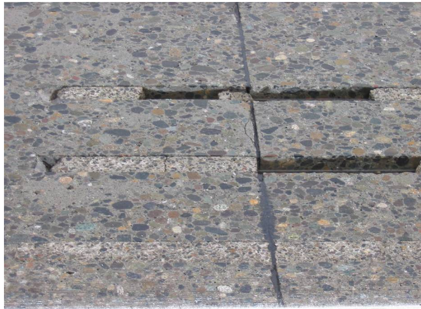
Figure A-45. Patching material bond failure.
