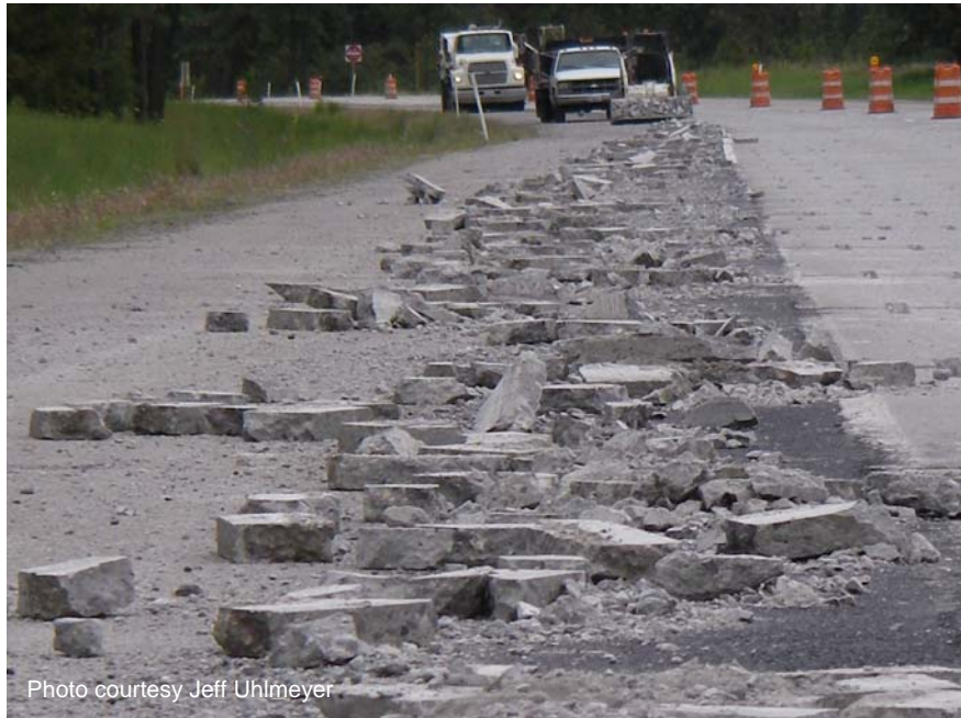
Figure A-32. Debris from the jackhammering process.
