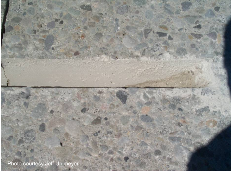
Figure A-36. Sawcut blade residue on slot walls.
