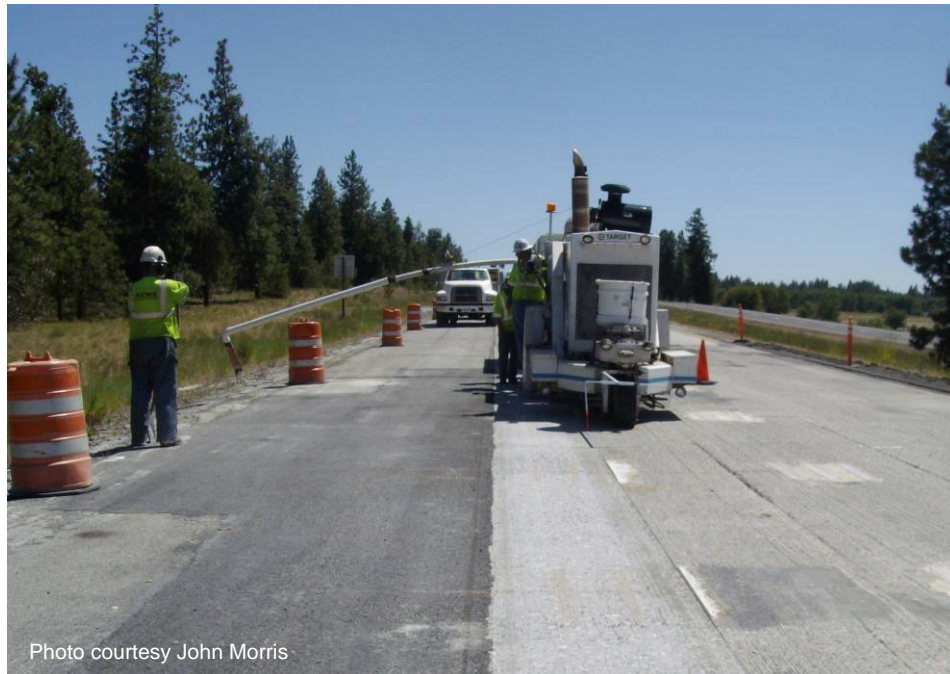
Figure A-82. Diamond grinding equipment.
