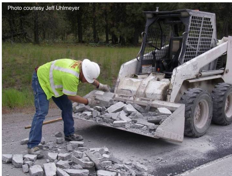
Figure A-34. Debris removal.
