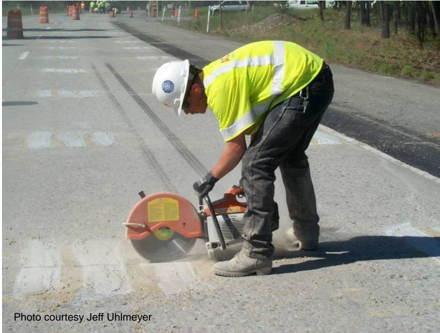
Figure A-76. Establishing joint in patching material.
