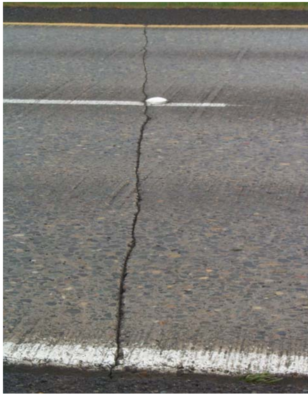
Figure A-77. Transverse tape joint (original construction).
