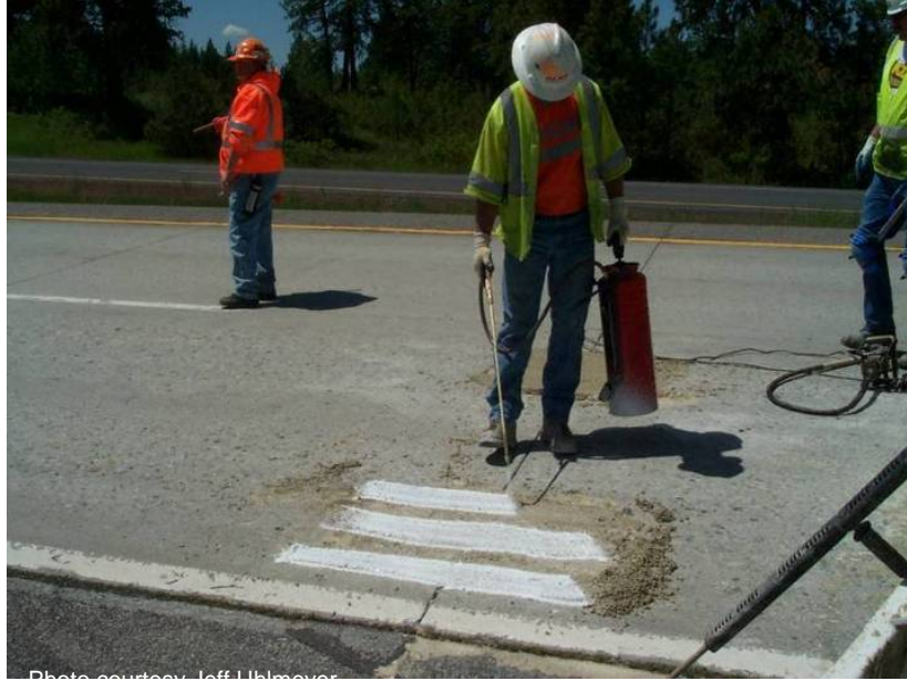
Figure A-75. Applying curing compound.
