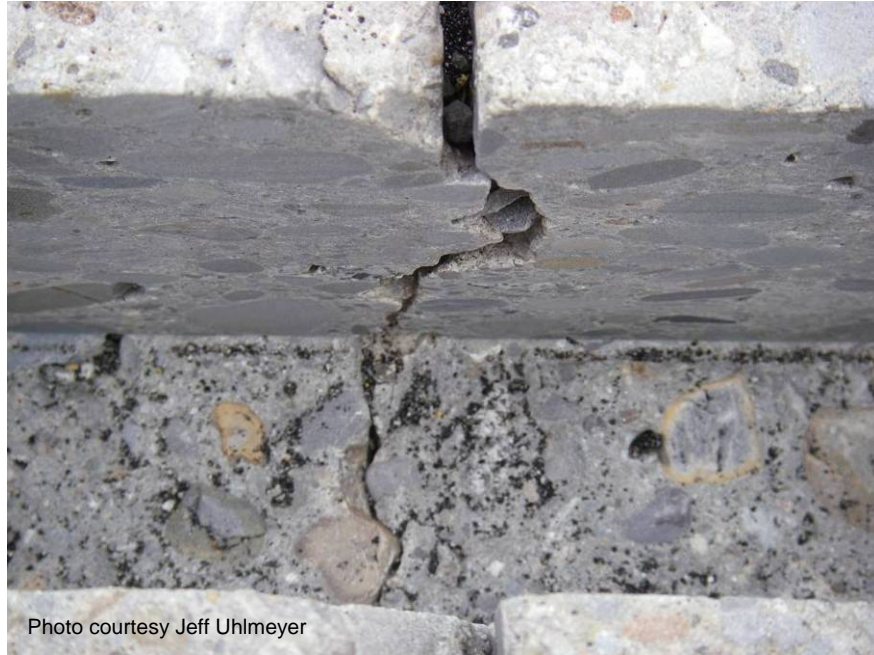
Figure A-38. Dowel bar slot after shot blasting.
