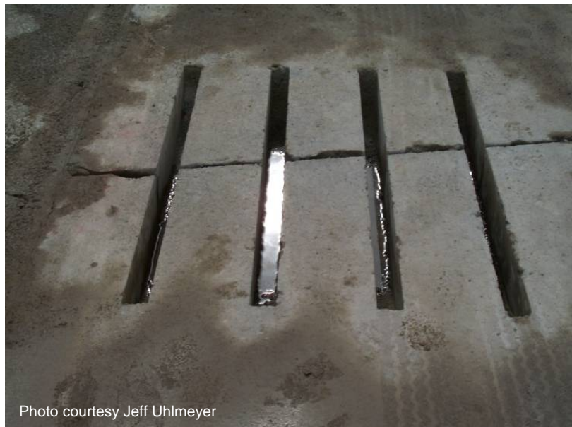
Figure A-43. Water must be removed prior to placement of patching material.
