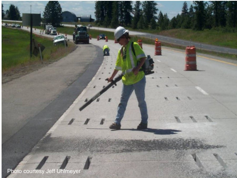
Figure A-39. Cleaning shot blasting debris from roadway.
