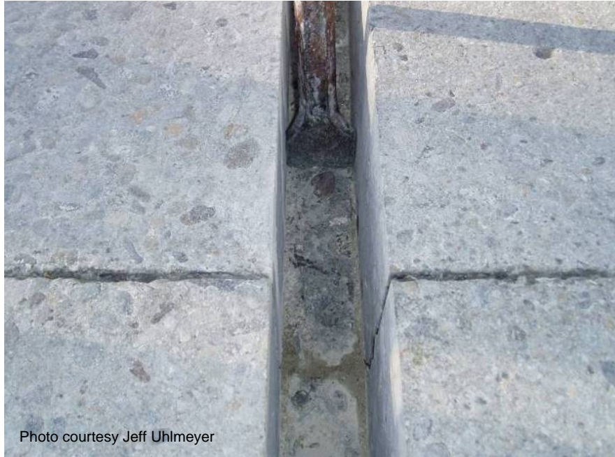
Figure A-26. Leveling dowel bar slot bottom.
