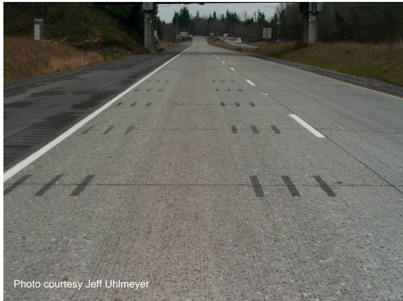
Figure A-84. Completed roadway.
