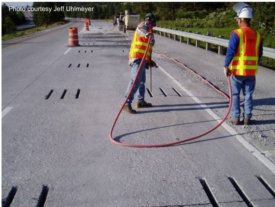
Figure A-41. Cleaning dowel bar slots with compressed air.
