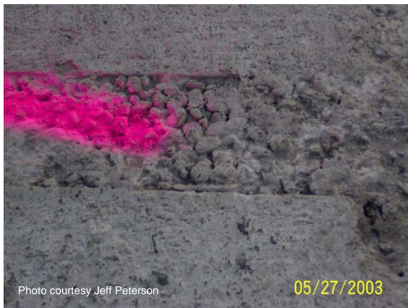
Figure A-47. Insufficient consolidation of patching material.
