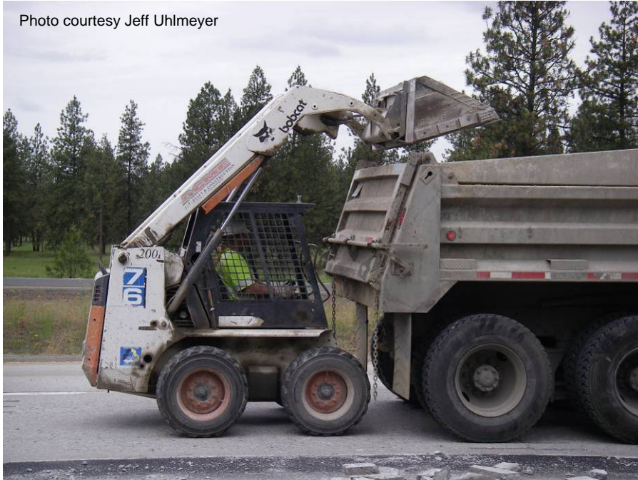
Figure A-35. Debris removal.
