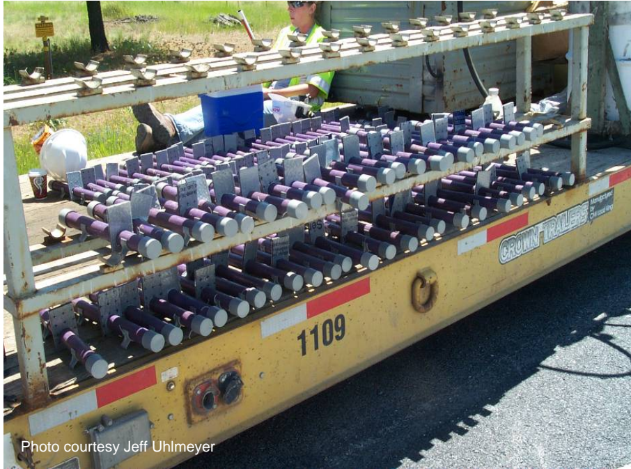
Figure A-52. Dowel bar retrofit assemblies.
