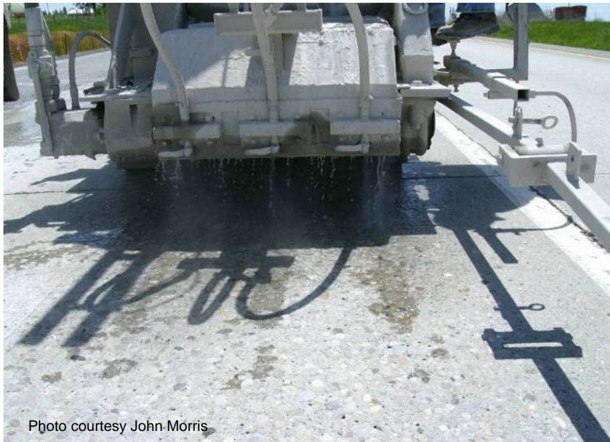
Figure A-10. Cutting equipment for three dowel bar slots per wheelpath.
