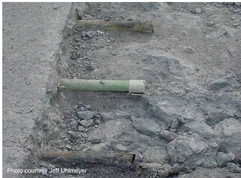
Figure A-59. Corroded epoxy coated dowel bars.
