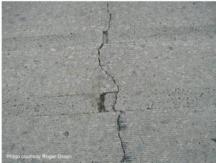
Figure A-67. Misaligned foam core board.
