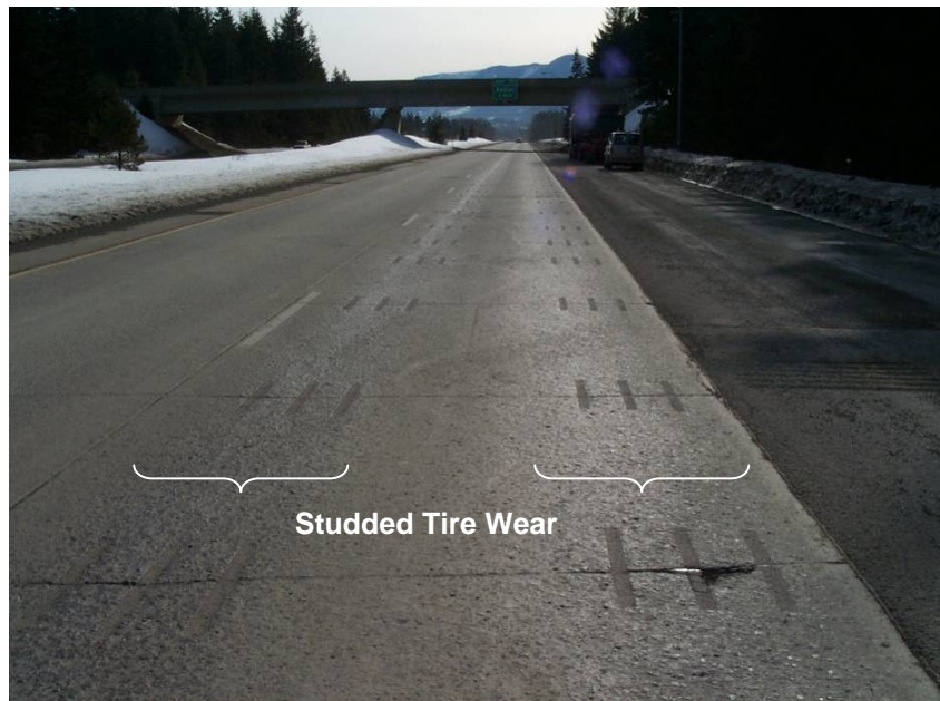
Figure A-79. Wear due to studded tires.
