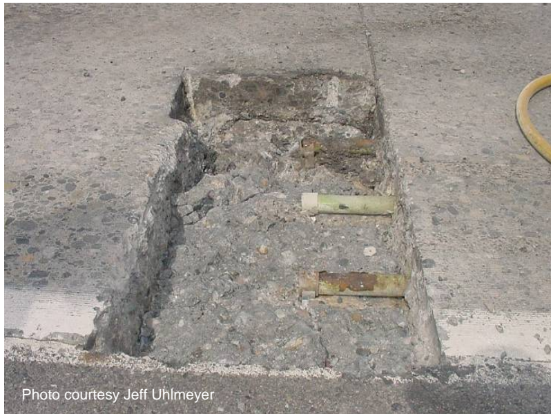
Figure A-60. Corroded epoxy coated dowel bars.
