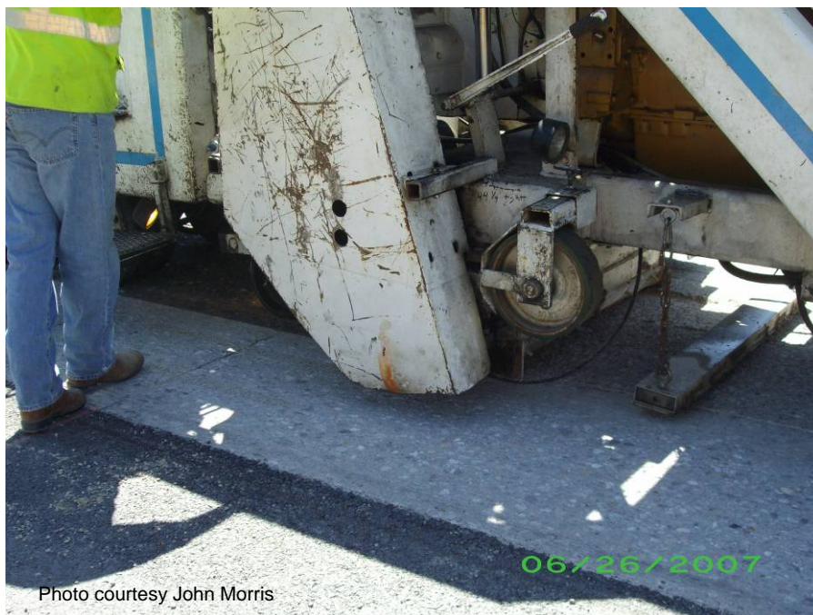
Figure A-83. Diamond grinding equipment.
