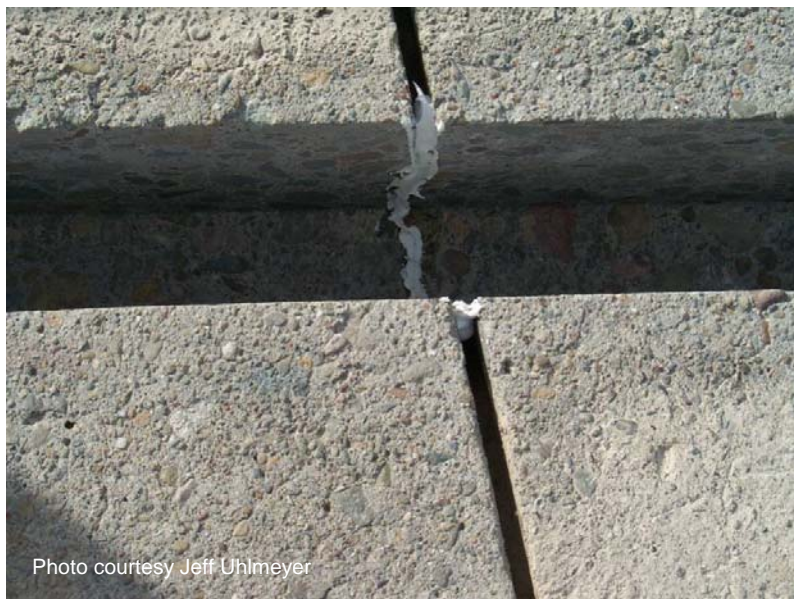
Figure A-51. Caulked dowel bar slot.
