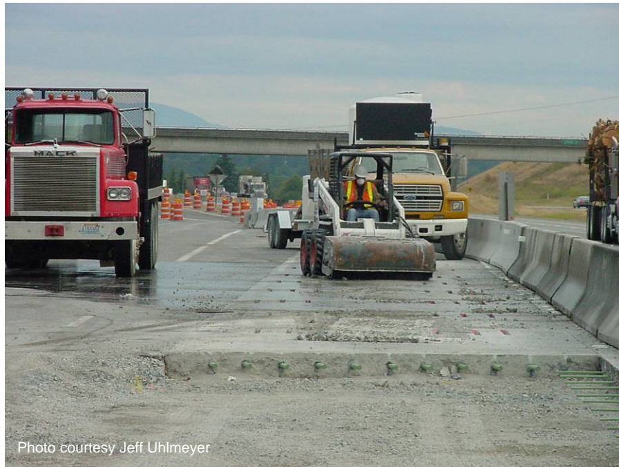
Figure A-33. Debris removal.
