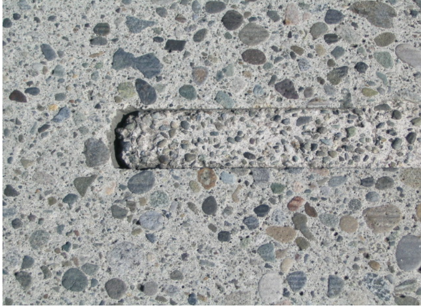
Figure A-44. Patching material bond failure.
