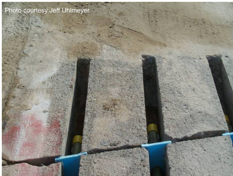
Figure A-49. Debris should be cleared to a sufficient distance to prevent intrusion.
