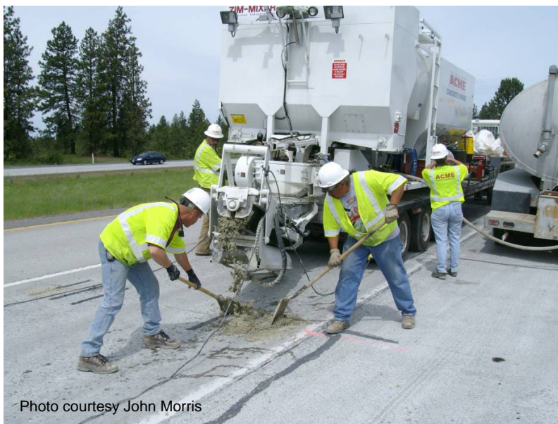
Figure A-63. Placing patching material.
