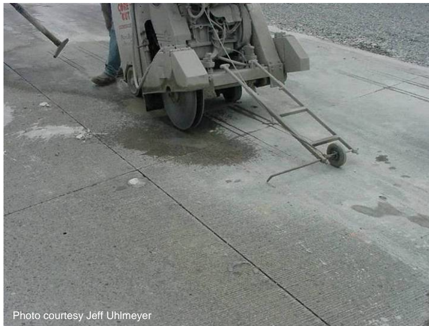
Figure A-12. Cutting equipment for one dowel bar slot at a time.
