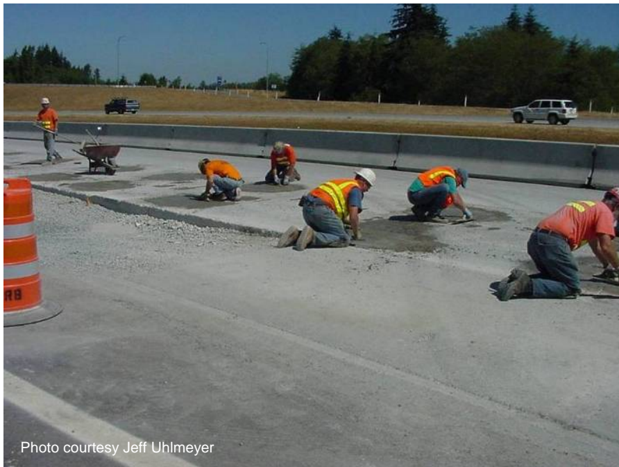
Figure A-72. Finishing patching material.
