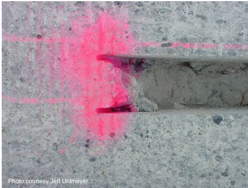
Figure A-30. Concrete not sufficiently removed from the end of the dowel bar slot.
