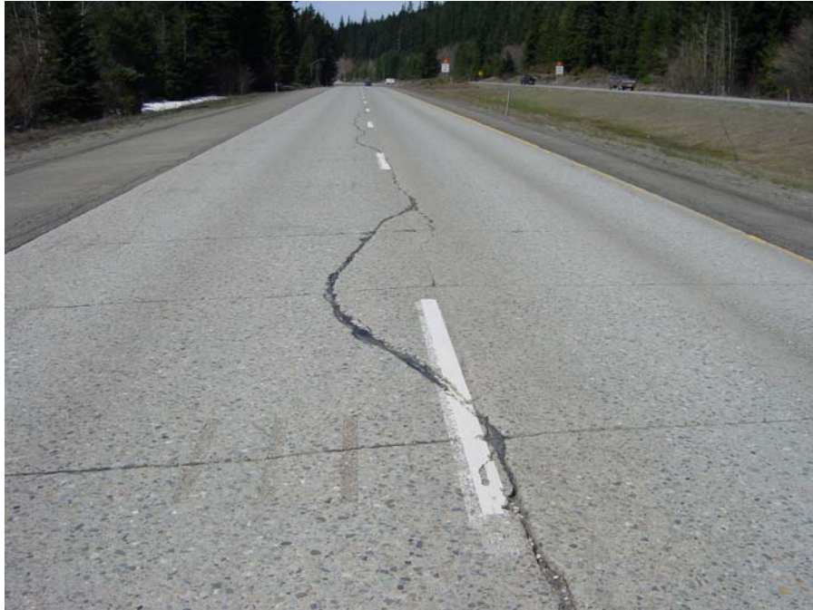
Figure A-19. Left wheelpath dowel bar slots not installed to avoid existing longitudinal crack.
