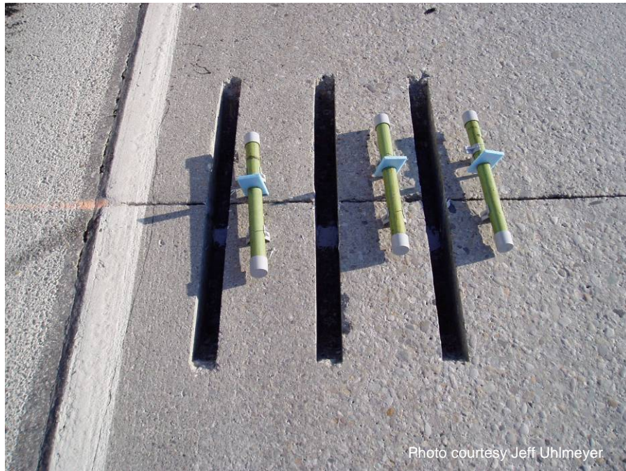
Figure A-54. Dowel bar retrofit assemblies.
