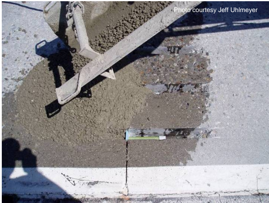
Figure A-64. Placing patching material.
