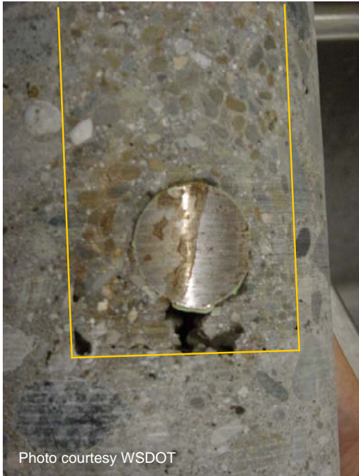
Figure A-69. Poor consolidation.
