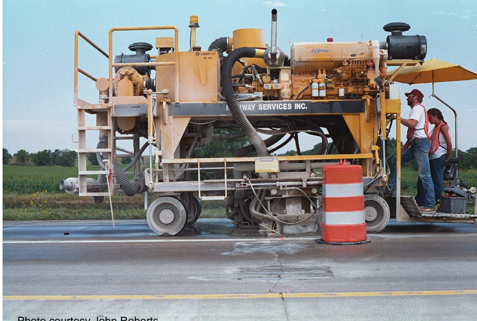
Figure A-9. Cutting equipment for six dowel bar slots per joint.
