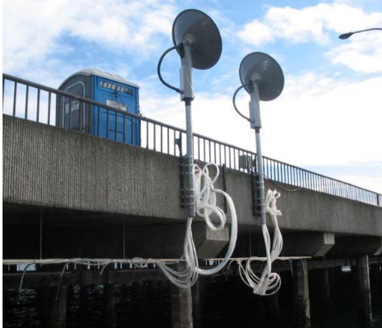
Figure A-1: Image of the fiber optic lighting system. The two dishes above the dock optimize light reception by tracking the sun position, and the cables transmit light underneath the dock.
