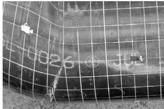
b) Tearing of Steel in Shear Zone
