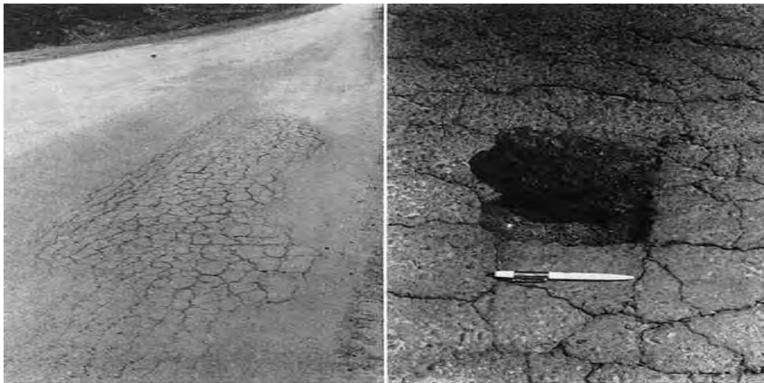
Figure 1.1. Typical Pavement Failure Primarily Caused by Degradation of Underlying Base Material (Minor, 1959).
