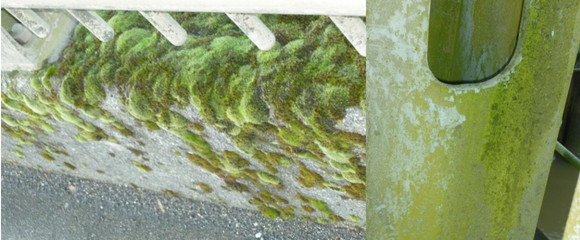
Figure 6. Hoquiam River Riverside 1417 Bridge
