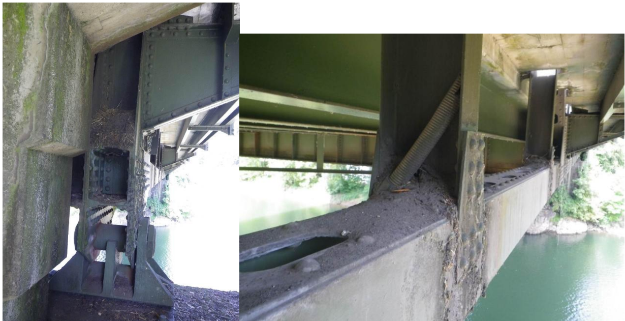
Figure 1. Bottom chord ends
