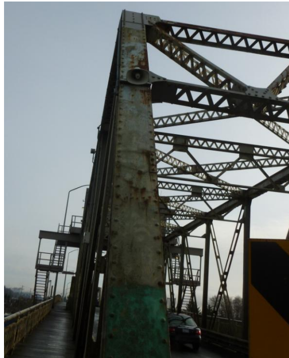
Figure 7. Southeast-bound US 101 Bridge
