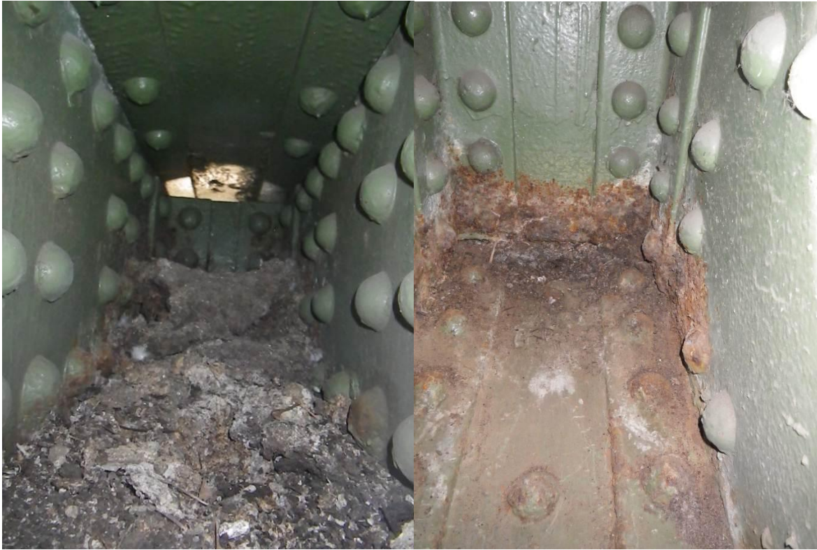
Figure 2. Bottom chord interiors
