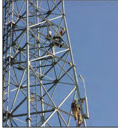
Figure 7: WSDOT radio crews installing dishes and antennas (credit: WSDOT)
