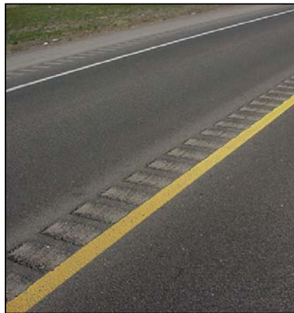
Figure 1: Milled centerline rumble strip (CLRS).
