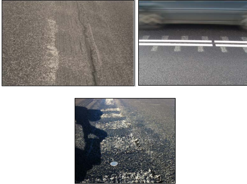
Figure 4: From left to right: European “sinus,” rectangular (Kragh, 2007), and WSDOT cylinder design.
