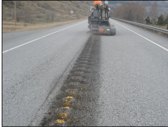
Figure 2: Grinding CLRS on SR 97
