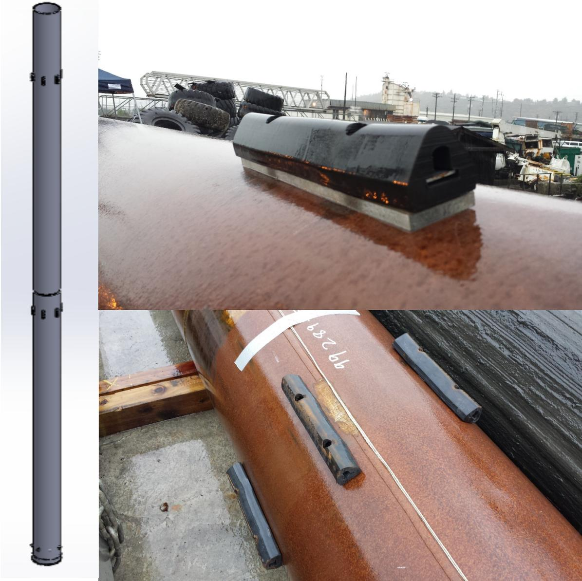
**Figure 16:** Installation of pile spacers
