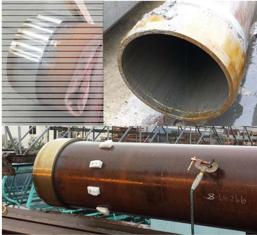
**Figure 17:** Mandrel before and after pile installation
