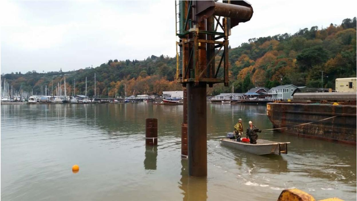
**Figure 3a.** Photograph made on October 30<sup>th</sup> of the 3 piles shown in order of nearest to farthest: Mandrel Pile, Double Pile and Control Pile. Buoy marker on left shows approximate position of the VLA.
