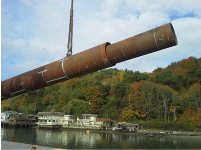
**Figure 26:** Lofting of the double pile
